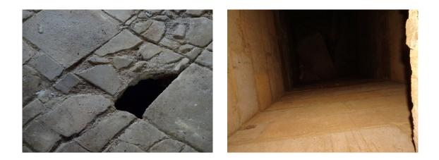
Figure 11 Partially collapsed flagstone (left) in the storeroom together with a view of through the opening to reveal the underlying void space (right). It would appear that the flagstone floor is suspended between structural walls with no additional packing material to stabilise the void.
