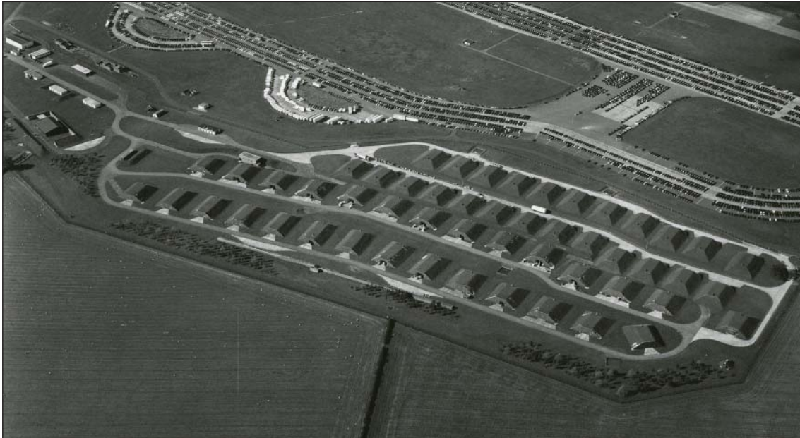
Figure 12: RAF Upper Heyford, southern conventional bomb stores showing the Igloo stores constructed during the 1970s and 1980s. (c) Historic England 18537/04
