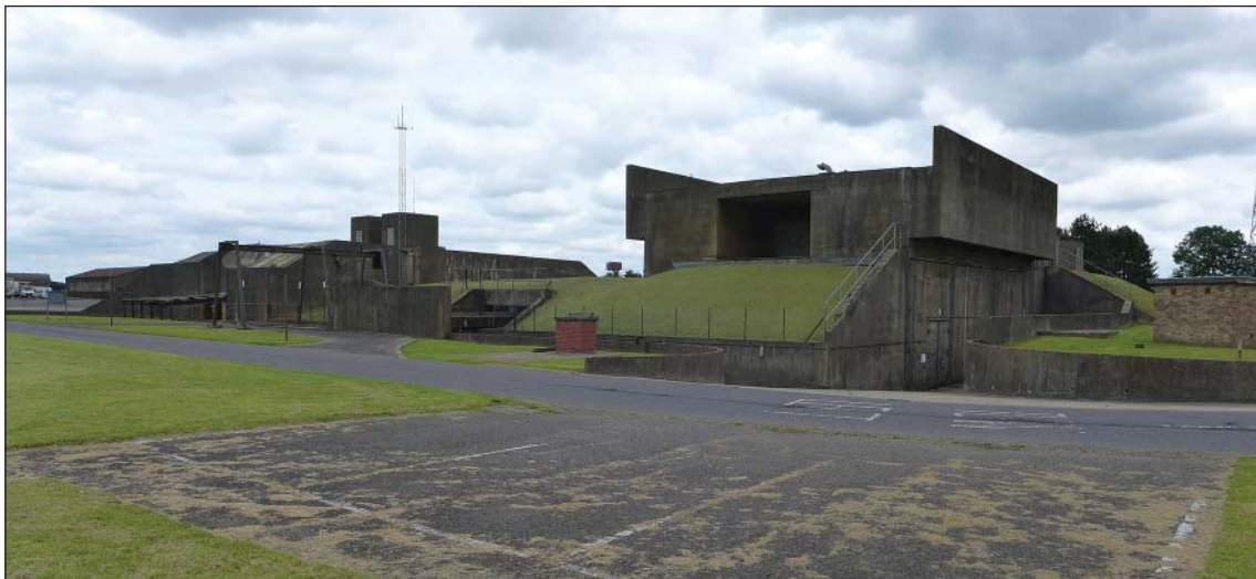
Figure 17: RAF Upper Heyford, 299 Avionics Building. (c) W D Cocroft
