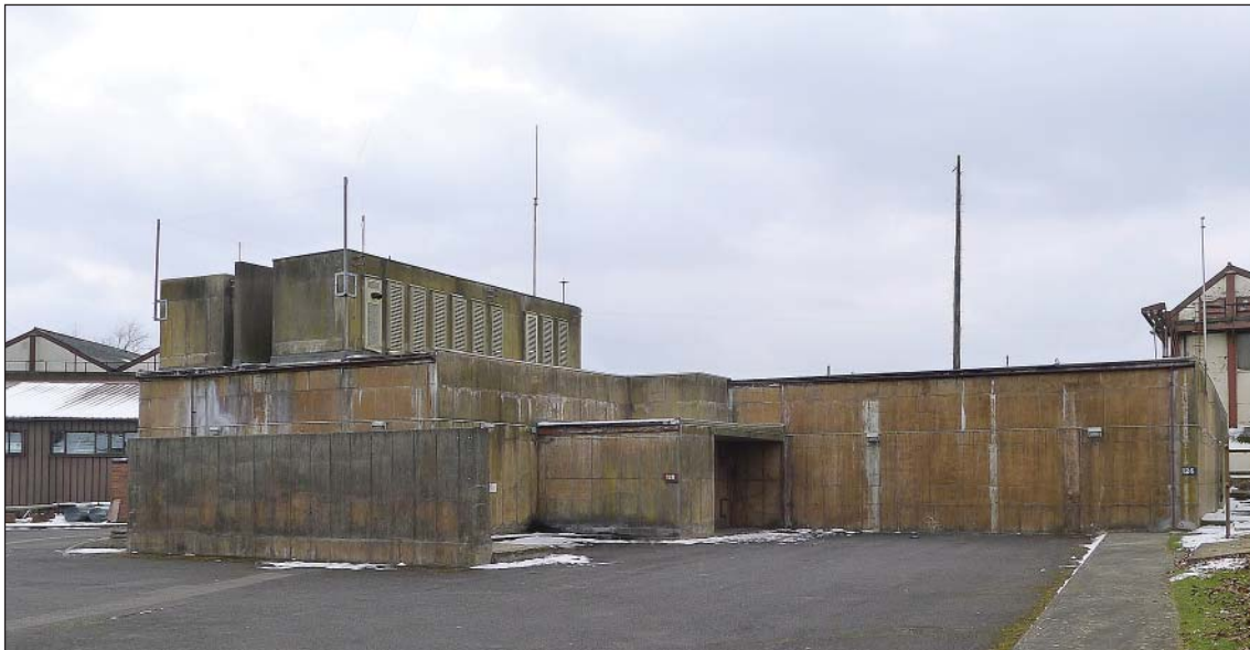
Figure 18: RAF Upper Heyford, 126 hardened Wing Headquarters built to a standard NATO design. (c) W D Cocroft
