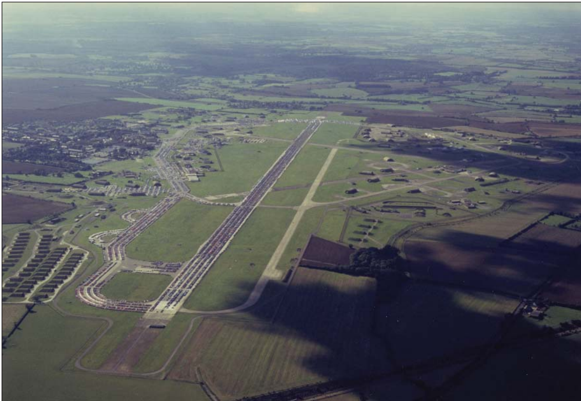
Figure 5: RAF Upper Heyford, February 1999 this view shows the airfield soon after closure with the new NATO emergency runway to the right (c) Historic England 18517/25
