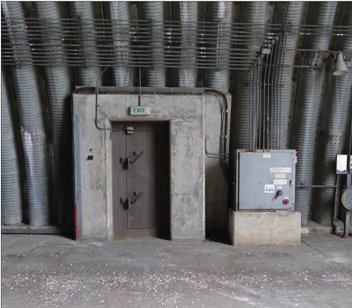
Figure 16: RAF Upper Heyford, typical Hardened Aircraft Shelter, interior showing metal formers and pedestrian access door. (c) W D Cocroft
