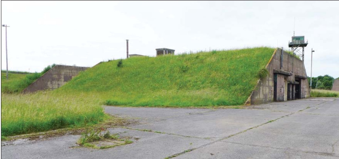
Figure 22: RAF Upper Heyford, 1006 Northern Bomb Stores , early 1950s Plant building for maintaining nuclear weapons. (c) W D Cocroft
