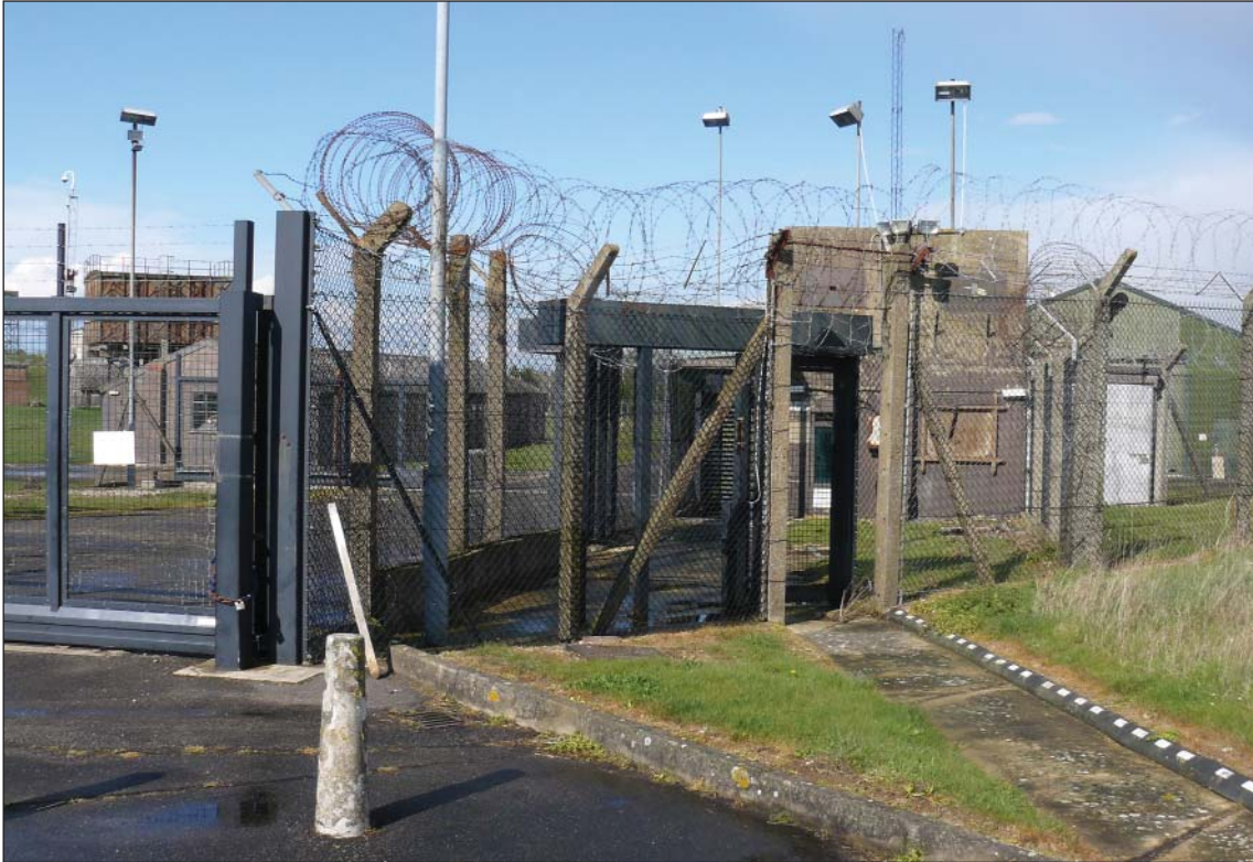
Figure 10: RAF Upper Heyford, 1980s heavily protected entrance to the Northern Bomb Stores. (c) W D Cocroft
