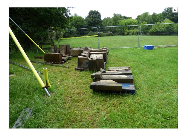
6 As dismantling continued, the masonry elements were carefully stored so that they could be incorporated accurately as the monument was rebuilt.
