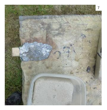
7 Replacement stainless-steel cramps were fixed in lead. This image shows a trial after the lead was introduced. Hot, molten lead was poured into the cavity in the stone. Once cooled, the lead solidifies tightly around the cramp (not seen).
