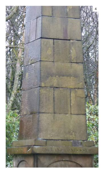
4 The effect of corroded cramps was evident in the jacking of course joints throughout the monument. Individual masonry pieces were generally in a sound condition, with minor surface delamination.
