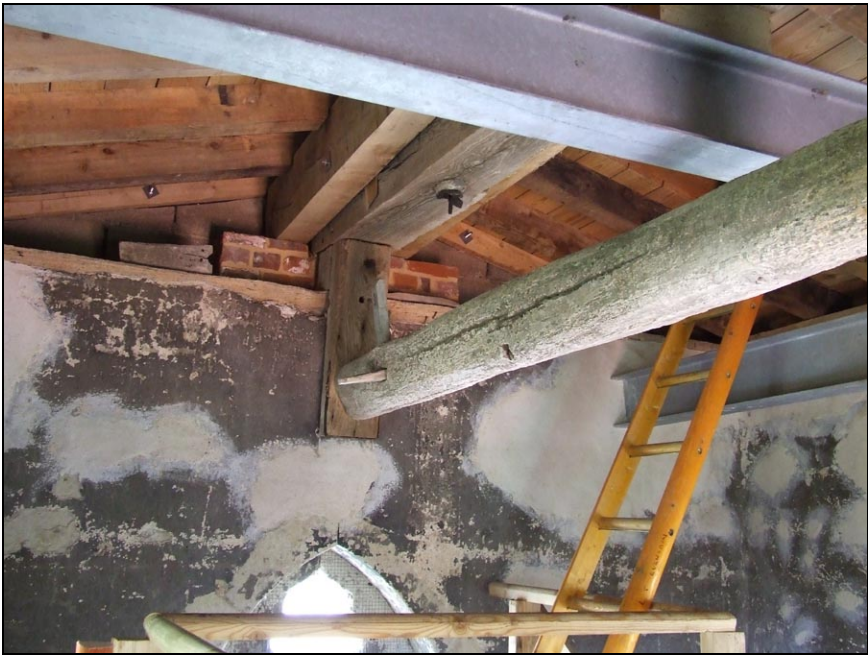
Figure 2: Photograph of the windlass in position under the repaired roof
