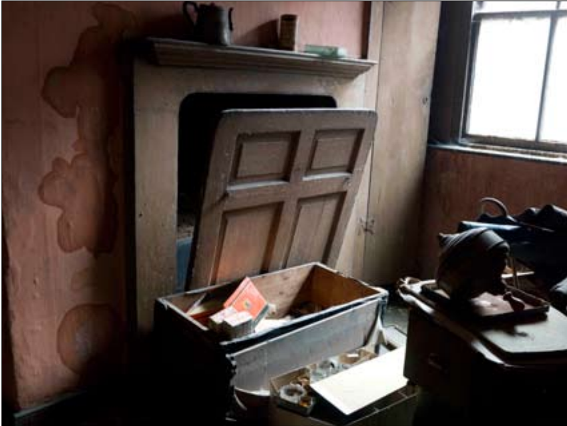
Fig. 72: The bedroom over the kitchen on the second floor of the outshot, 57 West Street / 64-66 Bridge Street. The fireplace can be closed off with a chimney board. DP065395 © English Heritage
