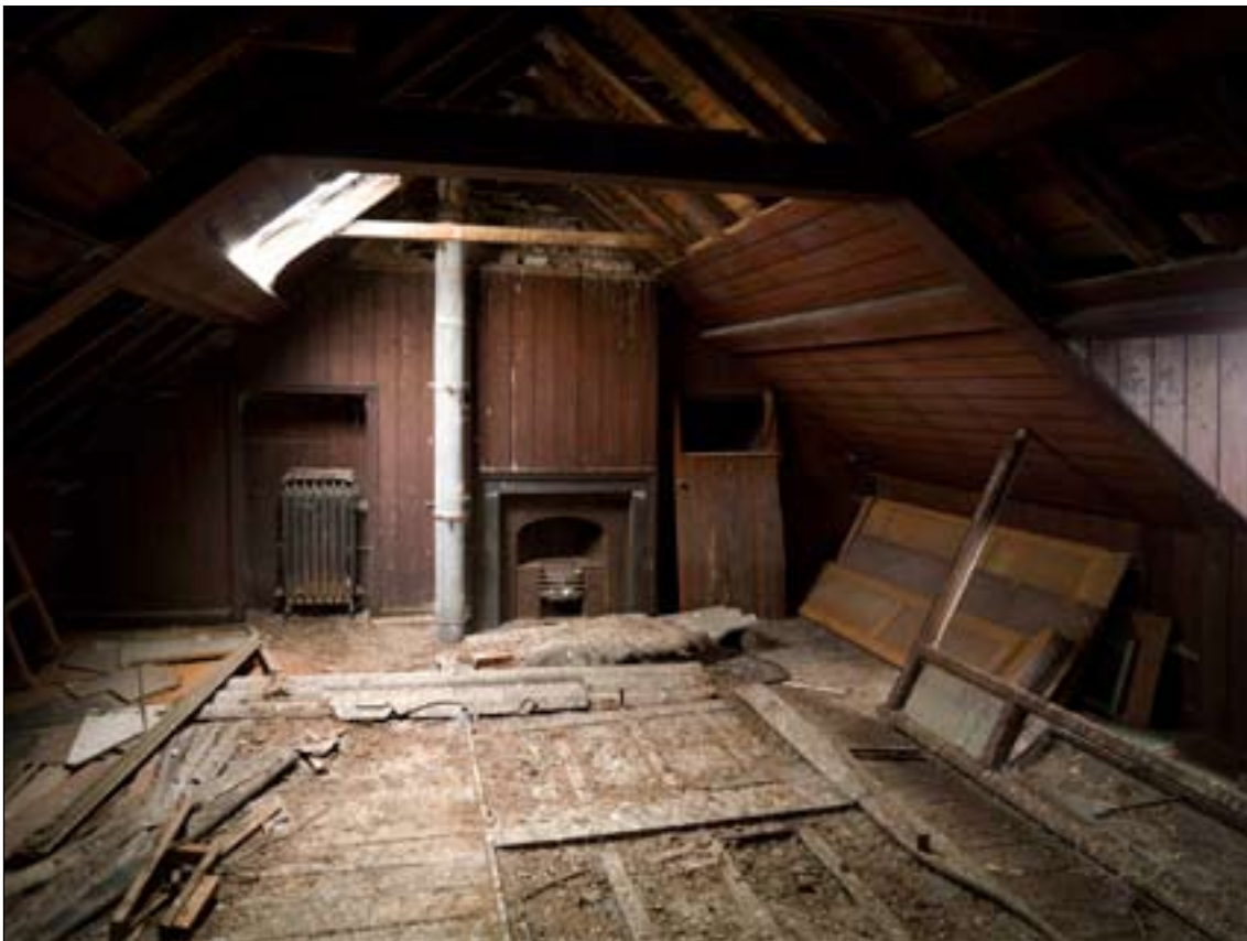
Fig. 51 (below): The tongued-and-grooved boarded office in the attic of the granary. DP065355 © English Heritage
