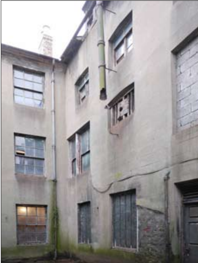
Fig. 50 (left): Altered fenestration in the south wall of the granary, including a paired sash window on the first floor. © English Heritage
