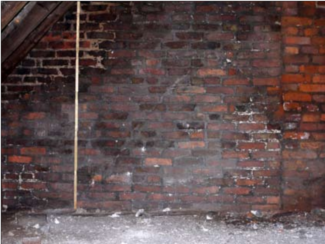
Fig. 57: The mortar traces of an earlier, probably thatched roofline visible on the eastern gable wall of the attic, 57 West Street / 64-66 Bridge Street. © English Heritage
