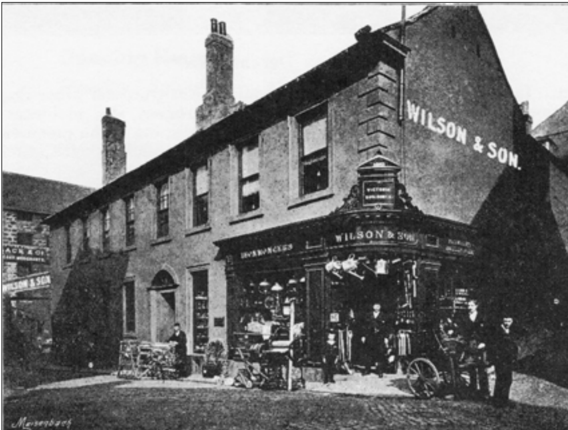
Fig. 14: The corner of 2 Love Lane / 64 West Street transformed into Victoria Buildings. Late 19th-century photograph reproduced from Pike 1894, 26, reprinted 1995. © Berwick-upon-Tweed Record Office
