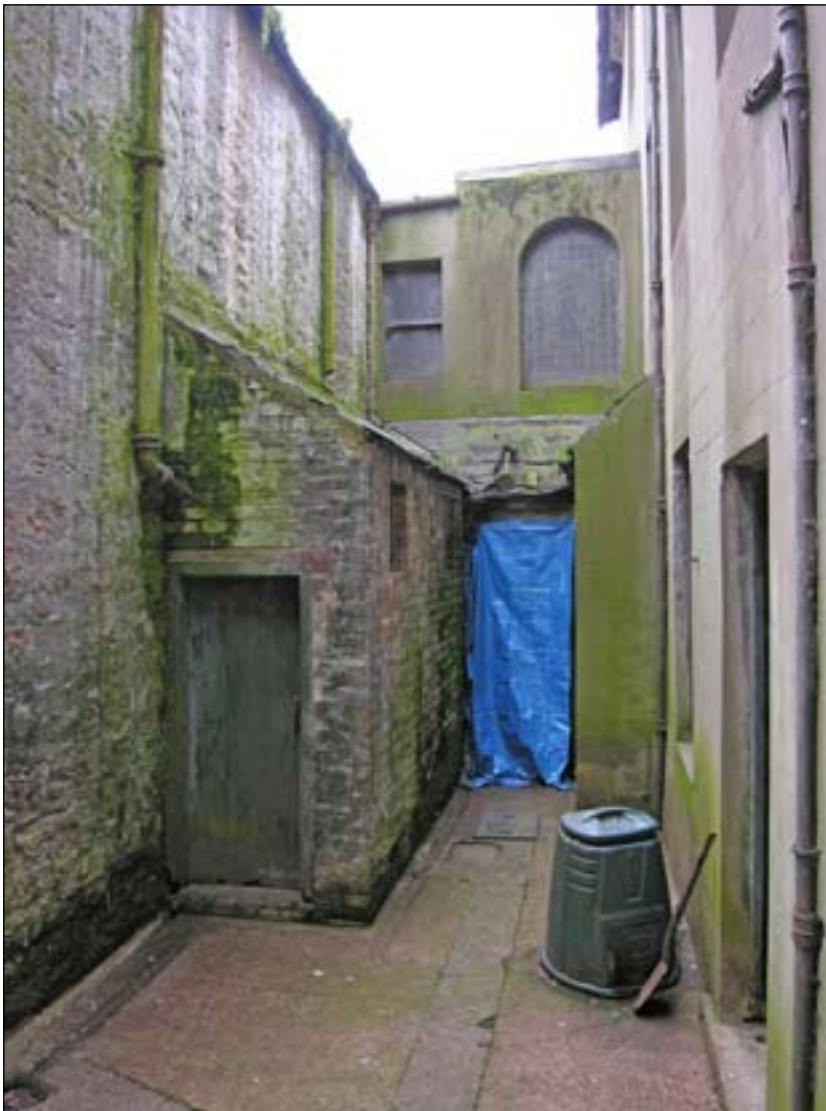
Fig. 16: The northern elevation of the stair turret of 2 Love Lane / 64 West Street, seen from the 'inside yard'. © English Heritage
