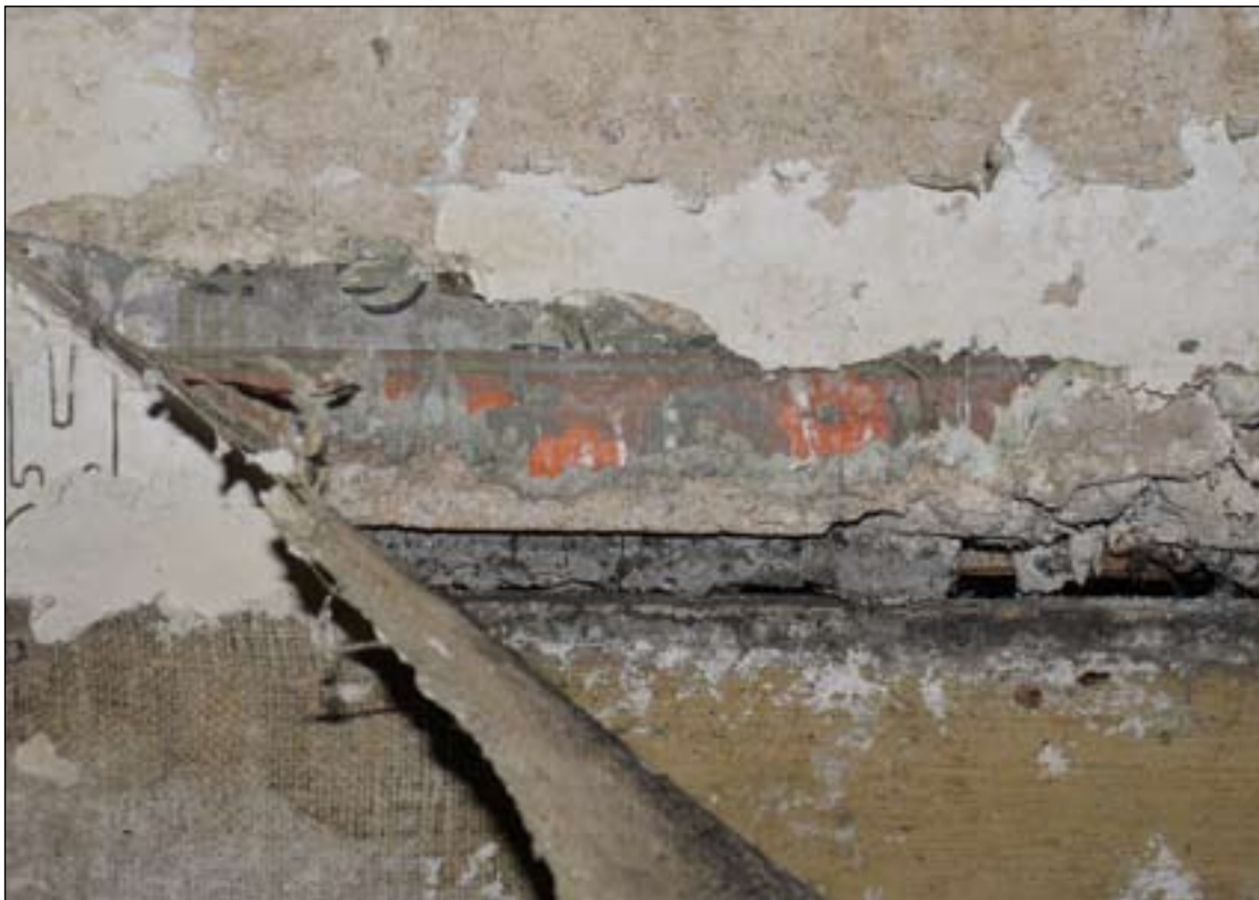
Fig. 69: The wallpaper border at dado-rail height in the west room on the second floor of the principal range, 57 West Street / 64-66 Bridge Street. © English Heritage
