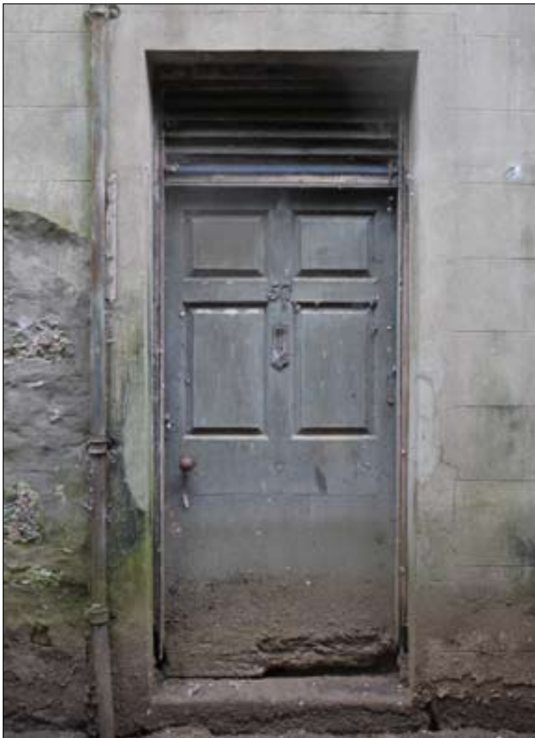
Fig. 61: The former door of 57 West Street, complete with number, reused on the ground floor of the granary at 60 West Street. © English Heritage
