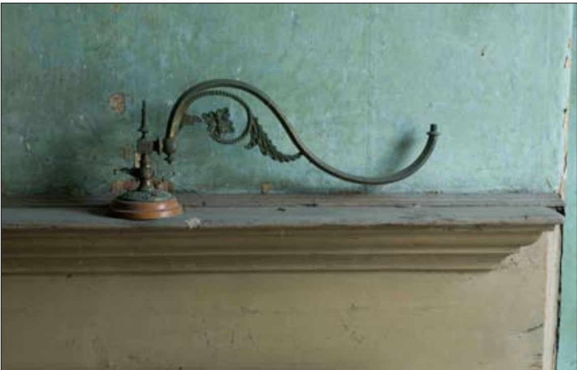
Fig. 83: An adjustable bracket which once supported a gas lamp, found in the bedroom on the second floor of the western end of the outshot, 64-66 Bridge Street / 57 West Street. DP065392 © English Heritage
