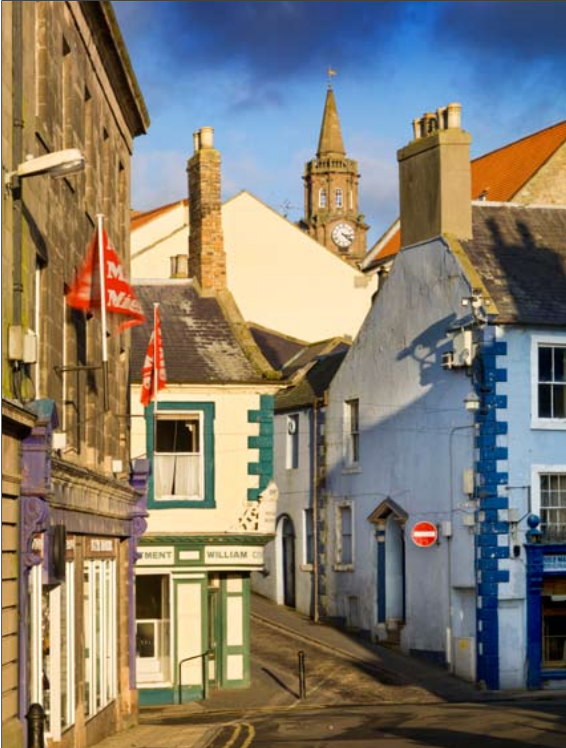
Fig. 2: View north-eastwards from the Berwick end of the bridge, showing West Street with the corners of 2 Love Lane / 64 West Street (painted green and cream) and 57 West Street / 64-66 Bridge Street (painted blue). DPI36050 © English Heritage
