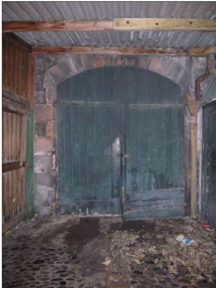
Fig. 44: The carriage house arch in the western end of the southern wall of the granary. © English Heritage
