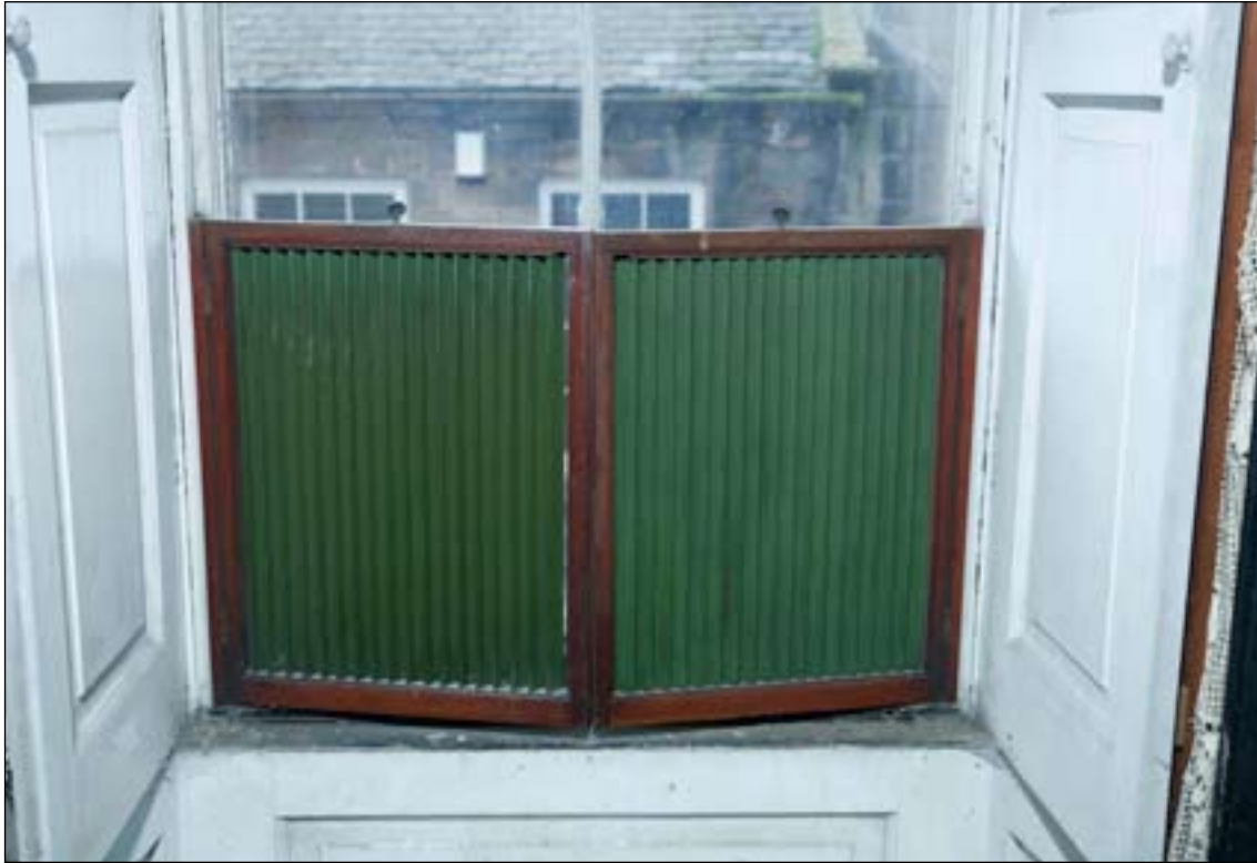
Fig. 79: Dwarf blinds (shut) in one of the windows of the largest second-floor room at 64-66 Bridge Street / 57 West Street. DP065385 © English Heritage
