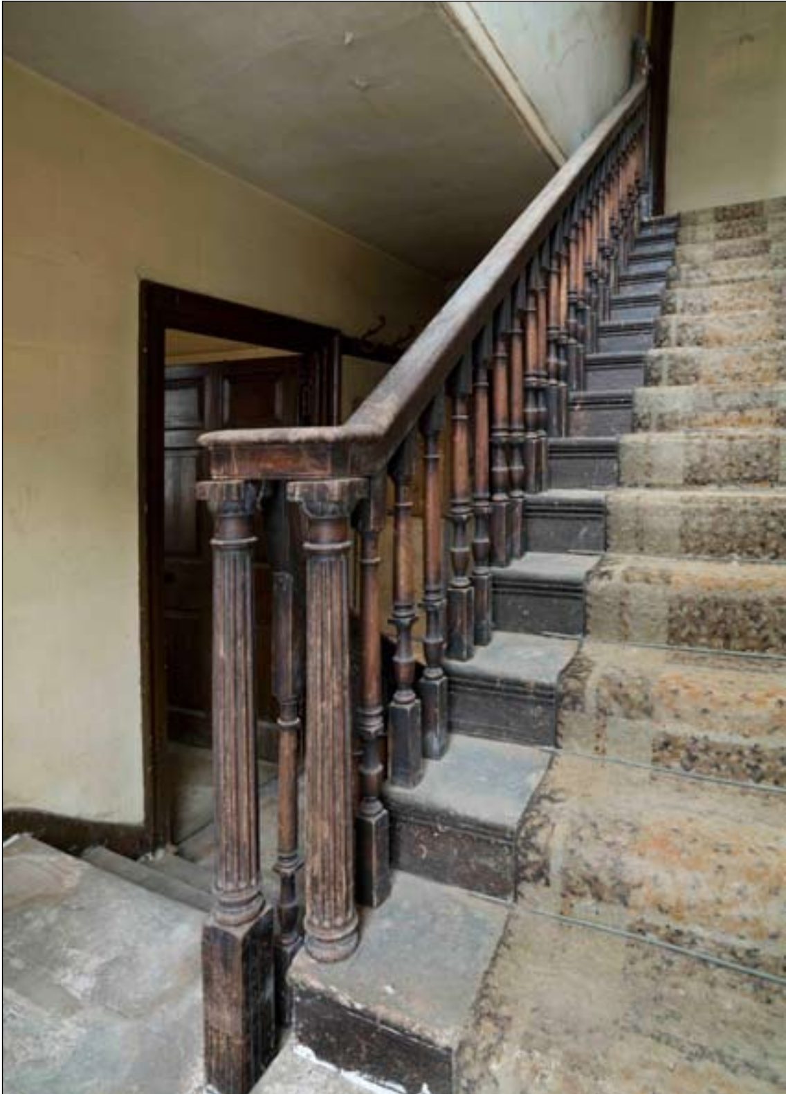
Fig. 67: The main stair, with its column newels and two balusters per tread, in the principal range of 57 West Street / 64-66 Bridge Street. The lower flight has been shortened by one step, and the corresponding newel lengthened, to maintain headroom when the second-floor west room was extended into the stair compartment. DP065374 © English Heritage
