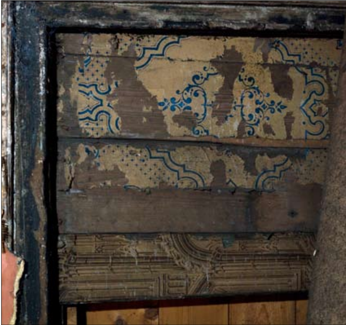
Fig. 73: The blocked doorway with its wallpapered planks, on the second floor of the outshot, 57 West Street / 64-66 Bridge Street. The pillar-and-arch paper, applied sideways, is characteristic of the third quarter of the 18th century; the blue design is mid-19th-century. DP065397 © English Heritage
