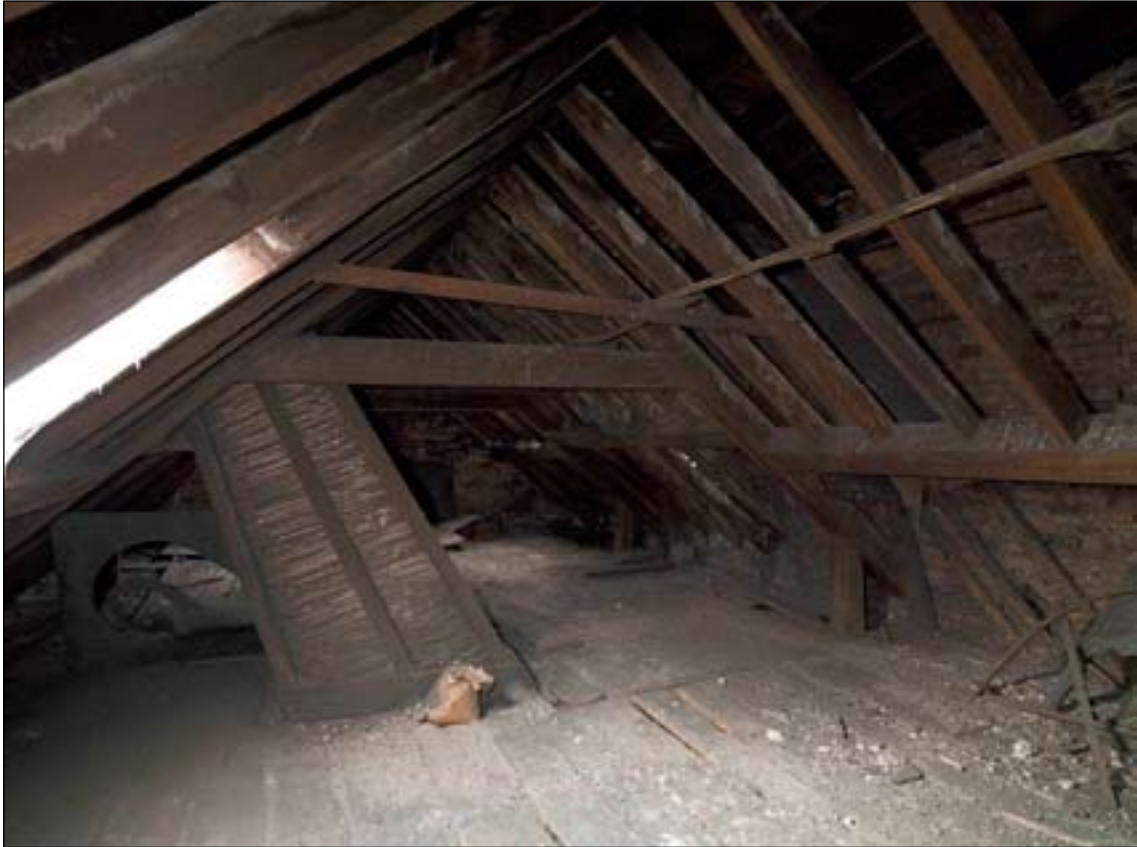
Fig. 27: The roof of the front range of 2 Love Lane / 64 West Street. The boxed-in skylight illuminates the stair serving the western first-floor room. DP065340 © English Heritage
