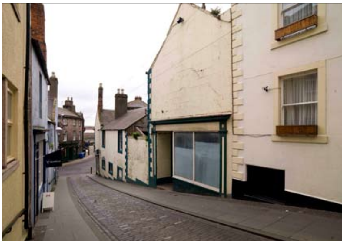
Fig. 39: View of the east end of the granary facing onto West Street, denoted by the large gable and shop front as well as the 2-storey strip of green quoins to its left-hand side. DP065338 © English Heritage
