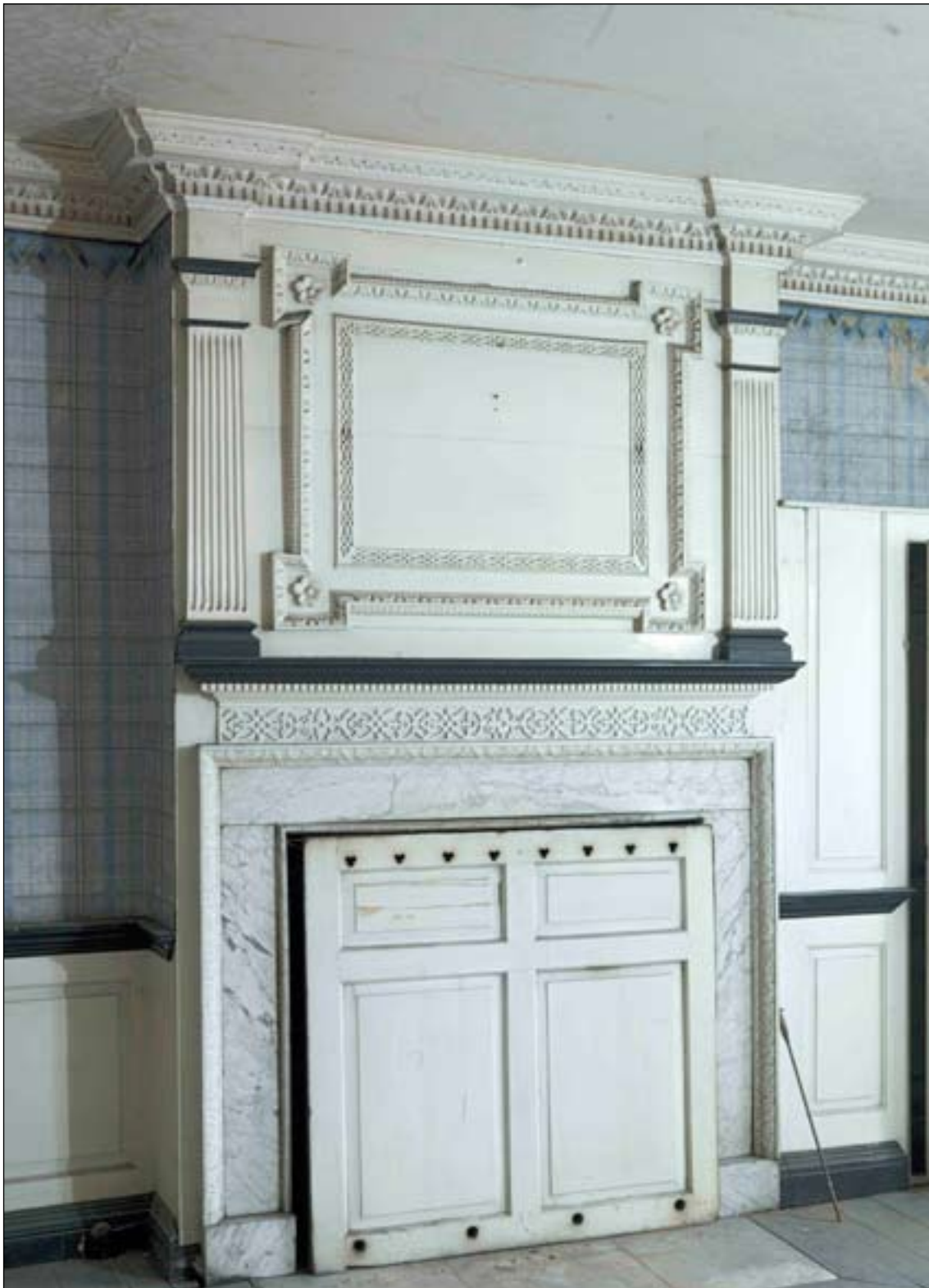
Fig. 70: The chimney piece and over mantel, complete with chimney board, in the large east room on the second floor of the principal range, 57 West Street / 64-66 Bridge Street. DP065380 © English Heritage
