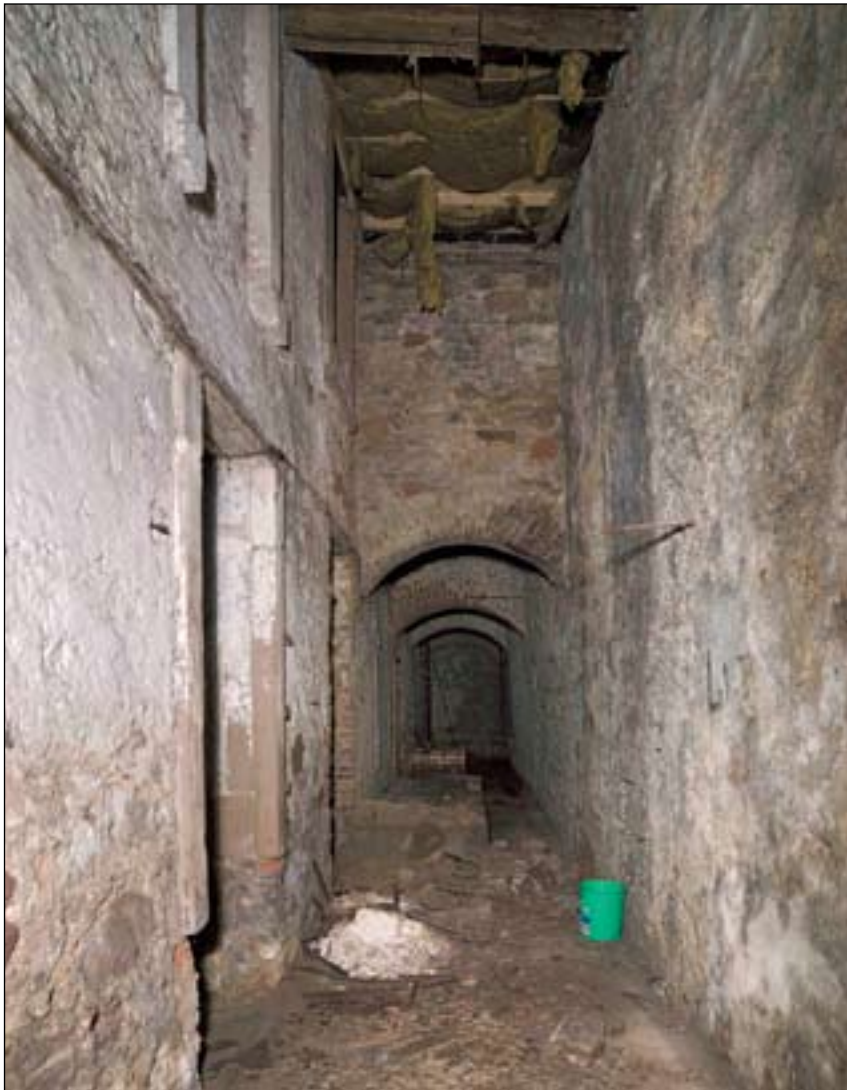
Fig. 45: The passageway on the line of the Cat Well Wall, showing the north wall of the granary to the left. DP065315 © English Heritage
