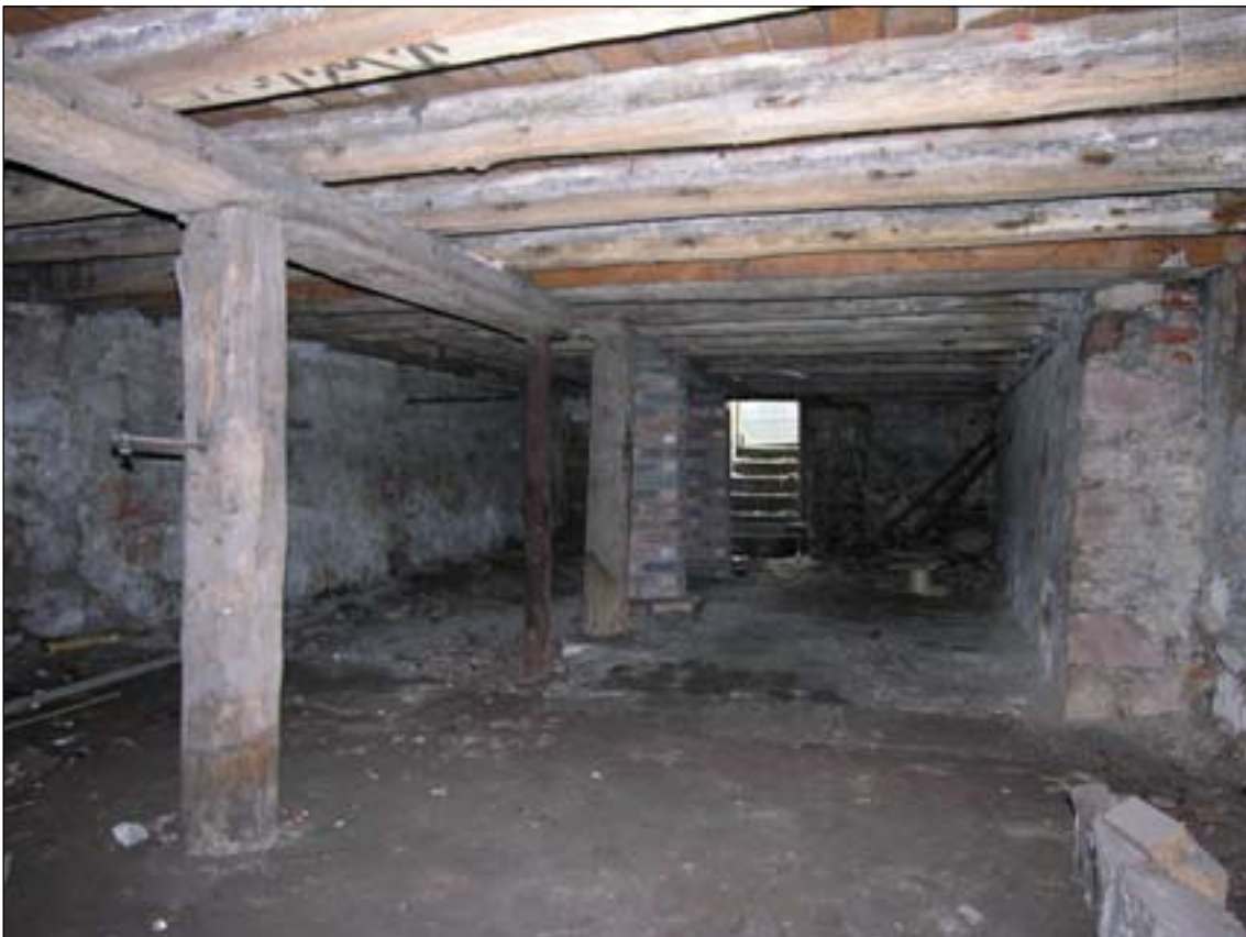
Fig. 38: The cellar of 2 Love Lane / 64 West Street, looking west. The ceiling bears a series of painted inscriptions, including J Wilson's name on a joist and the date 1887 (not visible) on plaster. The supporting axial beam and Samson posts are more characteristic of 18th- and early 19th- century warehouses and granaries. © English Heritage
