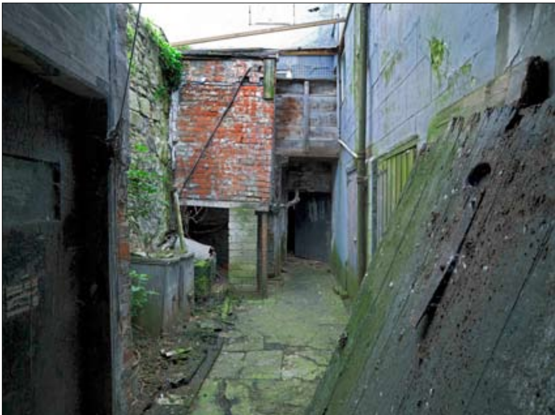
Fig. 56: The cramped yard at the rear of 57 West Street / 64-66 Bridge Street. The rendered rear range is to the right and the brick coal bin of 51 West Street is in the centre. DP065401 © English Heritage
