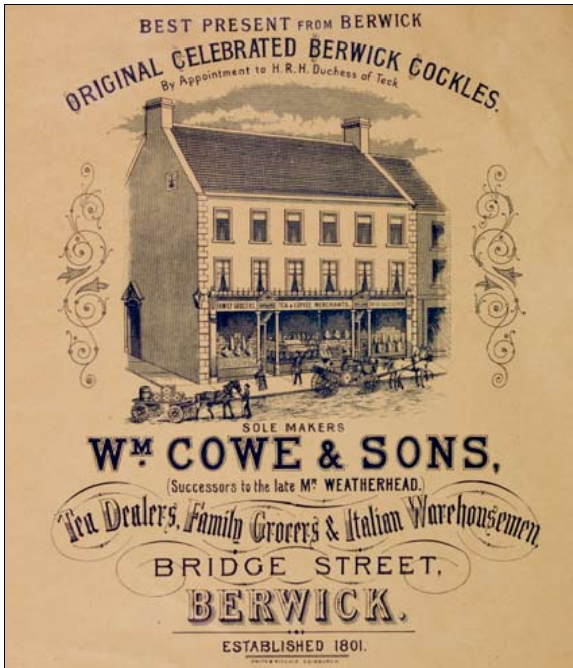
Fig. 78: Blinds can be seen in the second-floor windows of 64-66 Bridge Street / 57 West Street, as illustrated in this William Cowe & Sons publicity material, found in the shop. DP065140 © English Heritage
