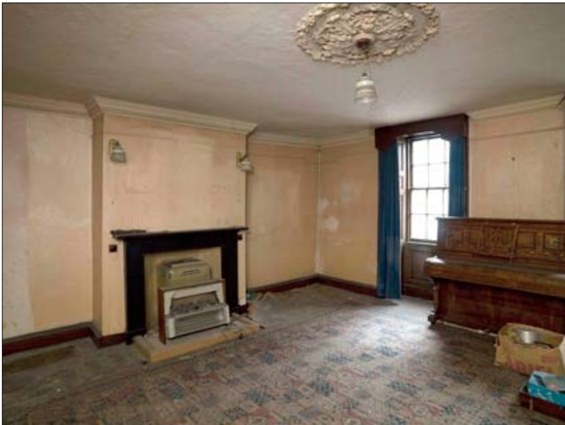
Fig. 65: The large first-floor room in the principal range of 57 West Street / 64-66 Bridge Street. DP065365 © English Heritage
