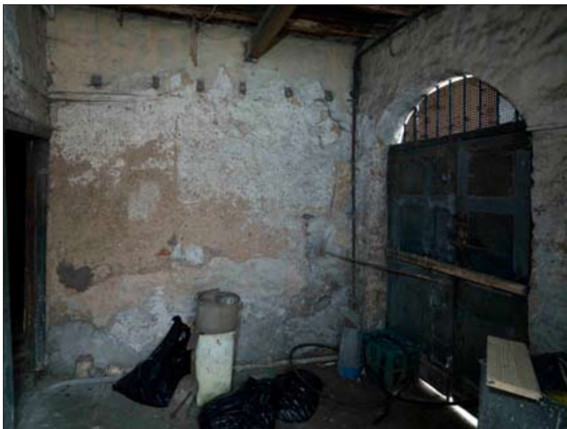
Fig. 76: The yard entrance at the side of 57 West Street / 64-66 Bridge Street, looking south-west. The rafter ends of a former pent roof are visible a little below the ceiling of the added rear range. DP065402 © English Heritage
