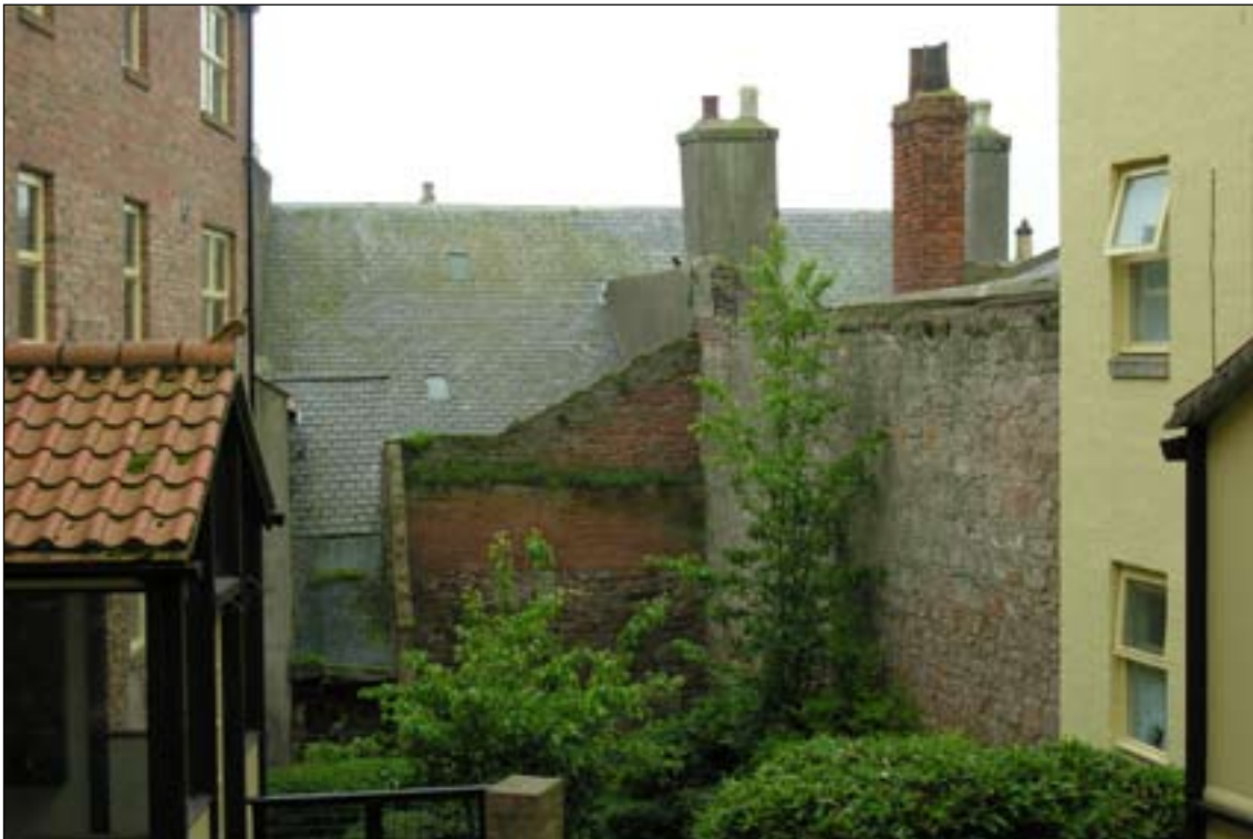
Fig. 60: The rear wall of the rear range and the roof of the principal range of 57 West Street / 64-66 Bridge Street as seen from Easter Wynd. DP065410 © English Heritage
