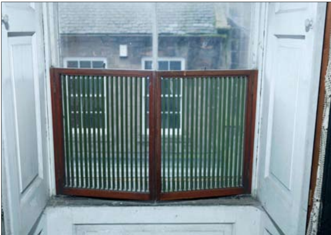
Fig. 80: Dwarf blinds (open) in one of the windows of the largest second-floor room at 64-66 Bridge Street / 57 West Street. DP065386 © English Heritage
