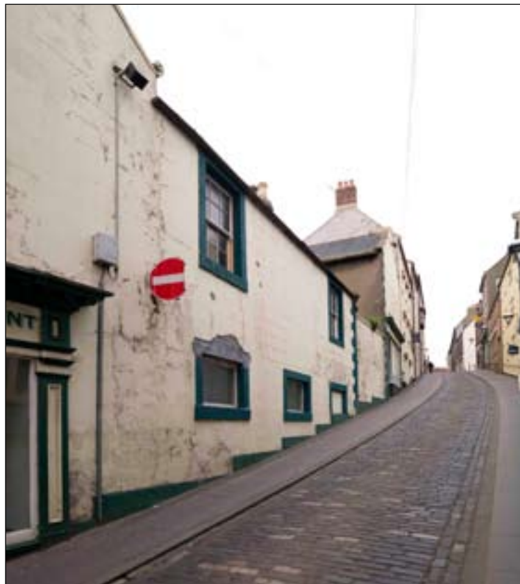
Fig. 34: The billiard room with bedrooms above, added to the rear of 2 Love Lane / 64 West Street. This addition faces onto West Street. DP065337 © English Heritage
