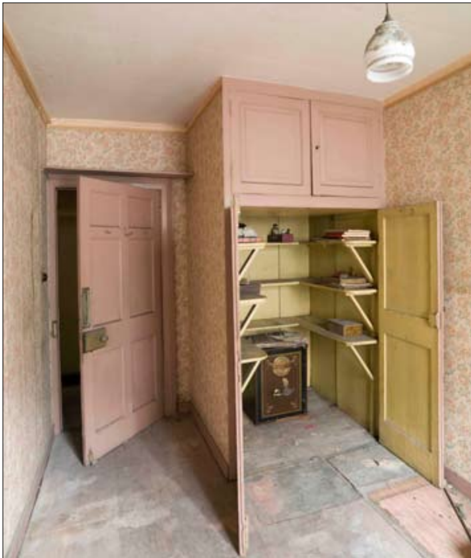
Fig. 64: The small first-floor room east of the stair at 57 West Street / 64-66 Bridge Street. DP065371 © English Heritage
