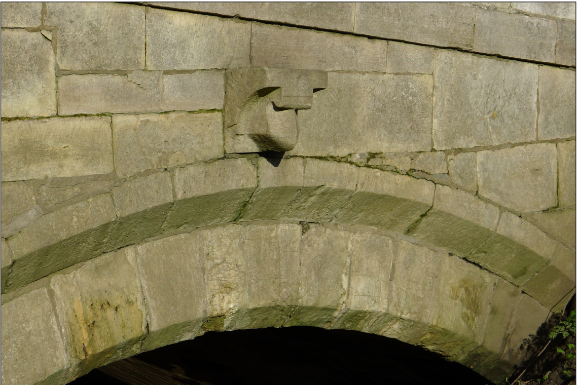
Figure 4: Detail of the downstream arch ring and archivolt of arch 1, showing also the corbel over the crown and the early string course rising at an angle above it. (AF00398021 © Historic England/Lucy Jessop).
