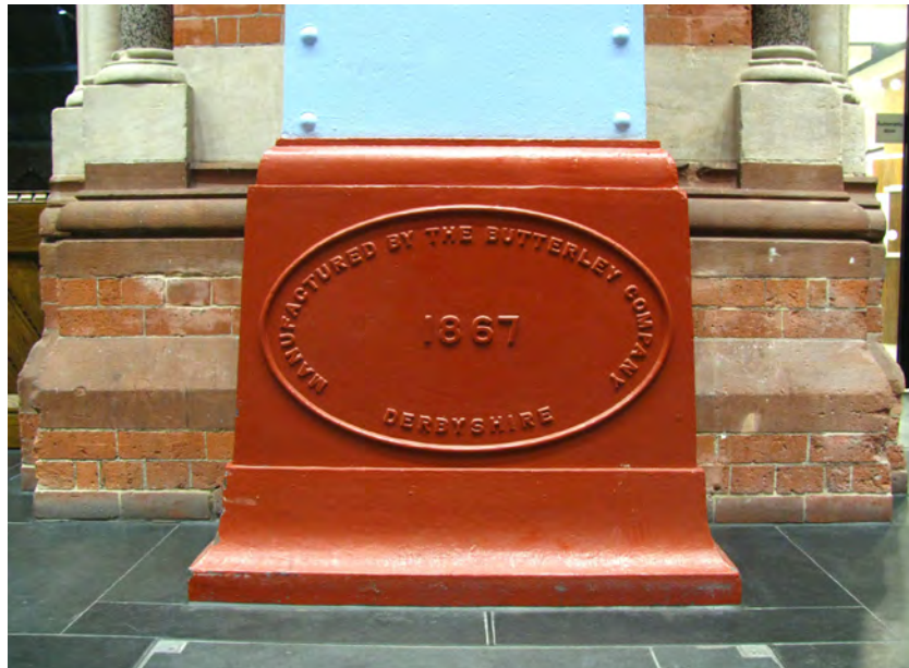
Figure 21: The Butterley Company stamp at the foot of one of the iron roof spans at St Pancras Station. Photographed by Rebecca Pullen, © English Heritage
