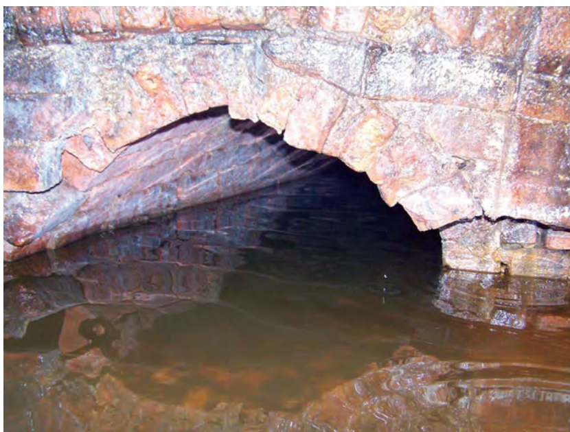
Figure 12: Low entrance to blast receiver passage in north wall of tunnel, looking north (after Cordon 2006, image 59), © Tina Cordon, reproduced with permissions
