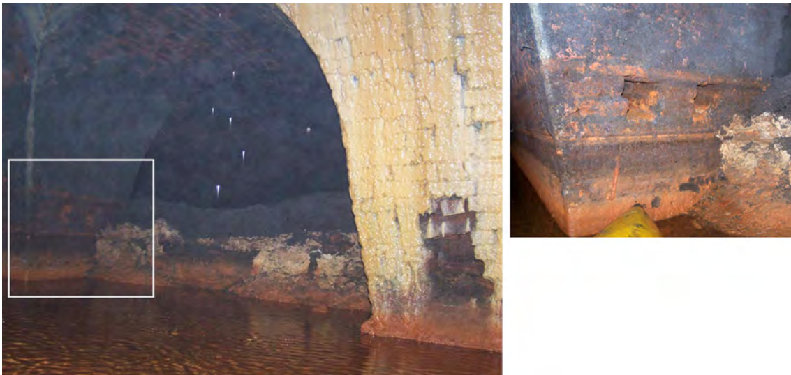
Figure 11: Rectangular recesses in the brickwork, main personnel unloading point, looking south-east (after Cordon 2006, images 67 and 69), © Tina Cordon, reproduced with permissions
