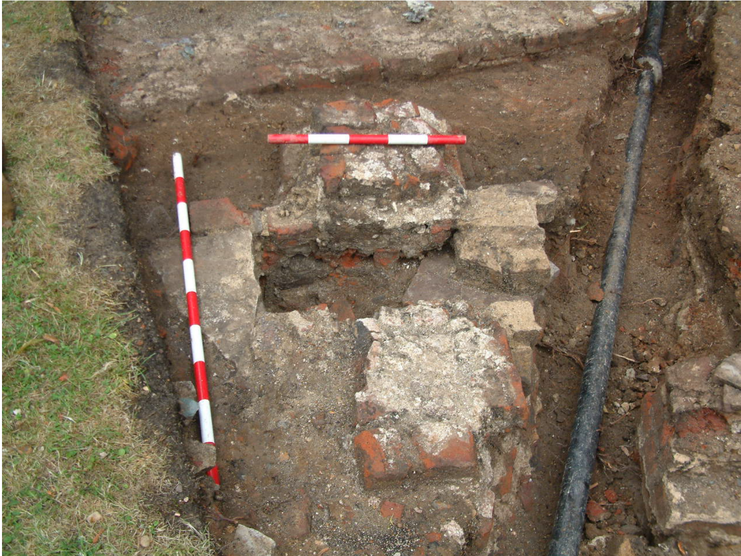
Plate 8 View of Trench 2B showing the cut for a lead water pipe, looking west (1m and 0.5m scales)
