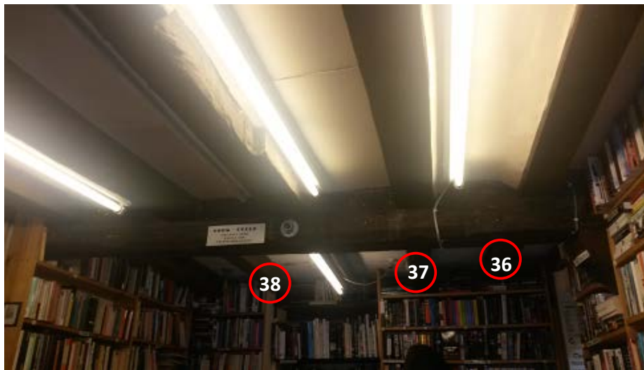
Figure 5e/f: Section through truss 2 of the western building (top, after Dunkley and Templeton in Dunkley et al 1985), and annotated photograph of ground floor ceiling timbers to 7 West Street (bottom) to show sampled timbers (photograph Robert Howard)
