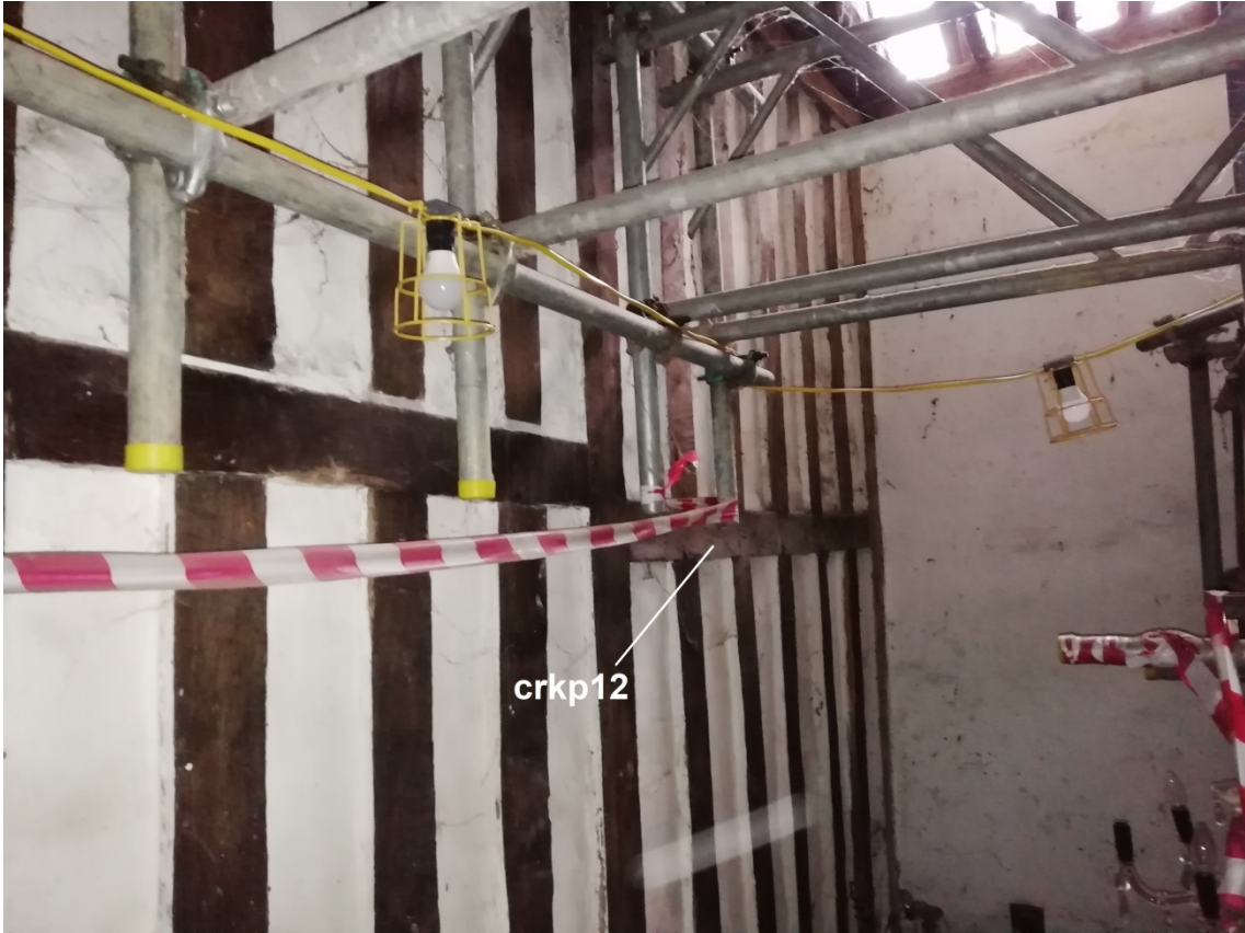
Figure 7: View of the north-west corner of the first-floor east-most room of the north range, showing the mid-rail sampled for dendrochronology (photograph Martin Bridge)
