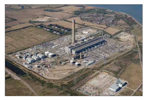
Isle of Grain, Medway, Uniper UK, to left is the Combined Cycle Gas Turbine a Combined Heat Power station during construction in 2009. The unit with the shorter chimney is the Open Cycle Gas Turbine plant; the larger oil-fired station has subsequently been demolished. © Historic England 26477/020 (2009)
