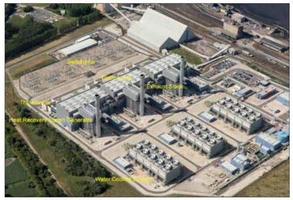
Figure 4. West Burton, Nottinghamshire, Combined Cycle Gas Turbine station showing its principal components. © Historic England 29953/048 (2016)
