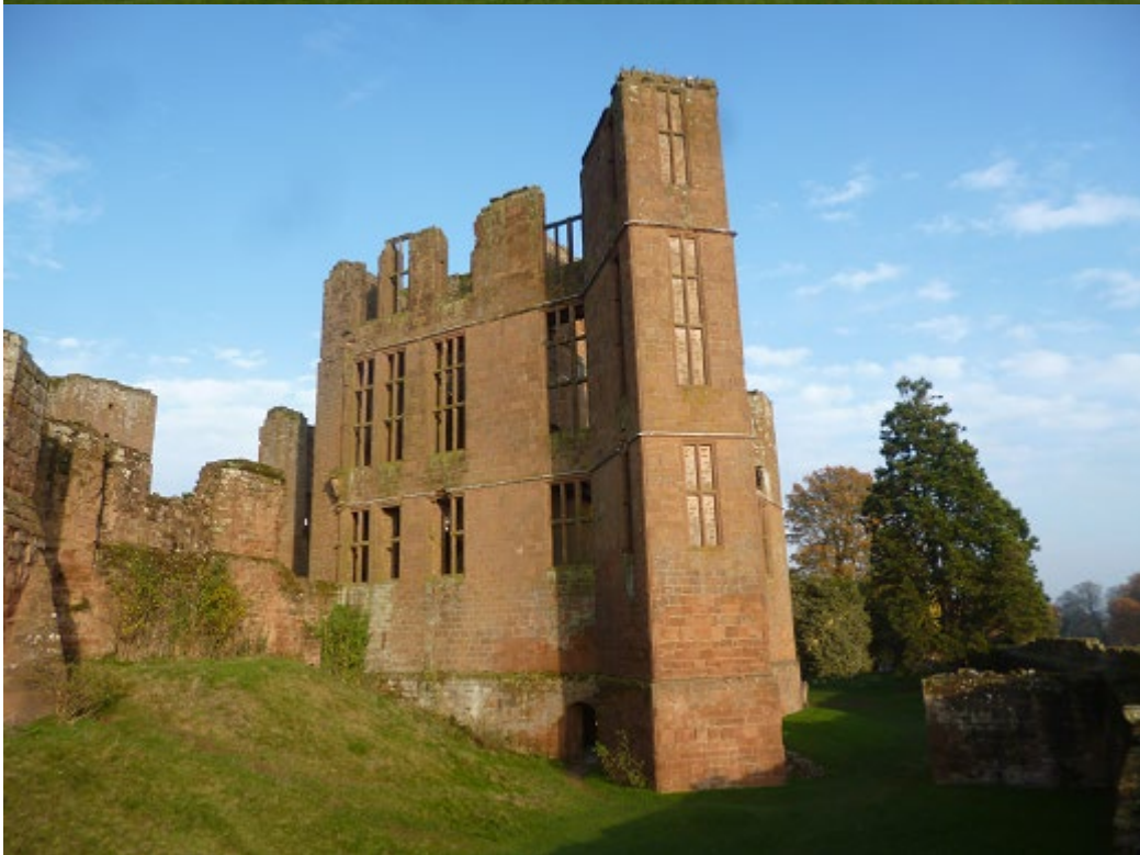
Figure 2a/b: Views of Leicester's Building from the east (top) and the southwest (bottom) (photographs Robert Howard)
