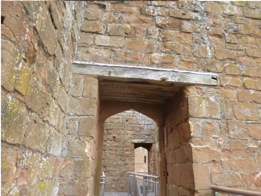
Figure 3a/b: Views showing examples of door lintels (photographs Robert Howard)
