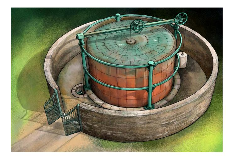
Figure 6 (top): The gasholder at the former Dolphinholme Worsted works as it may have looked in around 1820 after its construction following a major extension of the mill in 1818. The remains of the holder, comprising the circular stone tank, rubble stone wall and counterweight form part of what is thought to be the world's earliest surviving gasworks. © Historic England
