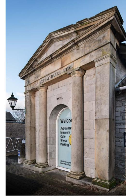
Figure 14: The façade of the original Kendal Gas Company meter house. Constructed in 1825, the façade comprises a pedimented portico carried on a pair of Tuscan columns and flanked by square corner pilasters and bears the inscription 'EX FUMO DARE LUCEM' which translates as 'Light from Smoke'. The façade was removed from its original gasworks location in 1984 and reconstructed as the west elevation of the extension to the Museum of Lakeland Life and Industry. [DP249853]
