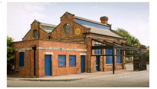
Figure 12: The former estate gasworks (later a blacksmiths) built in 1874 to serve Sudbury Hall in Derbyshire. Like many small estate gas works, the Sudbury gasworks were given the architectural embellishments of the other estate buildings, in this case blue brick diaper patterning and Flemish gables. The former retort house (rear) retains its chimney and characteristic clerestory. © Mr Geoffrey R Hood. Source: Historic **England Archive**
