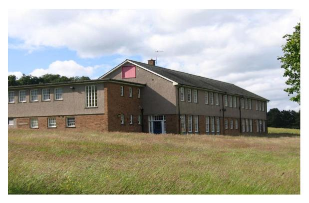
Figure 19.1 The buildings of the Boys' Village (1958) to the north are set in an arc overlooking the playing field of 1949, the site of which is associated with the most prominent area of terracing. The style of the buildings – including Tredgold Hall built for occupational classes to the west – is loosely classical and domestic, with sash windows and Westmorland slate roofs.
