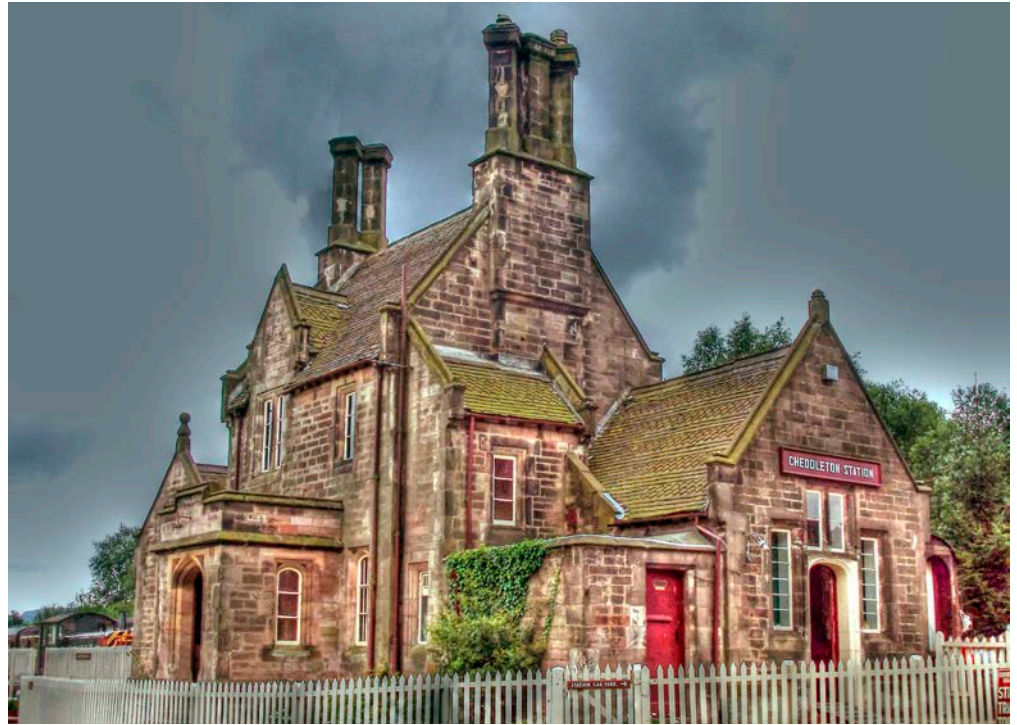
Figure 7: Station building, Cheddleton. Millstone Grit Group sandstone.
