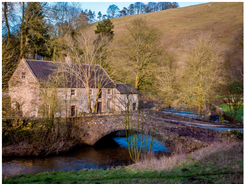
Figure 5: Lode Mill Bridge, Alstonefield. Limestone rubble.
