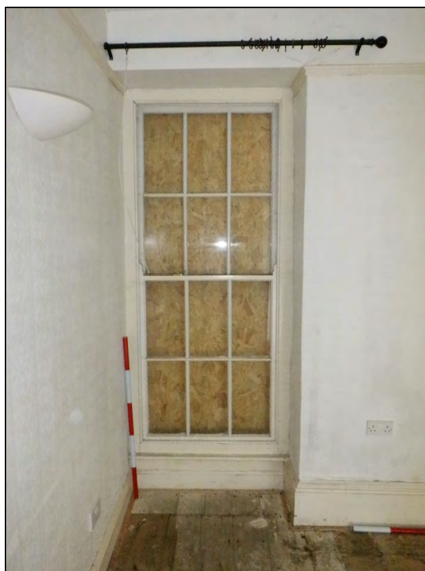
Plate 137: 2 Penrose Terrace, Room 2G1, view to the S. 2 x 1m scale.
