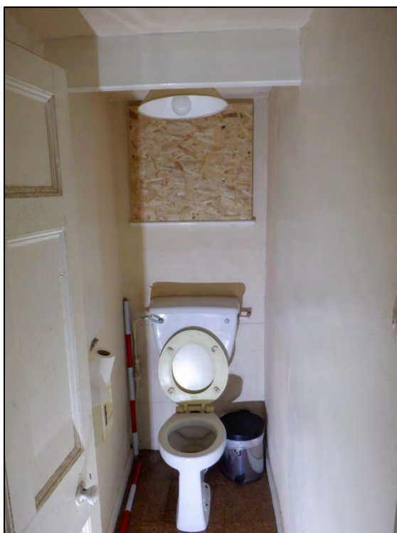
Plate 162: 2 Penrose Terrace, Room 2F6, view to the N. 2 x 1m scale.
