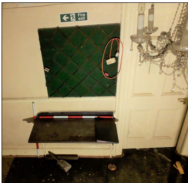
Plate 32: 1 Penrose Terrace, Room 1G3, view to the E. 2 x 1m scale.
