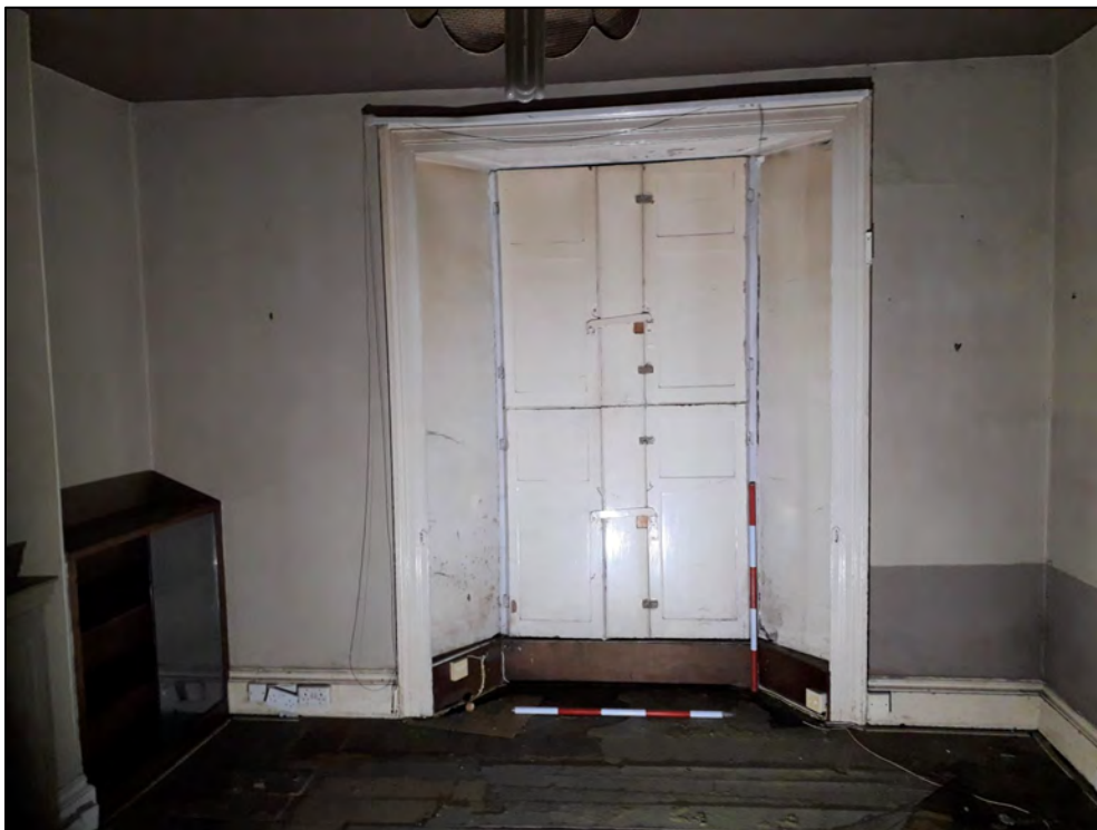
Plate 37: 1 Penrose Terrace, Room 1G2, view to the E. 2 x 1m scale.
