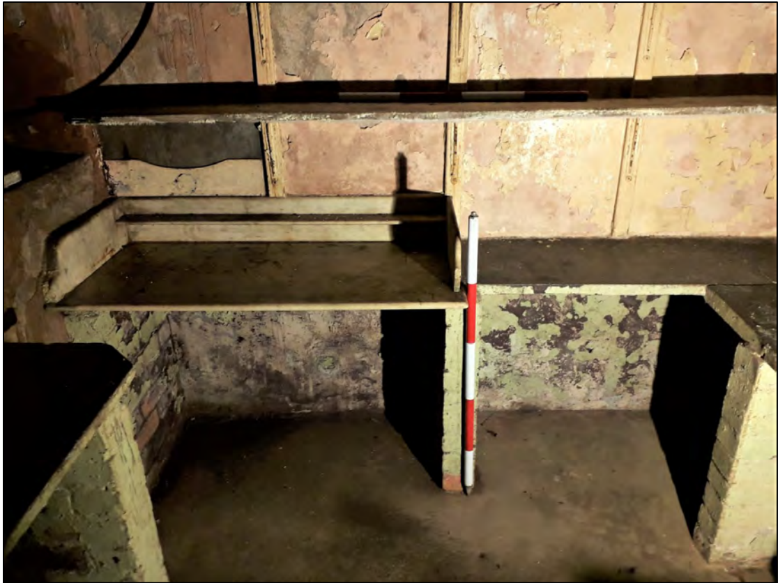
Plate 88: 1 Penrose Terrace, Room 1B5, view to the N. 1m scale.
