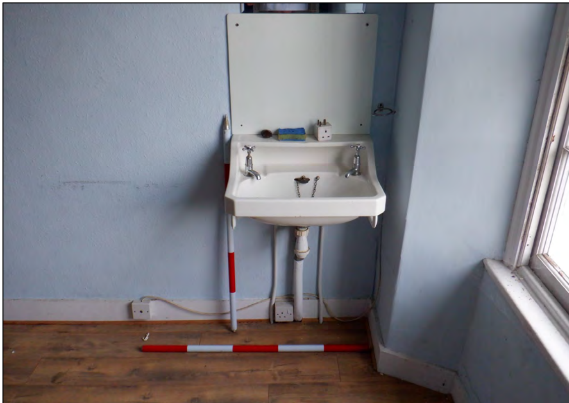
Plate 151: 2 Penrose Terrace, Room 2F1, view to the ESE. 2 x 1m scale.
