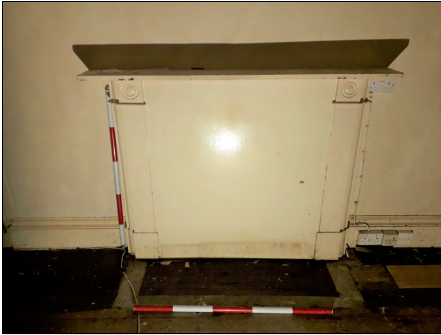
Plate 40: 1 Penrose Terrace, Room 1G1, view to the N. 2 x 1m scale.
