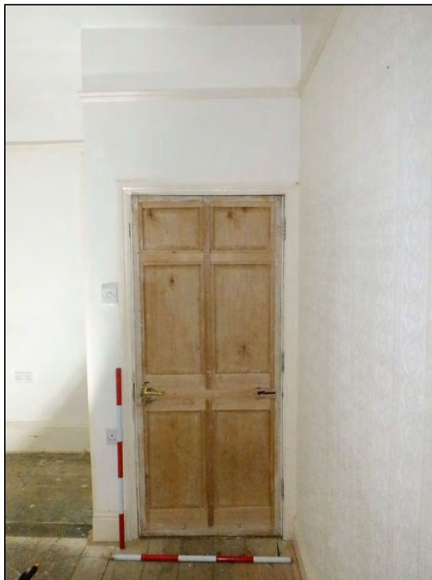
Plate 135: 2 Penrose Terrace, Room 2G1, view to the N. 2 x 1m scale.
