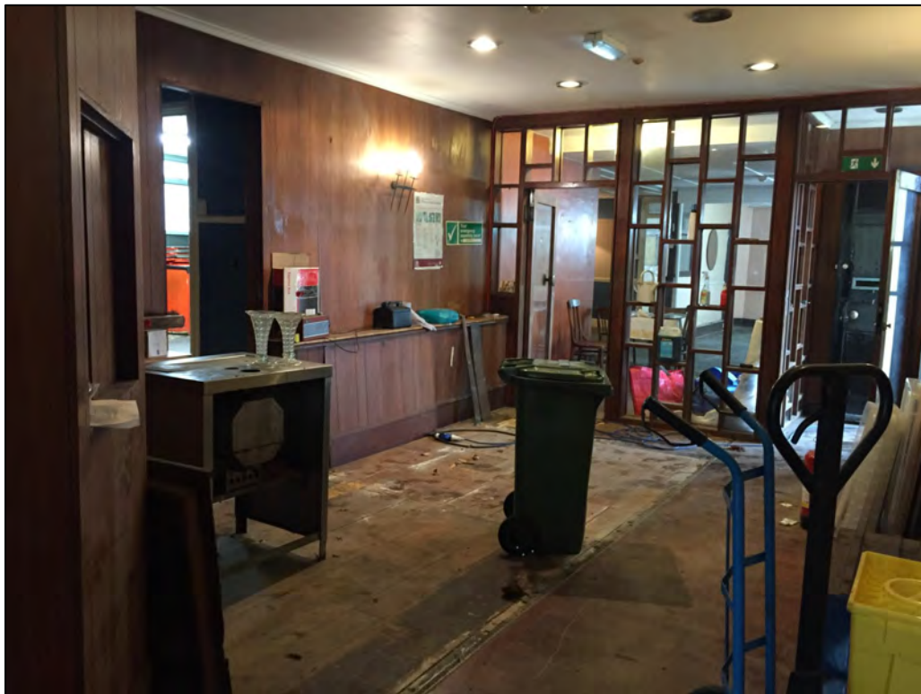
Plate 16: 1 Penrose Terrace, Room 1G7, view to the ENE. Image supplied by CAD Heritage.
