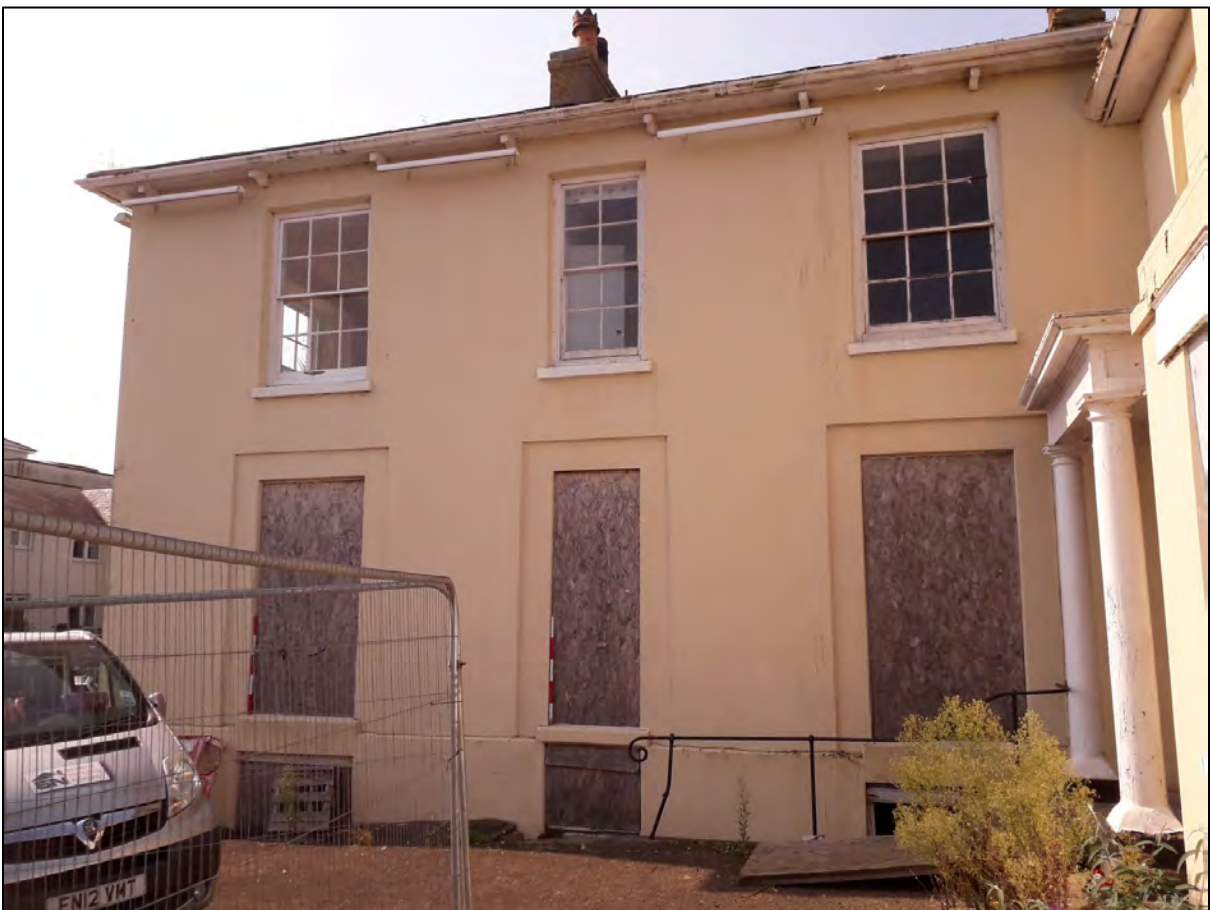
Plate 10: 1 Penrose Terrace, east elevation of South Wing, view to the West, 2 x 1m scale.
