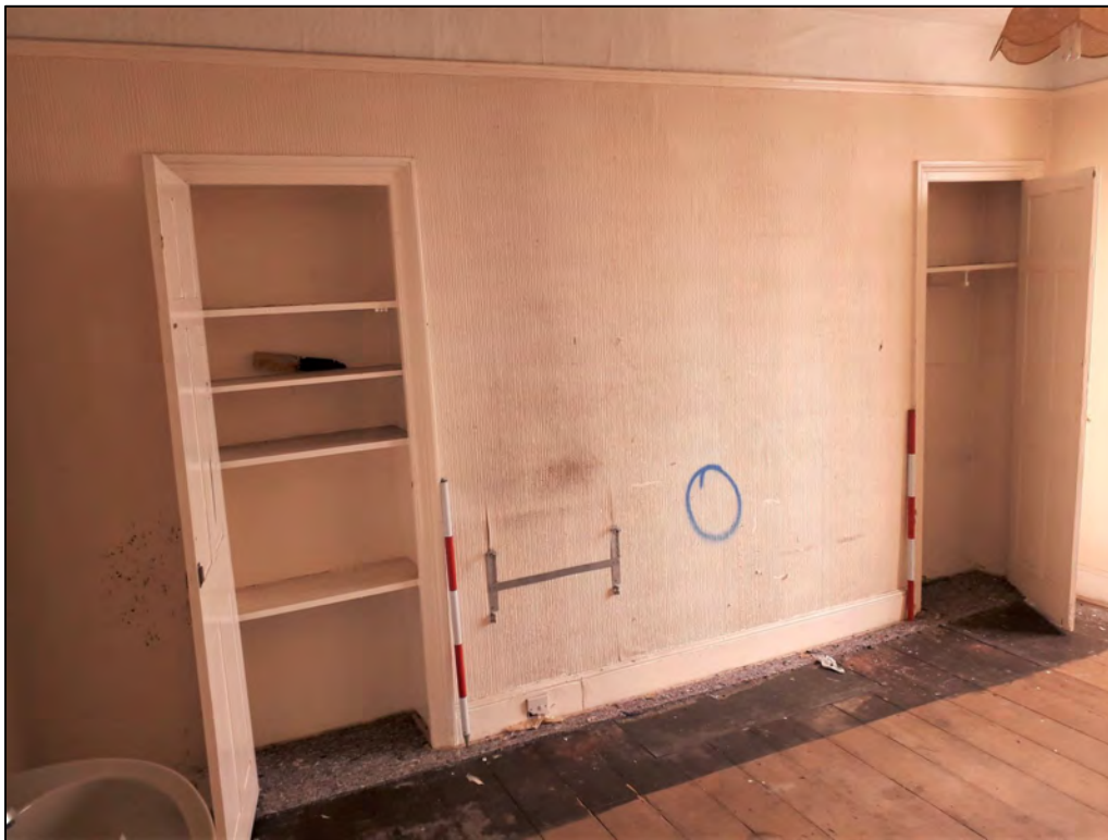
Plate 57: 1 Penrose Terrace, Room 1F8, view to the NE. 2 x 1m scale.
