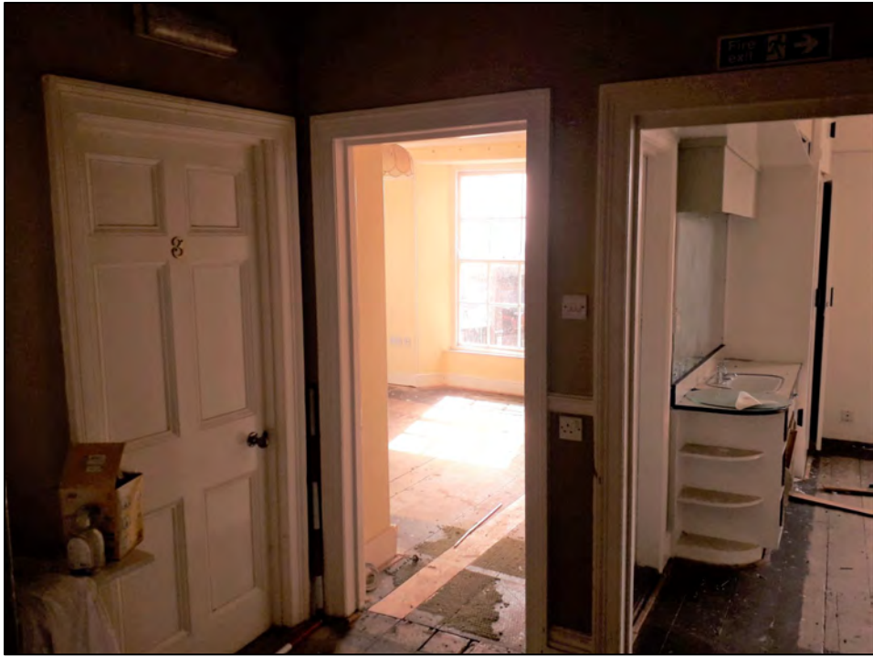
Plate 46: 1 Penrose Terrace, Room 1F4, view to the SE. 2 x 1m scale.
