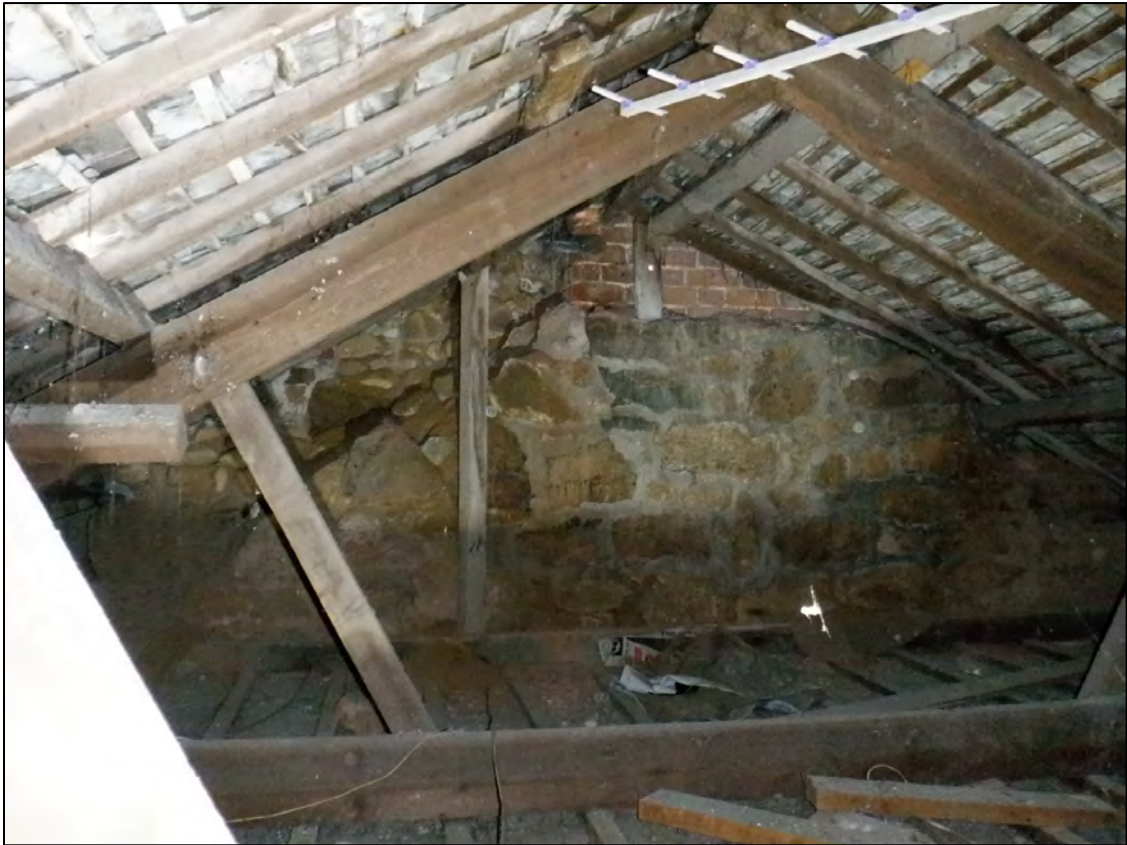
Plate 164: 2 Penrose Terrace, Roof Space, East Gable End, view to the E.
