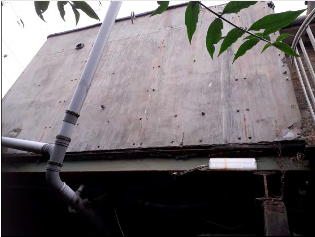
Plate 114: 1 Penrose Terrace, External Rear Yard, view to the ENE.
