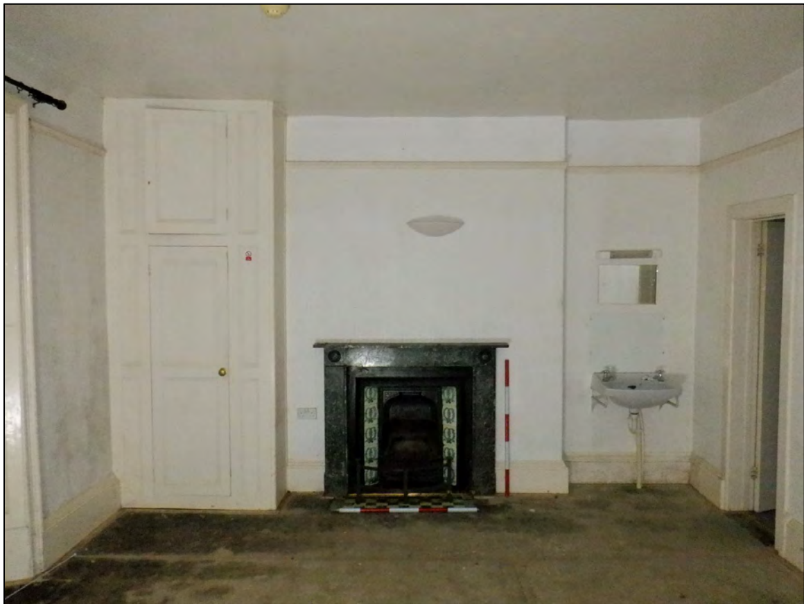
Plate 133: 2 Penrose Terrace, Room 2G1, view to the W. 2 x 1m scale.
