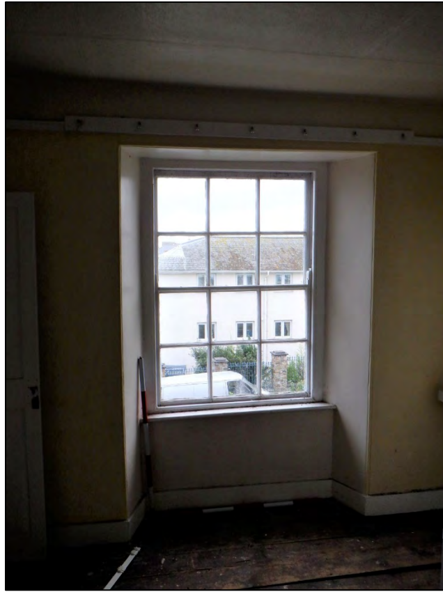
Plate 158: 2 Penrose Terrace, Room 2F3, view to the SSW. 2 x 1m scale.
