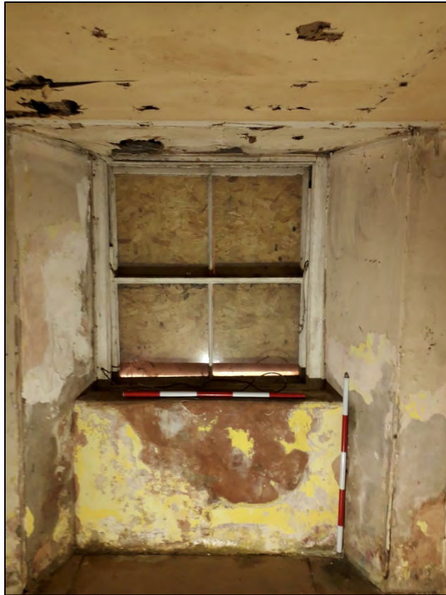
Plate 104: 1 Penrose Terrace, Room 1B2, view to the E. 2 x 1m scale.
