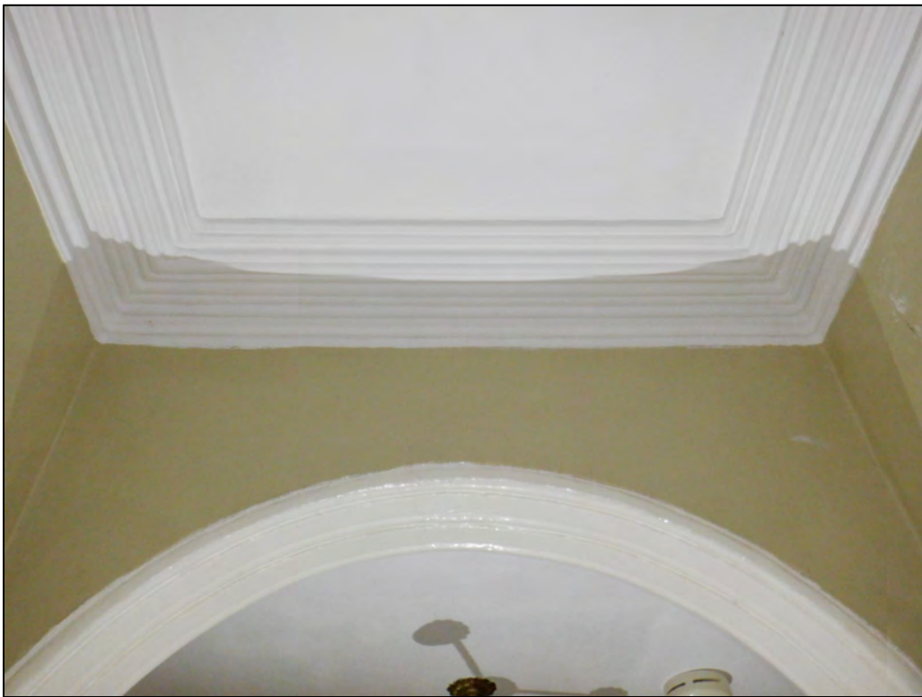
Plate 123: 2 Penrose Terrace, Room 2G5 (anteroom), view to the N.
