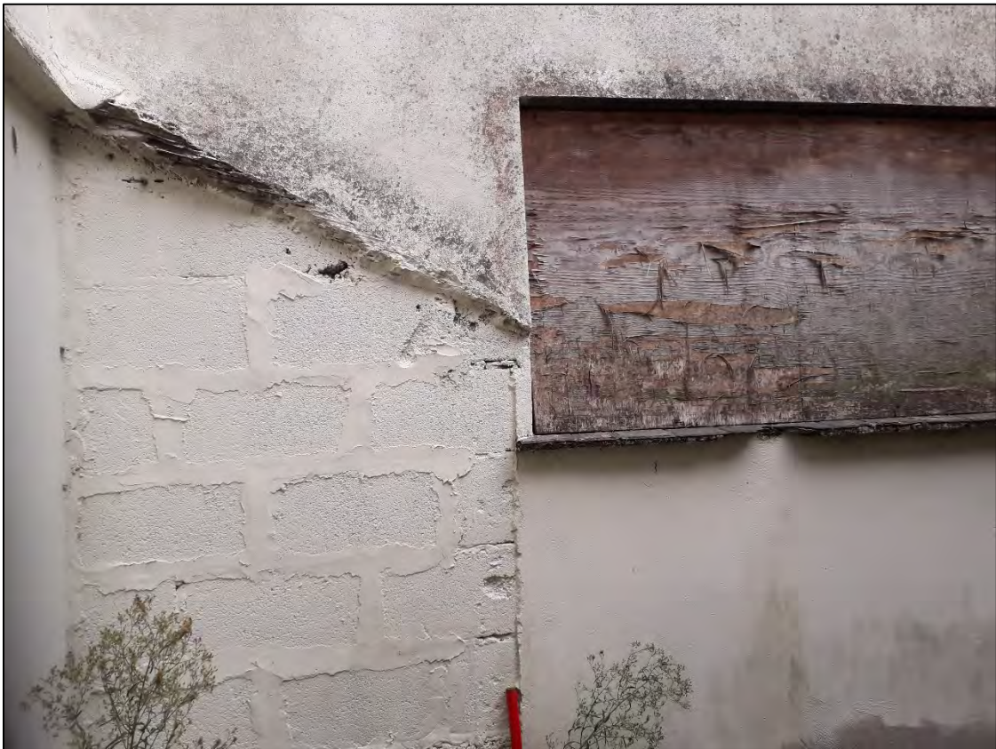
Plate 169: 2 Penrose Terrace, External Rear Yard, view to the N. 1m scale
