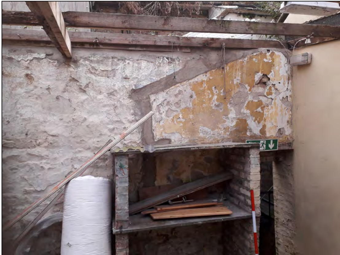
Plate 167: 2 Penrose Terrace, External Rear Yard, view to the ESE. 1m scale
