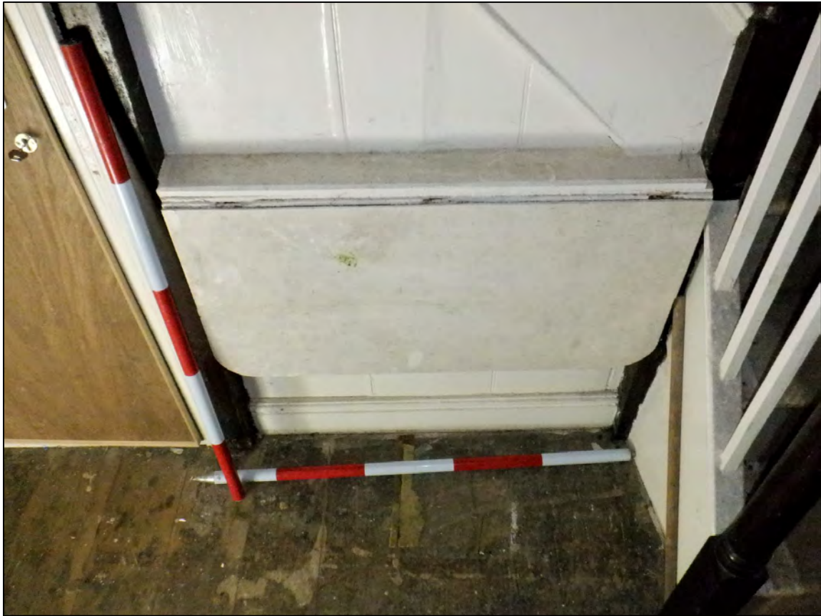
Plate 128: 2 Penrose Terrace, Room 2G5, view to the N. 2 x 1m scale.
