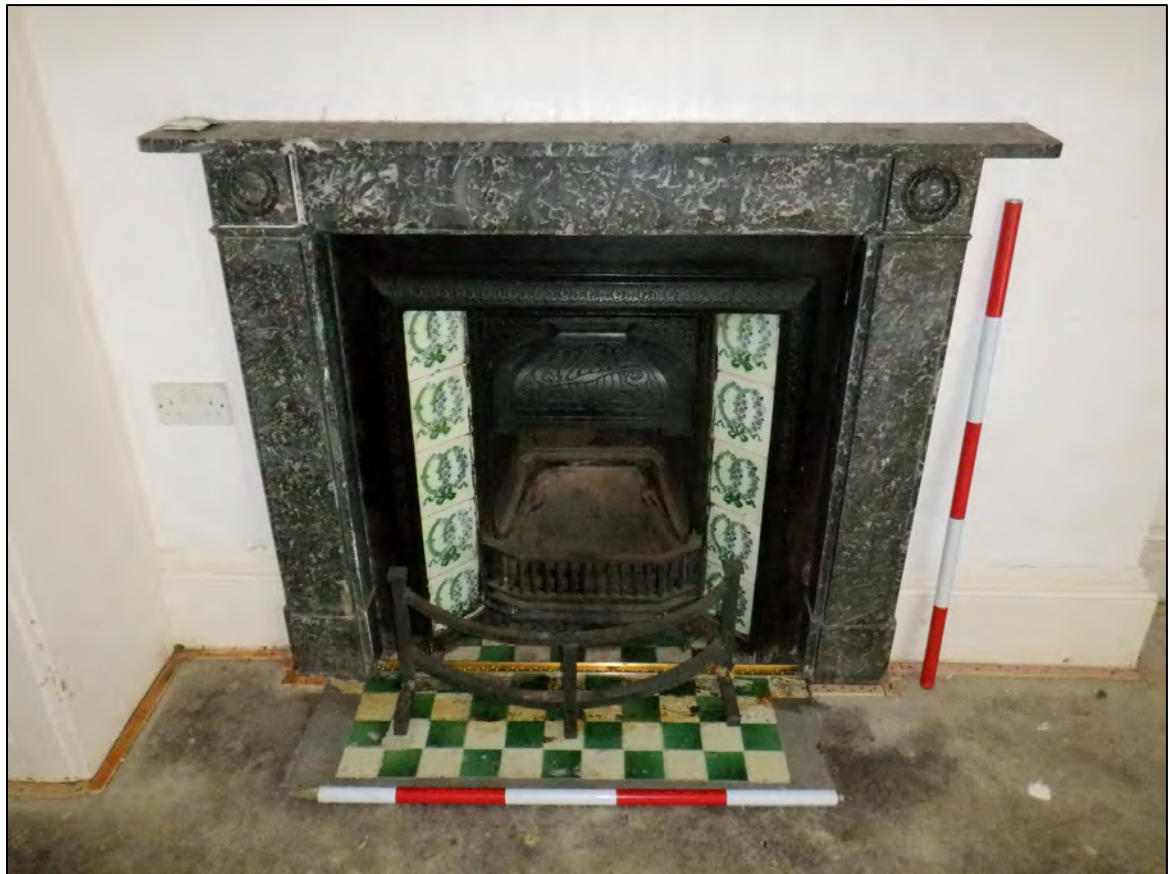
Plate 138: 2 Penrose Terrace, Room 2G1, view to the W. 2 x 1m scale.
