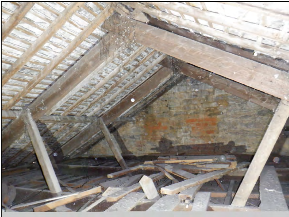
Plate 165: 2 Penrose Terrace, Roof Space, West End, view to the W.
