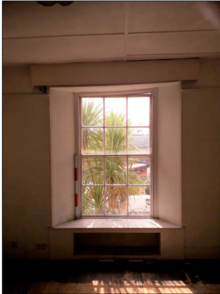
Plate 50: 1 Penrose Terrace, Room 1F1, view to the S. 2 x 1m scale.
