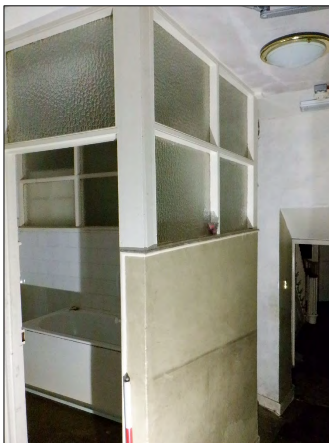
Plate 141: 2 Penrose Terrace, Room 2G7, view to the ENE. 1m scale.
