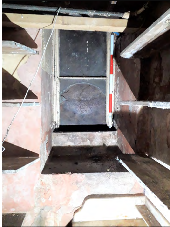
Plate 90: 1 Penrose Terrace, Room 1B5, view to the W. 1m scale.
