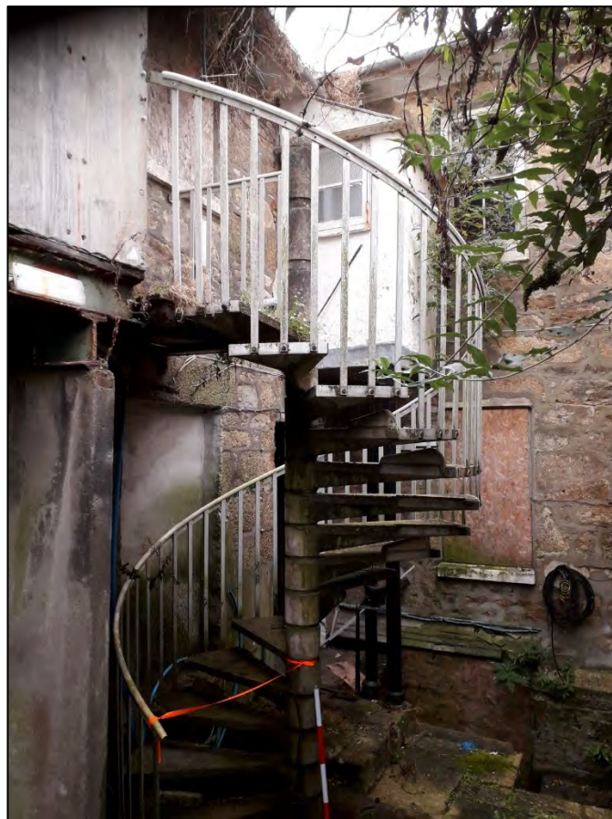
Plate 111: 1 Penrose Terrace, External Rear Yard, view to the SSE. 1m scale.
