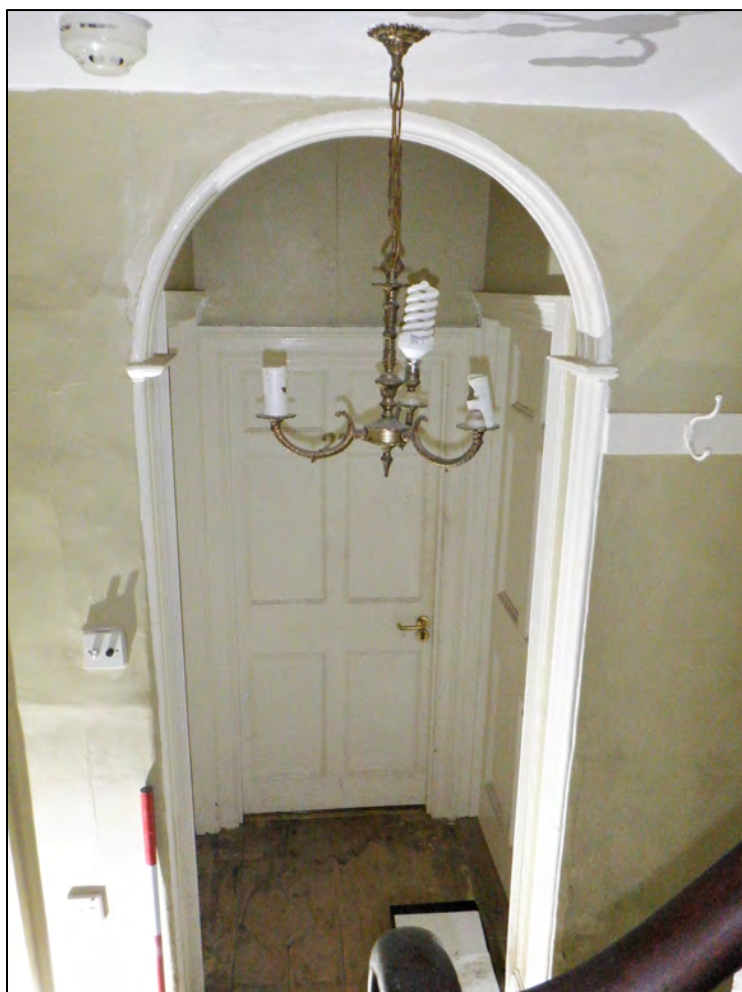
Plate 124: 2 Penrose Terrace, Room 2G5, view to the S. 1m scale
