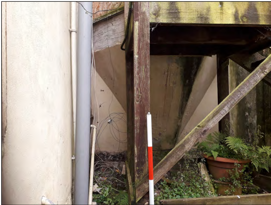
Plate 121: 2 Penrose Terrace, North Facing Elevation, view to the S. 1m scale.
