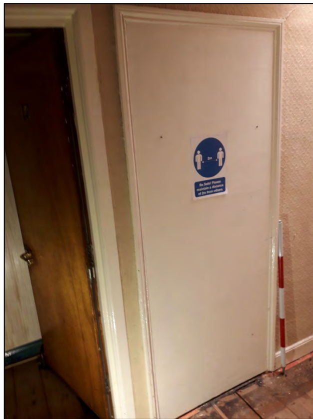
Plate 71: 1 Penrose Terrace, Room 1F10, view to the SE. 1m scale.
