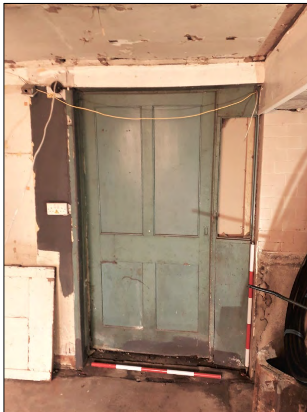
Plate 103: 1 Penrose Terrace, Room 1B4, view to the W. 2 x 1m scale.
