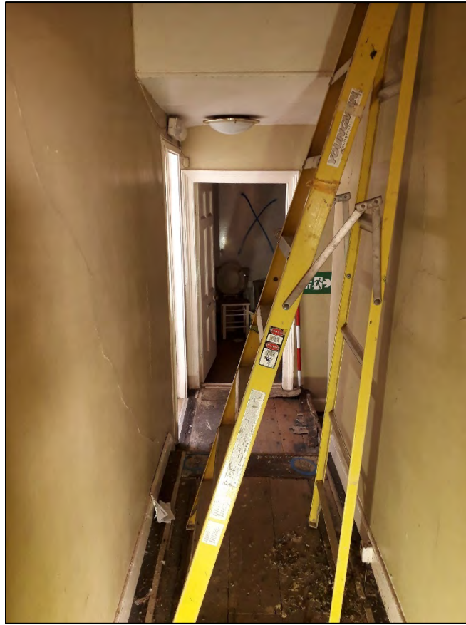
Plate 62: 1 Penrose Terrace, Room 1F10, view to the N. 1m scale.
