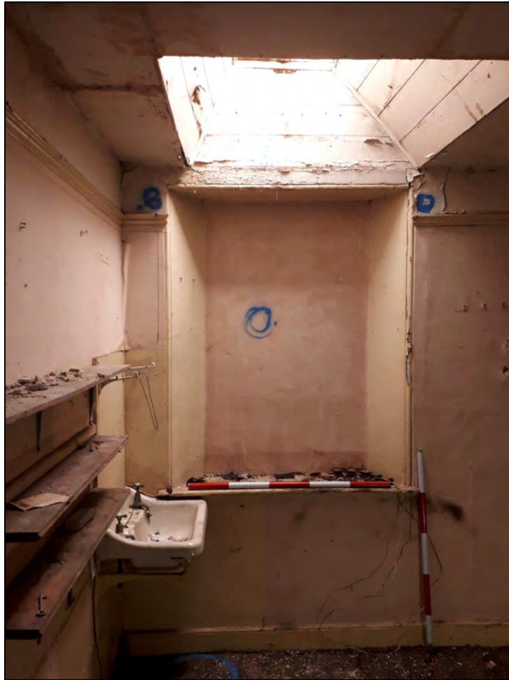
Plate 66: 1 Penrose Terrace, Room 1F12, view to the N. 2 x 1m scale.
