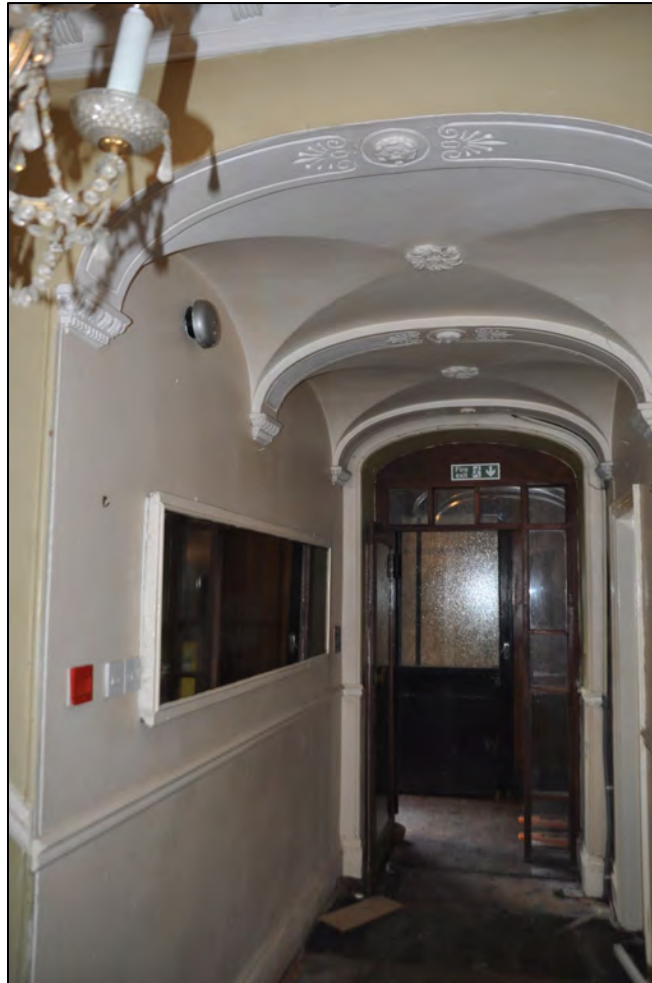
Plate 28: 1 Penrose Terrace, Room 1G3, view to the N. Image supplied by CAD Heritage
