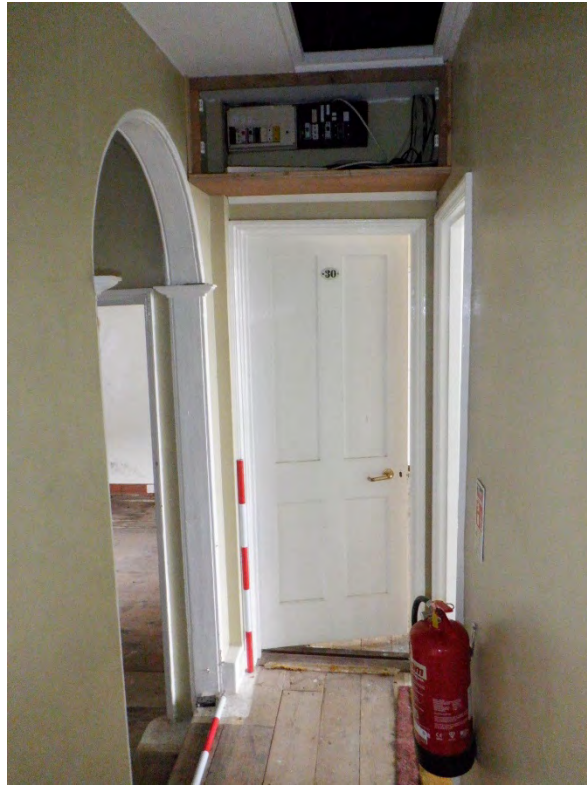
Plate 148: 2 Penrose Terrace, Room 2F4, view to the E. 2 x 1m scale.
