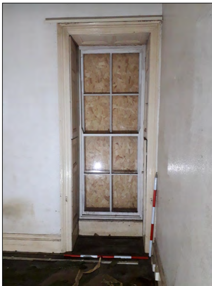
Plate 34: 1 Penrose Terrace, Room 1G5, view to the E. 2 x 1m scale.
