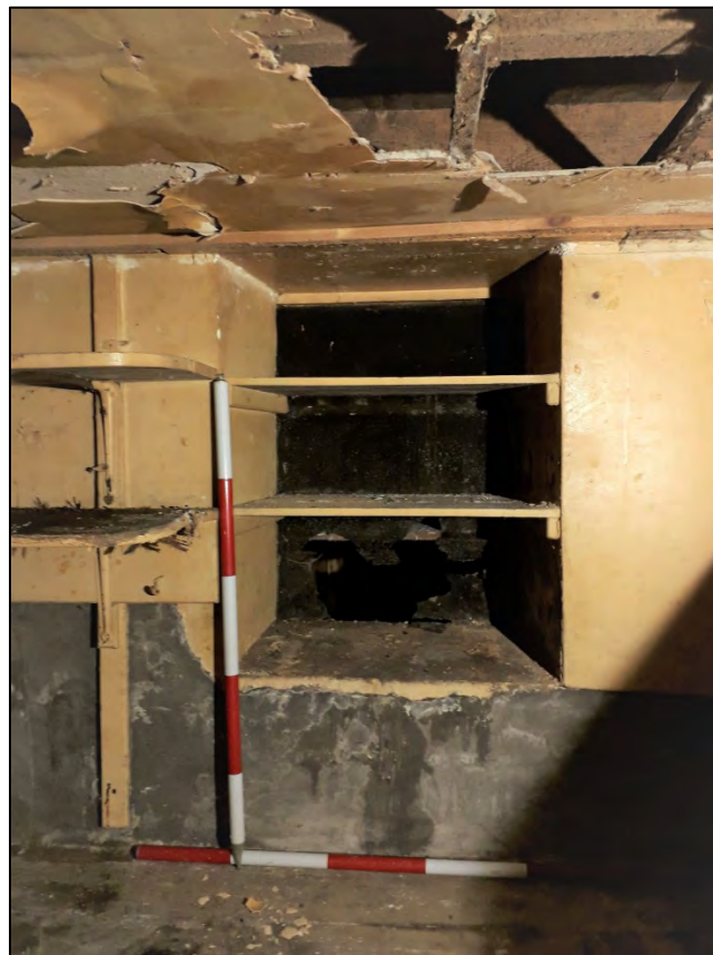
Plate 93: 1 Penrose Terrace, Room 1B6, view to the W. 2 x 1m scale.
