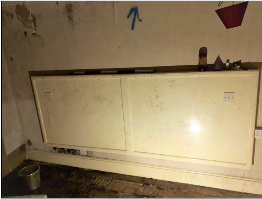
Plate 74: 1 Penrose Terrace, Room 1F15, view to the ENE. 1m scale.
