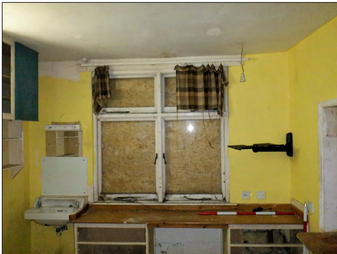
Plate 143: 2 Penrose Terrace, Room 2G8, view to the W. 2 x 1m scale.
