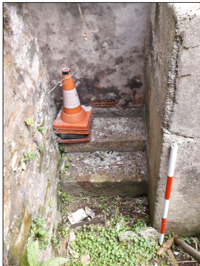
Plate 113: 1 Penrose Terrace, External Rear Yard, view to the E. 1m scale.
