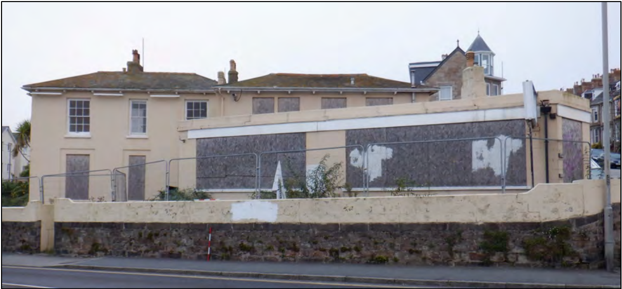
Plate 9: 1 Penrose Terrace, east elevation, view to the West, 1m scale.
