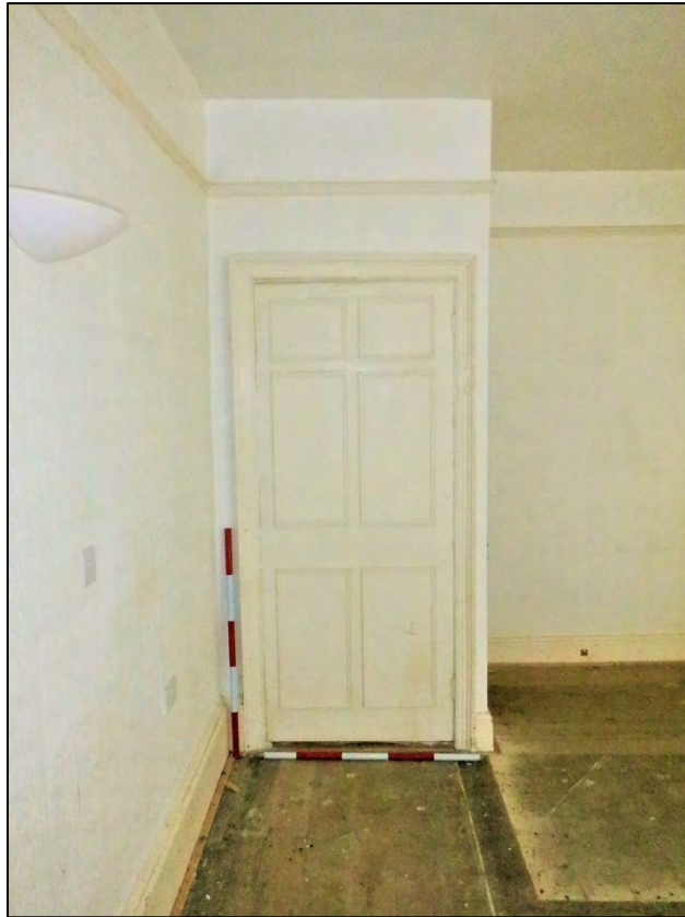
Plate 134: 2 Penrose Terrace, Room 2G1, view to the E. 2 x 1m scale.
