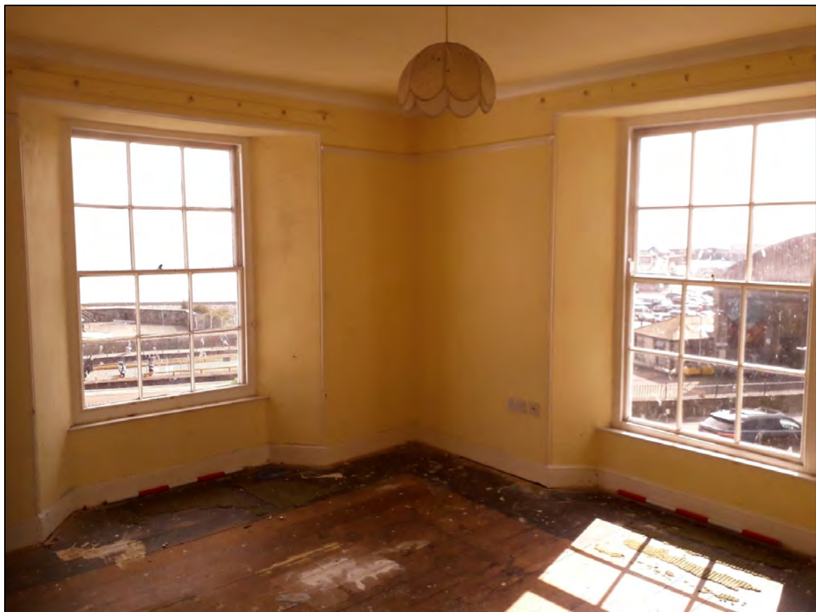
Plate 53: 1 Penrose Terrace, Room 1F2, view to the SE. 2 x 1m scale.
