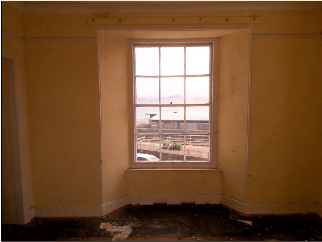
Plate 54: 1 Penrose Terrace, Room 1F2, view to the E. 1m scale.
