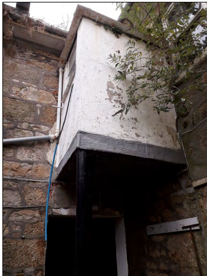
Plate 115: 1 Penrose Terrace, External Rear Yard, view to the ESE.
