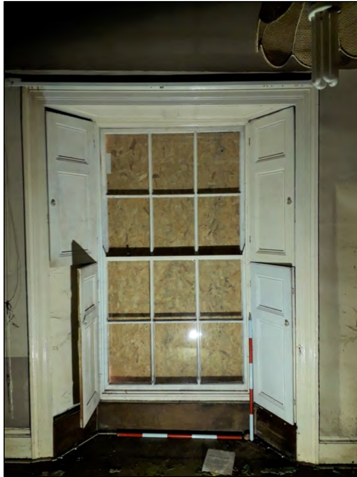
Plate 36: 1 Penrose Terrace, Room 1G2, view to the S. 2 x 1m scale.
