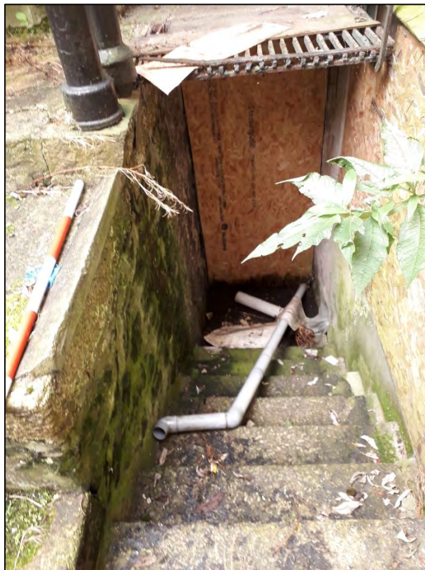
Plate 109: 1 Penrose Terrace, External Rear Yard, view to the E. 1m scale.
