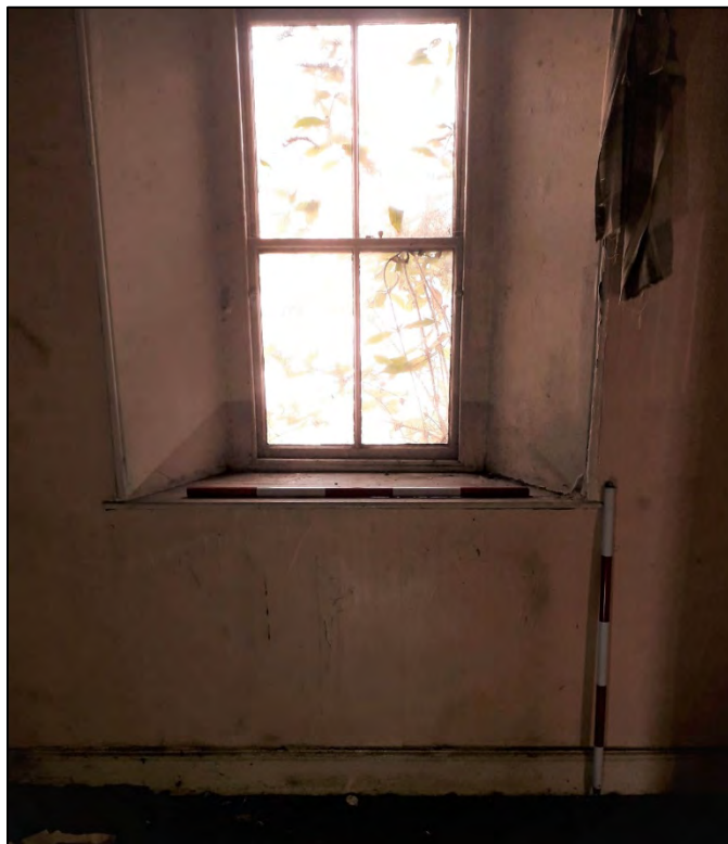
Plate 61: 1 Penrose Terrace, Room 1F7, view to the N. 2 x 1m scale.
