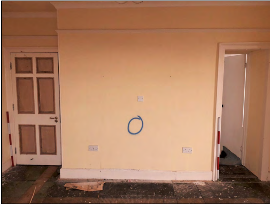
Plate 52: 1 Penrose Terrace, Room 1F2, view to the N. 2 x 1m scale.
