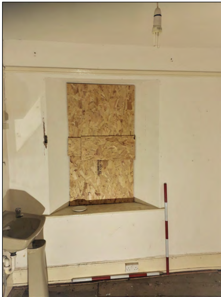
Plate 75: 1 Penrose Terrace, Room 1F16, view to the N. 2 x 1m scale.
