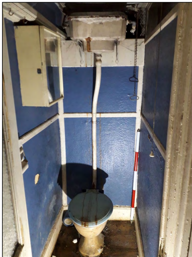
Plate 22: 1 Penrose Terrace, Room 1G10, view to the W. 1m scale.
