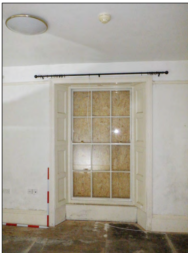
Plate 136: 2 Penrose Terrace, Room 2G1, view to the S. 2 x 1m scale.
