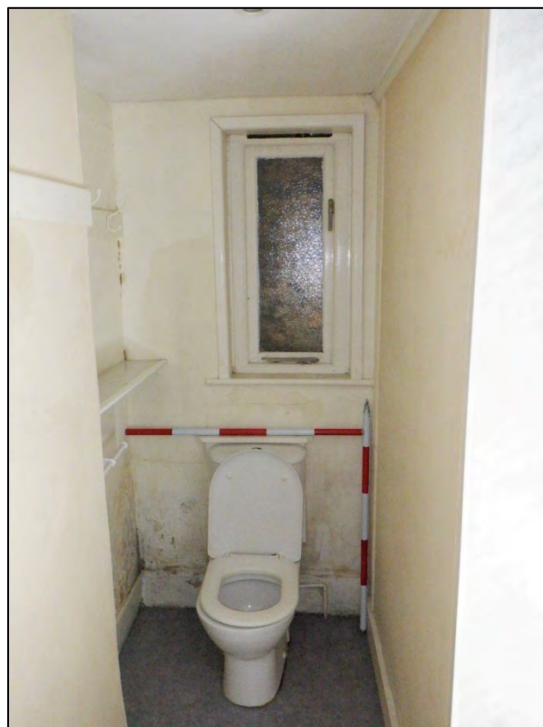
Plate 139: 2 Penrose Terrace, Room 2G3, view to the N. 2 x 1m scale.
