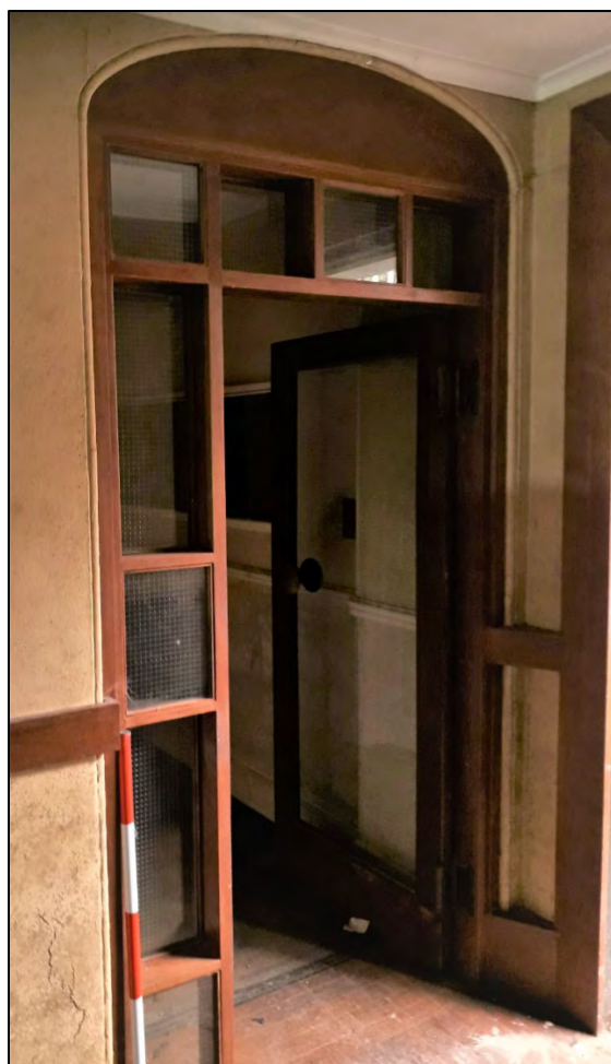
Plate 17: 1 Penrose Terrace, Room 1G7, view to the SW. 1m scale.
