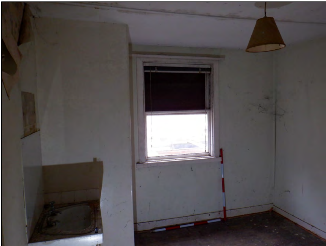
Plate 161: 2 Penrose Terrace, Room 2F10, view to the WNW. 2 x 1m scale.
