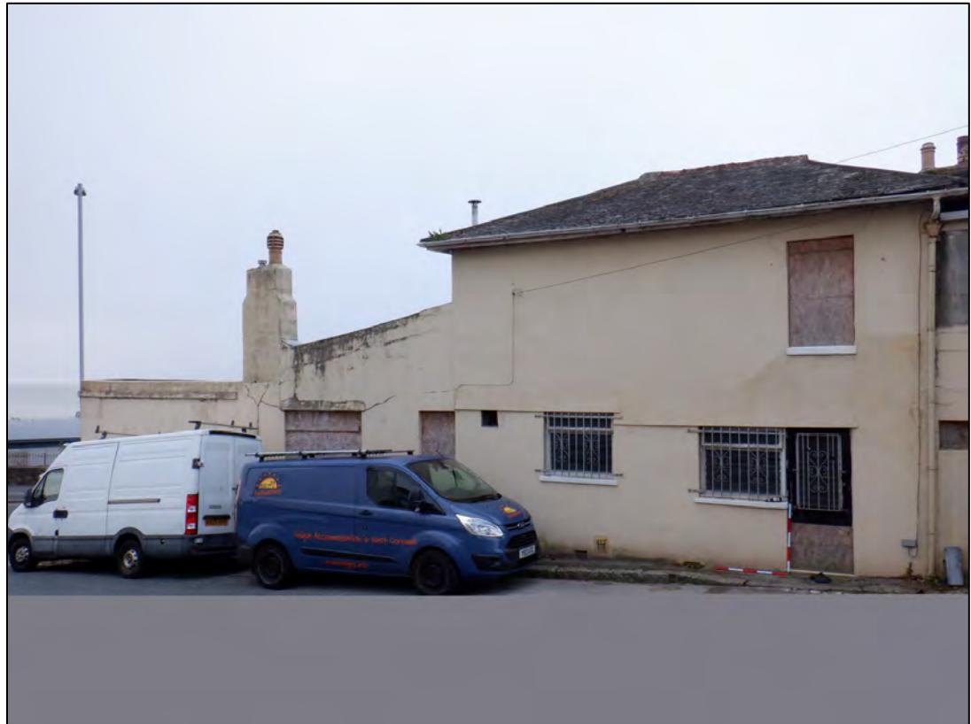
Plate 14: 1 Penrose Terrace, north elevation of north wing and NE Annexe, view to the SSE, 2 x 1m scale.
