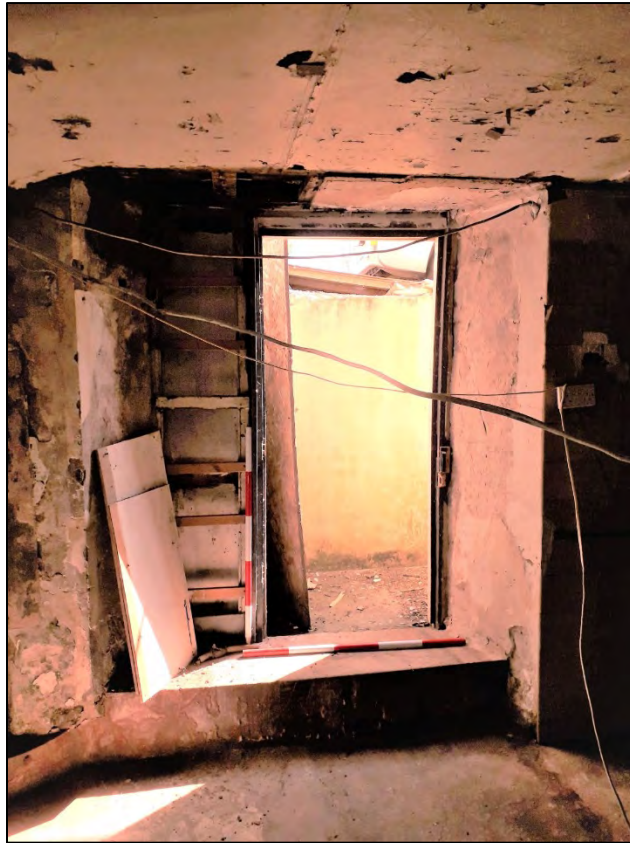
Plate 102: 1 Penrose Terrace, Room 1B4, view to the E. 2 x 1m scale.
