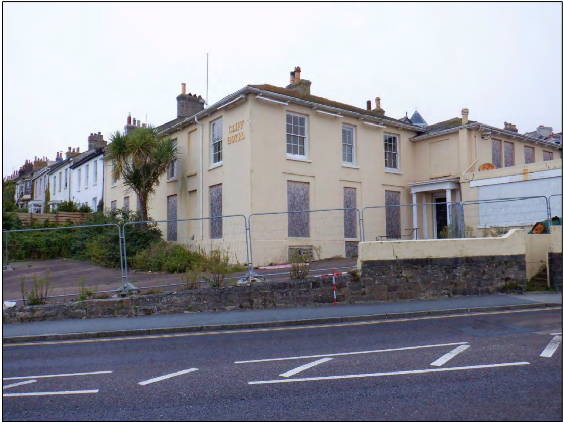
Plate 1: The former Cliff Hotel viewed from Chyandour Cliff, looking north-west. 1m & 1m scale.
