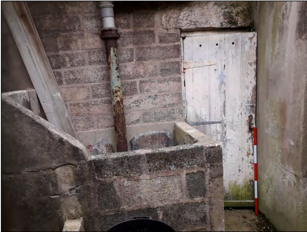
Plate 110: 1 Penrose Terrace, External Rear Yard, view to the ESE. 1m scale.
