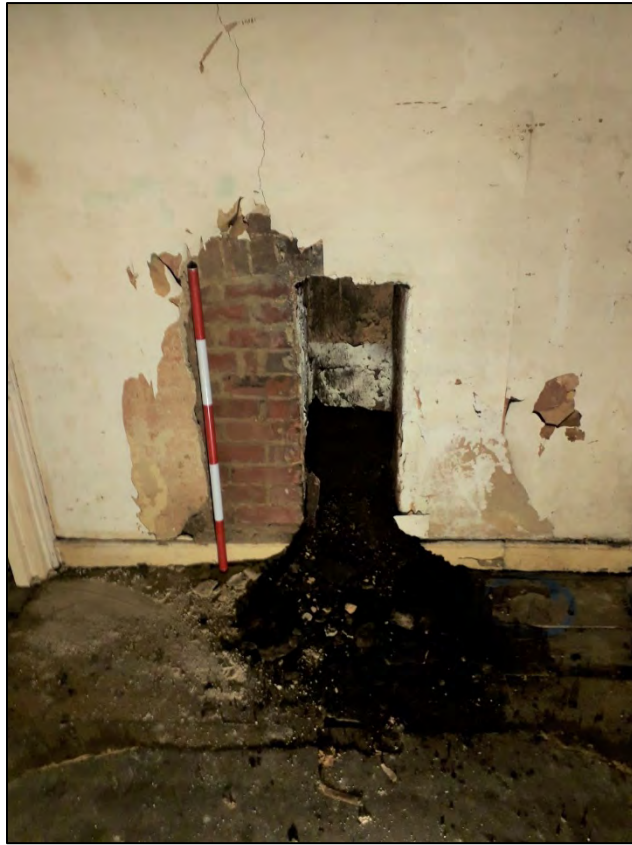
Plate 42: 1 Penrose Terrace, Room 1G4, view to the W. 1m scale.
