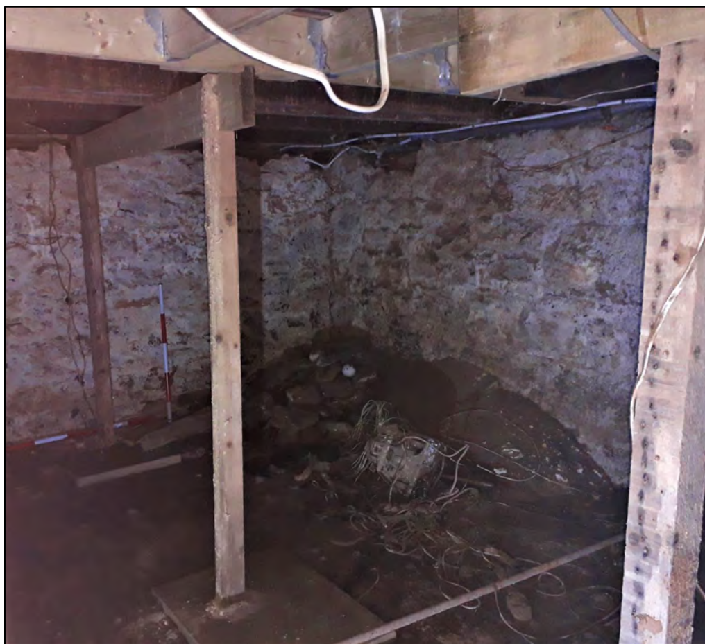
Plate 163: 2 Penrose Terrace, Room 2B1, view to the WNW. 2 x 1m scale.
