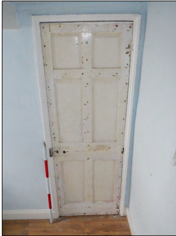
Plate 152: 2 Penrose Terrace, Room 2F5, view to the E. 1m scale.
