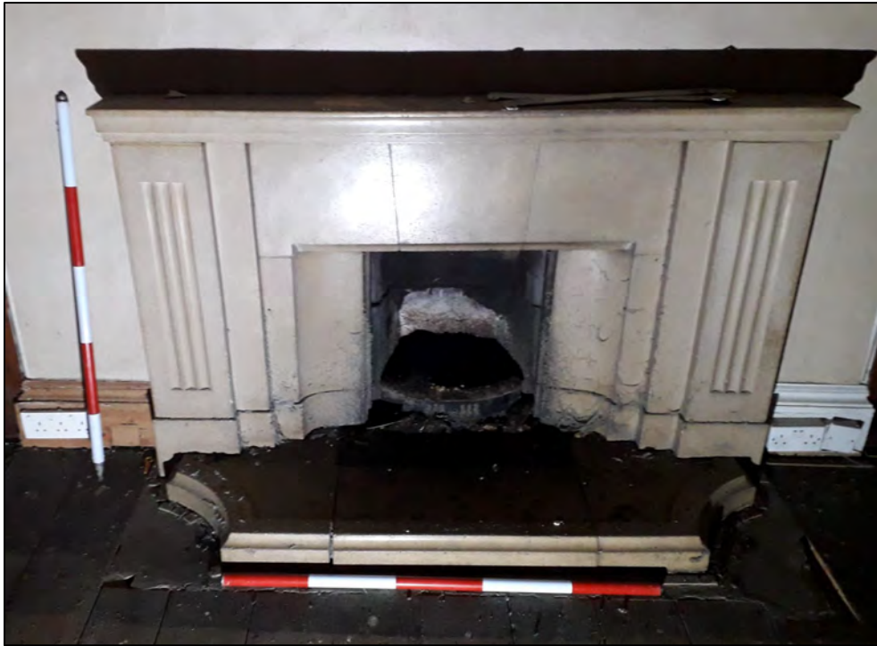
Plate 38: 1 Penrose Terrace, Room 1G2, view to the N. 2 x 1m scale.
