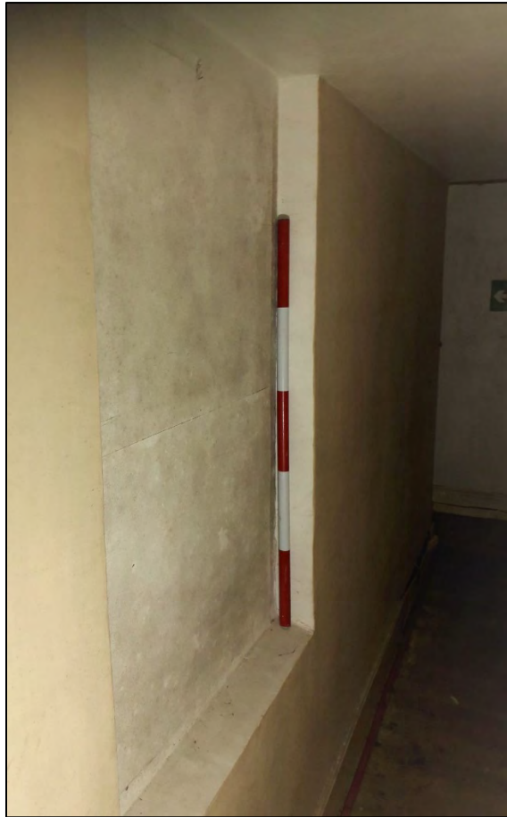
Plate 72: 1 Penrose Terrace, Room 1F10, view to the W. 1m scale.
