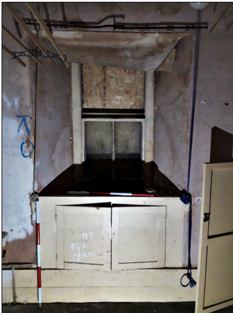
Plate 41: 1 Penrose Terrace, Room 1G4, view to the N. 2 x 1m scale.
