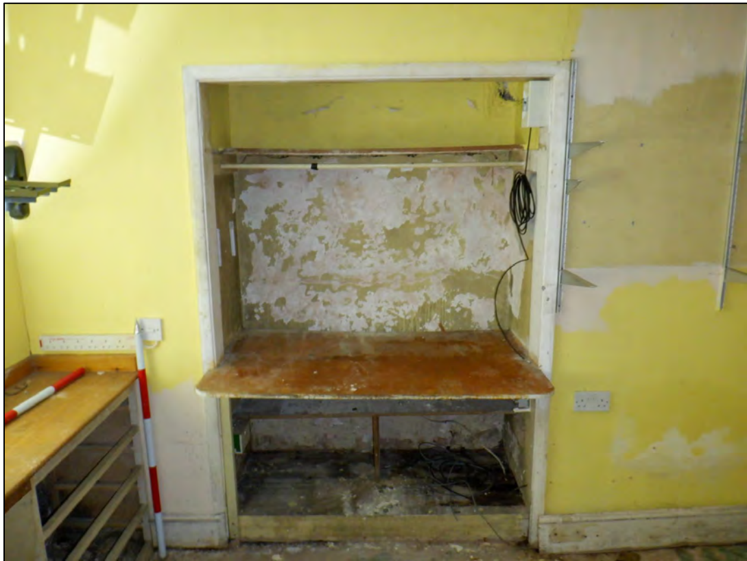
Plate 145: 2 Penrose Terrace, Room 2G8, view to the N. 2 x 1m scale.
