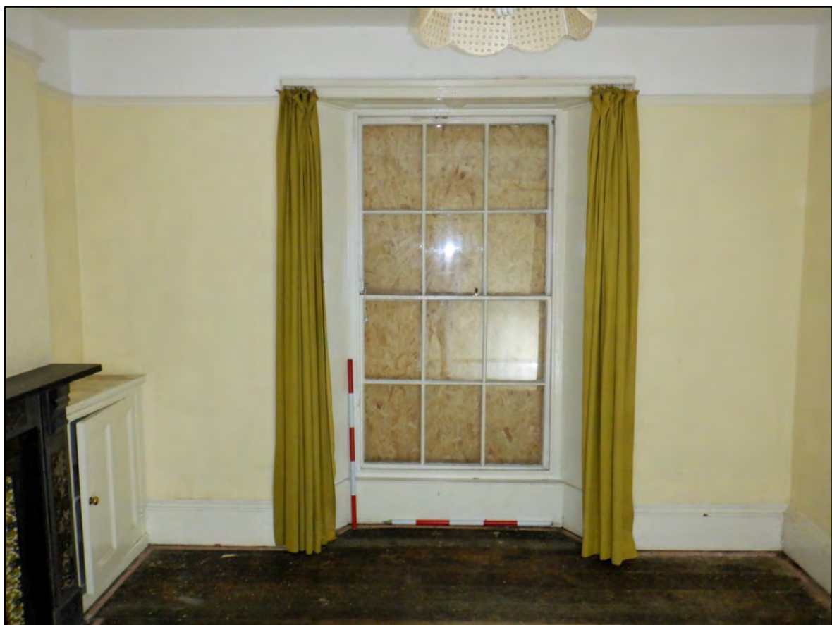
Plate 131: 2 Penrose Terrace, Room 2G2, view to the S. 2 x 1m scale.
