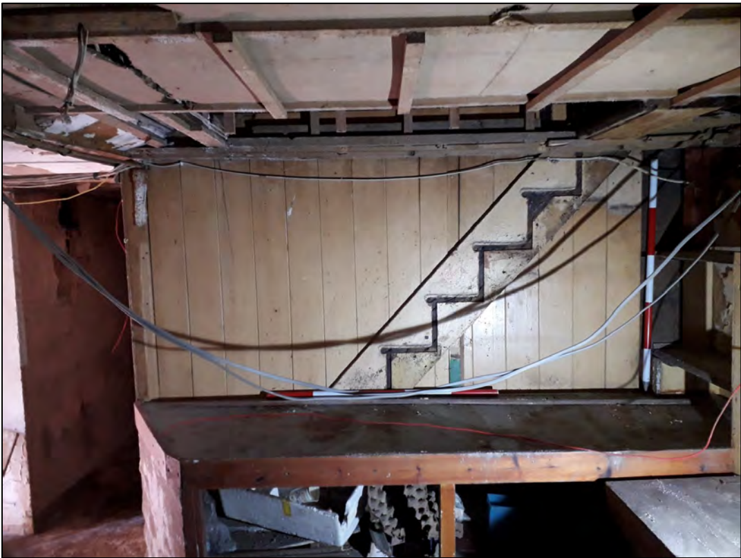
Plate 99: 1 Penrose Terrace, Room 1B7, view to the W. 2 x 1m scale.
