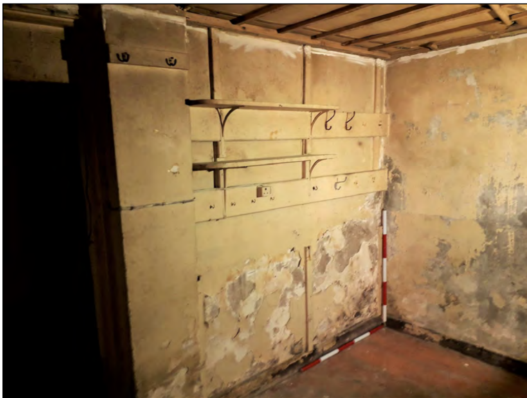
Plate 85: 1 Penrose Terrace, Room 1B3, view to the SW. 2 x 1m scale.
