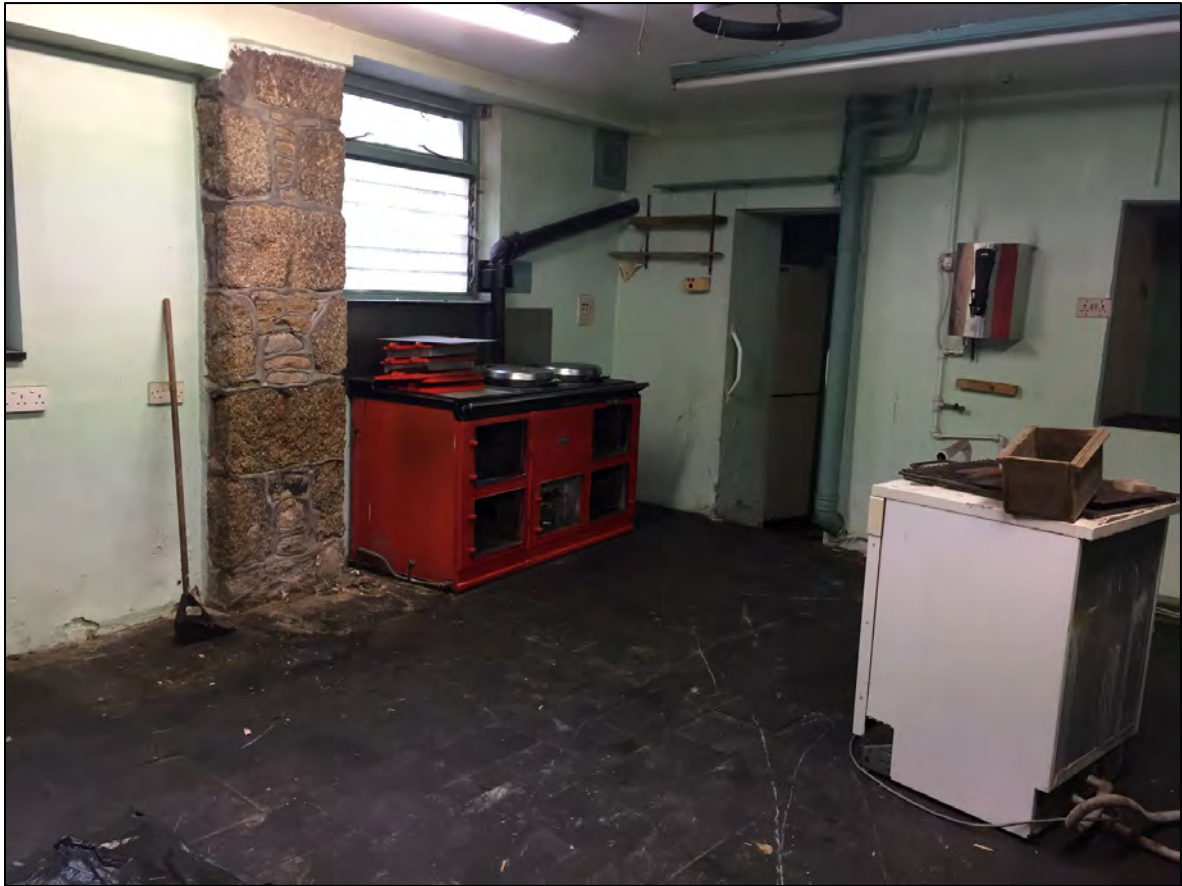
Plate 19: 1 Penrose Terrace, Room 1G12, view to the NE. Image Supplied by CAD Heritage.
