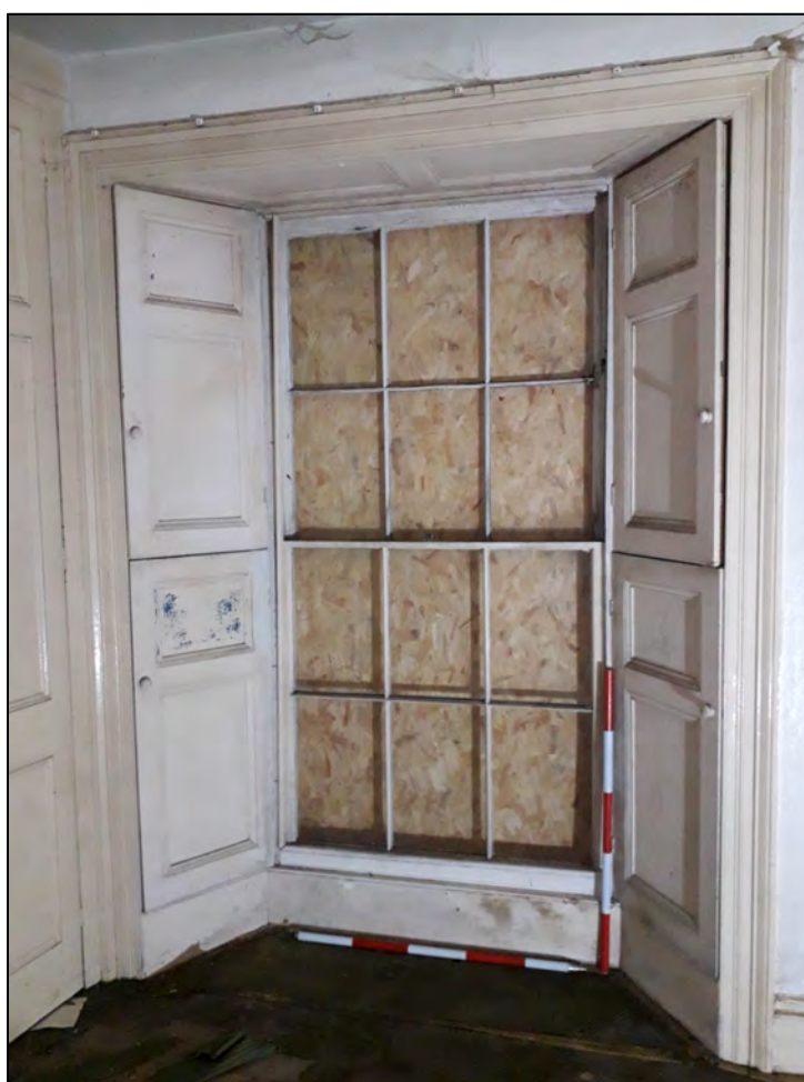
Plate 33: 1 Penrose Terrace, Room 1G5, view to the ENE. 2 x 1m scale.
