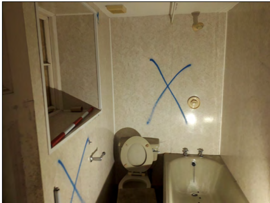
Plate 65: 1 Penrose Terrace, Room 1F11, view to the N. 1m scale.
