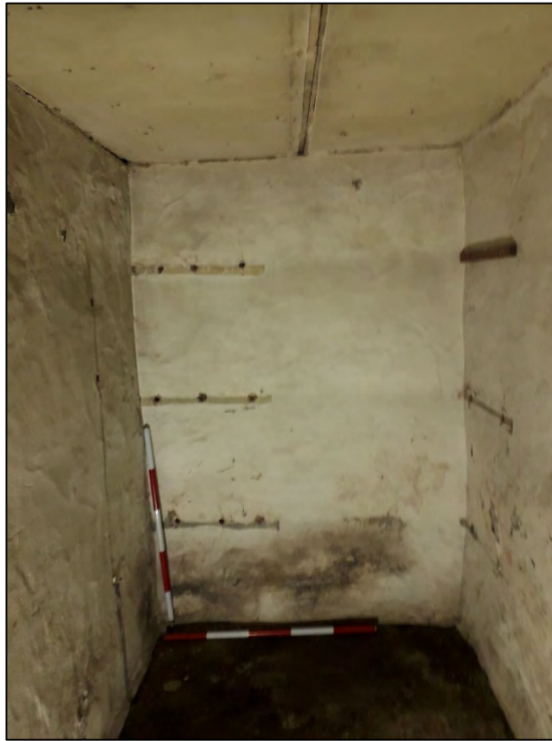
Plate 106: 1 Penrose Terrace, Room 1B1, view to the W. 2 x 1m scale.
