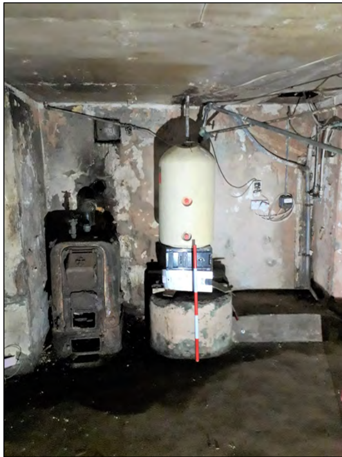
Plate 83: 1 Penrose Terrace, Room 1B3, view to the W. 1m scale.
