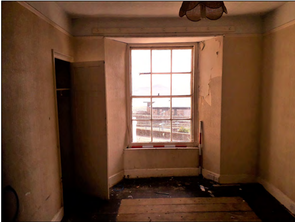
Plate 58: 1 Penrose Terrace, Room 1F8, view to the E. 2 x 1m scale.
