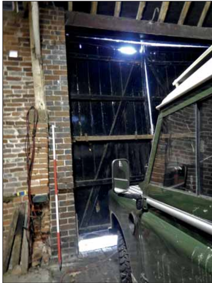
Plate 33: Main Barn, north wall, double doors, looking N. 2m scale
