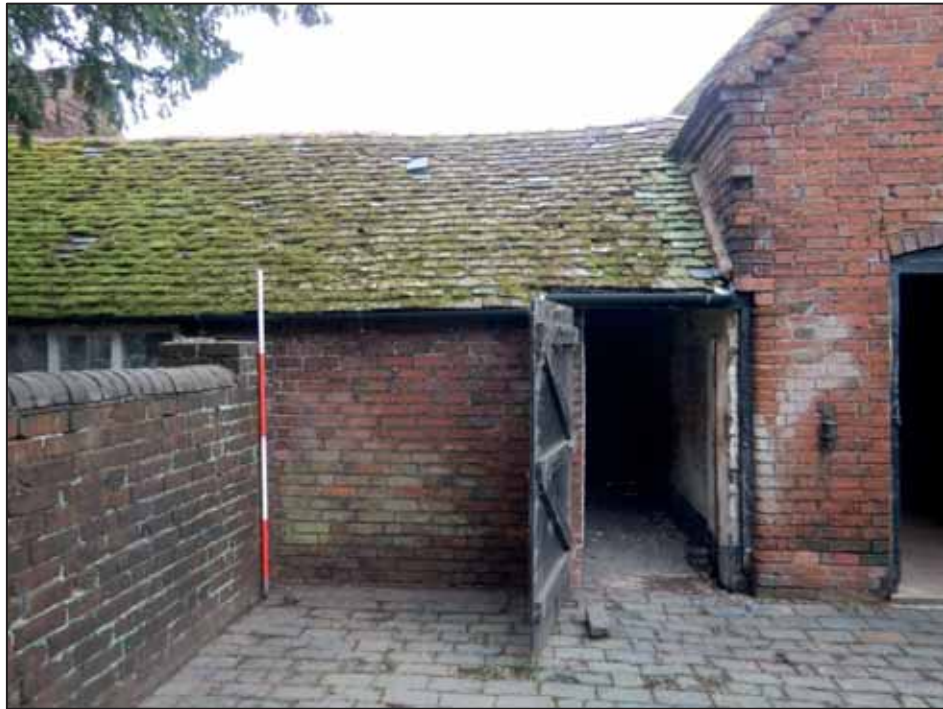
Plate 13: East Facing Elevation of the East Wing, looking W. 2m scale.
