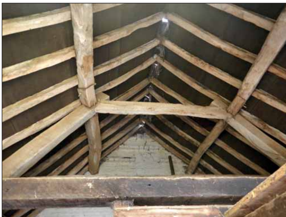
Plate 49: Dog Kennels modified roof structure, view to the W. 2m scale.
