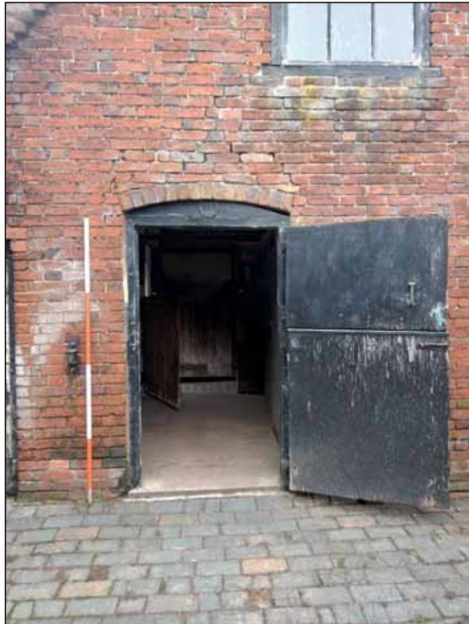
Plate 17: East Facing Elevation of the Dog Kennels, looking W. 2m scale.
