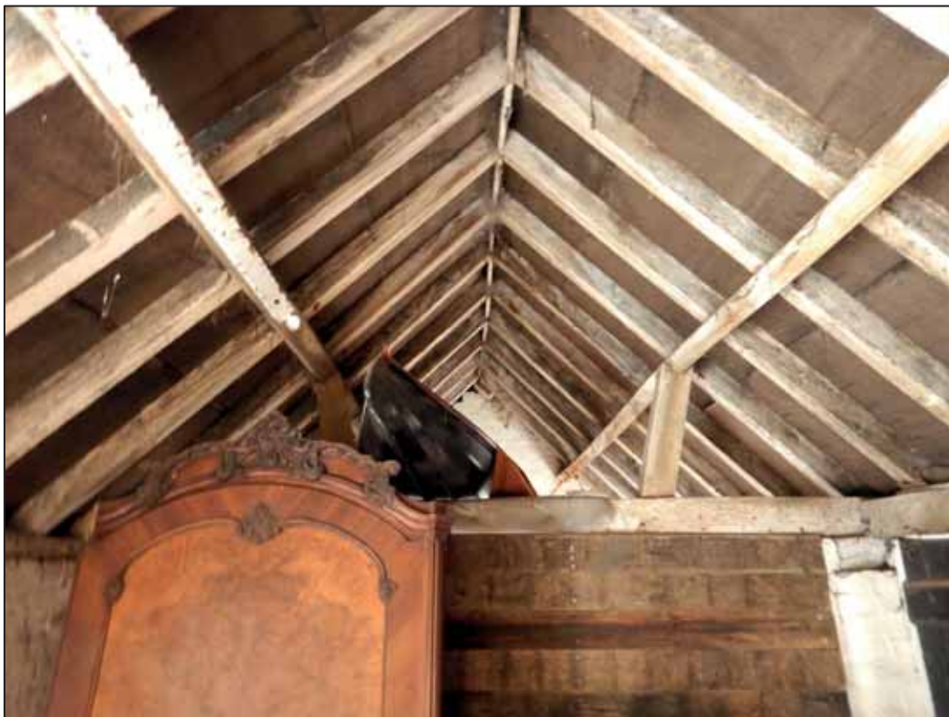
Plate 52: East Wing, North Store roof structure, view to the S.
