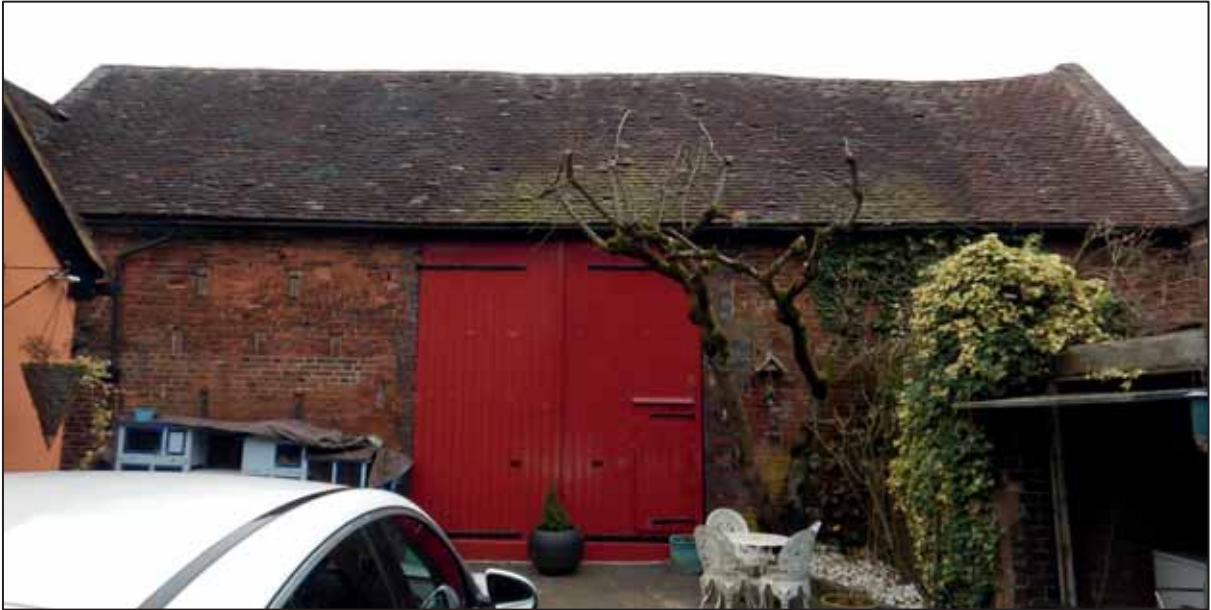
Plate 21: South Facing Elevation of the Main Barn, looking N.
