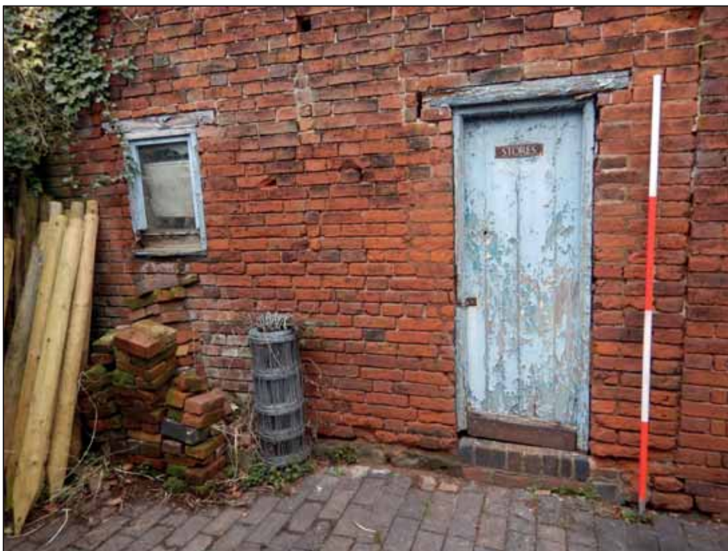
Plate 26: South Facing Elevation of the Main Barn (east end), showing partial sandstone base to wall and unkeyed junction with dog kennels. looking NNW. 2m scale.
