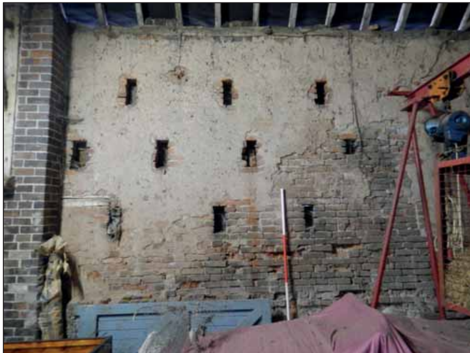
Plate 34: Main Barn, south wall (west end), looking S. 2m scale.
