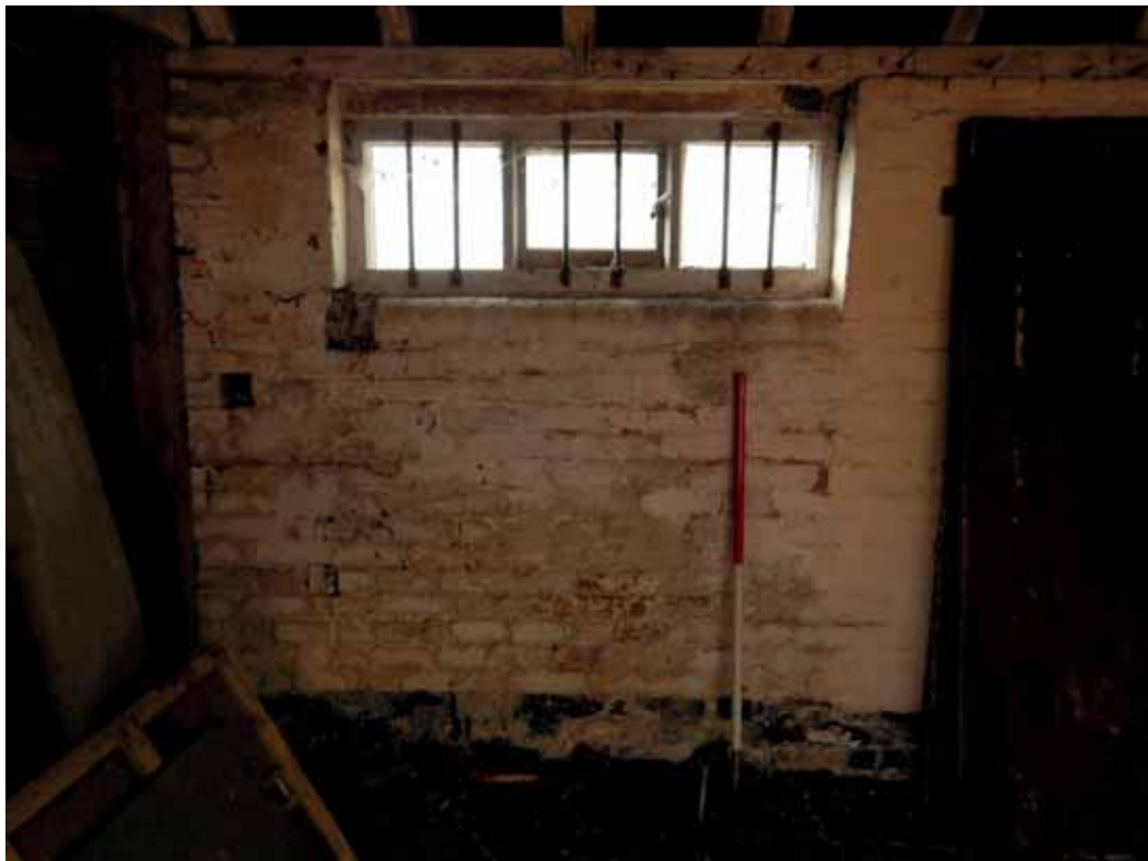
Plate 54: East Wing, South Store, view to the E. 1m scale.
