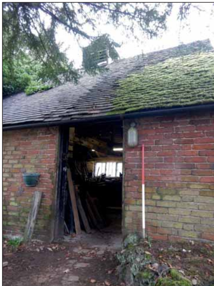
Plate 14: East Facing Elevation of the S end of the East Wing, looking SW. 1m scale.
