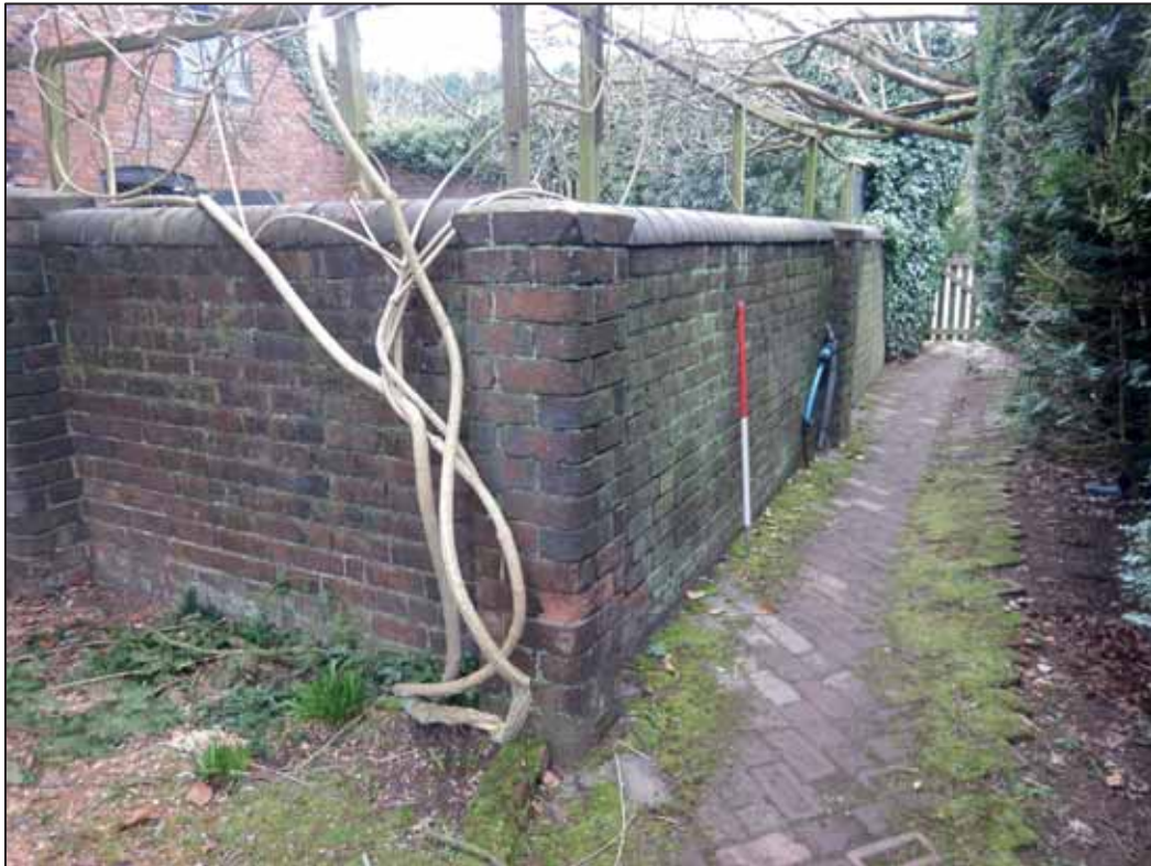
Plate 9: East facing elevation of the eastern courtyard, WNW, 1m scale.
