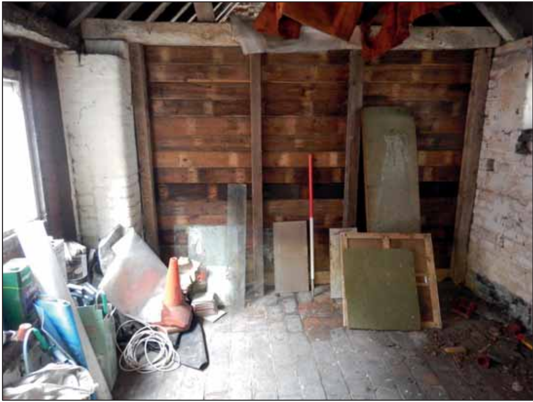
Plate 53: East Wing, South Store, view to the N. 1m scale.
