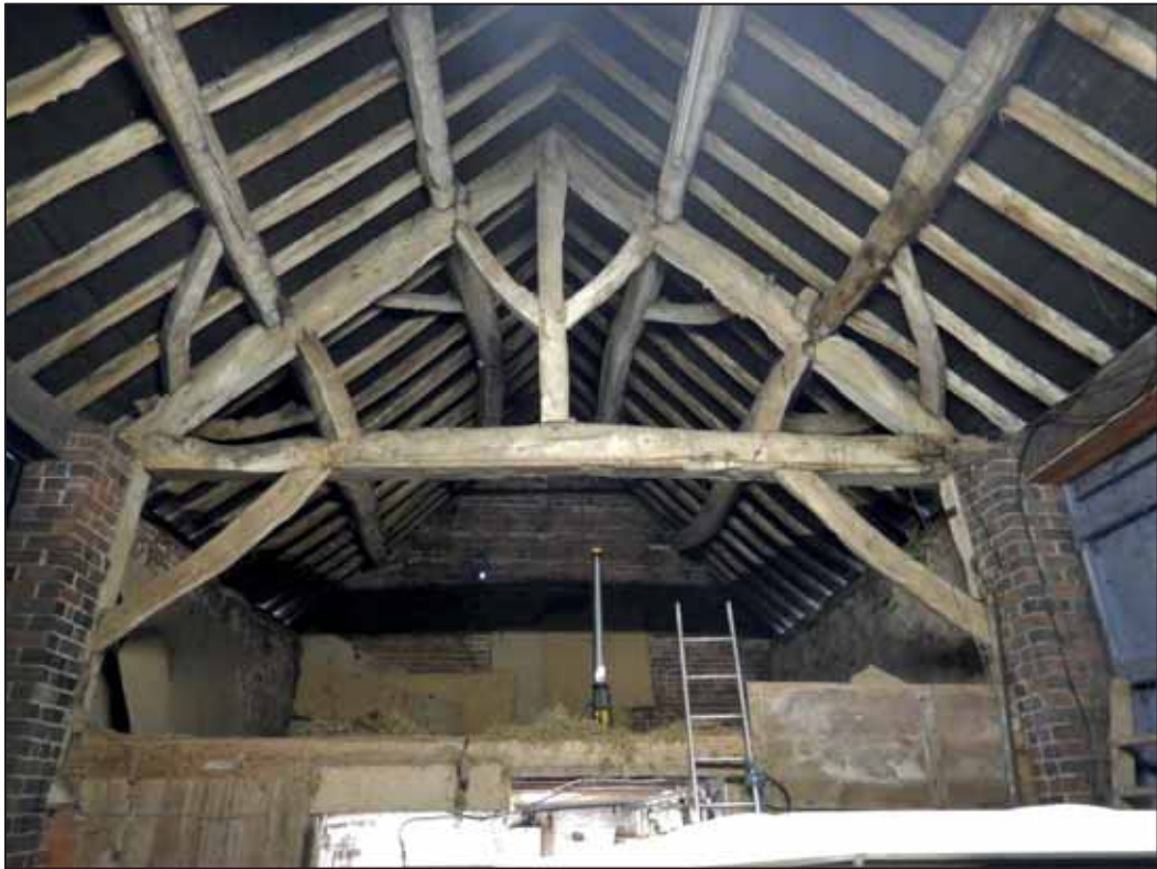
Plate 37: Main Barn, roof structure (east end), looking E.
