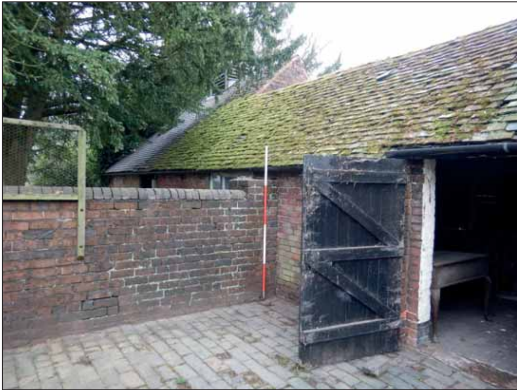
Plate 15: East Facing Elevation of the East Wing, looking SW. 2m scale.
