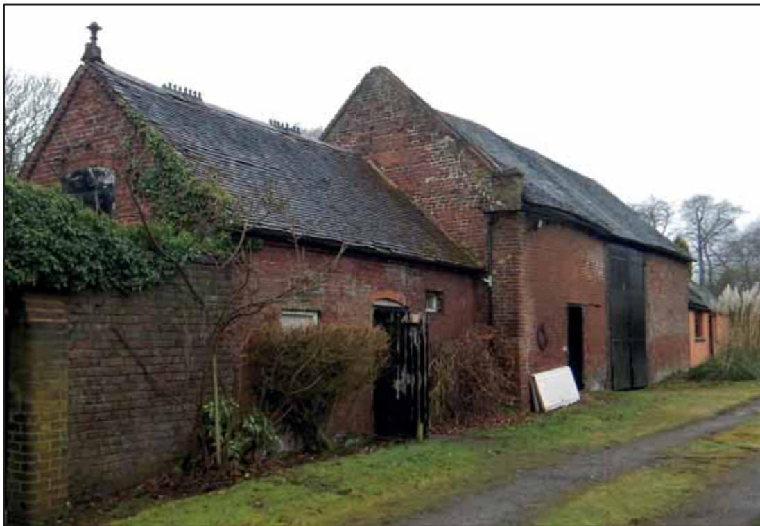
Plate 18: East facing elevation of the main barn (north side) looking ESE.
