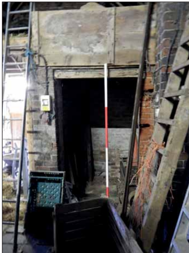
Plate 38: Main Barn, opening to small store looking E. 2m scale.
