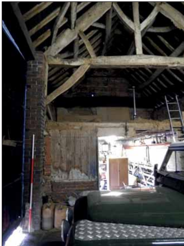
Plate 36: Main Barn, east partition wall looking E. 2m scale.
