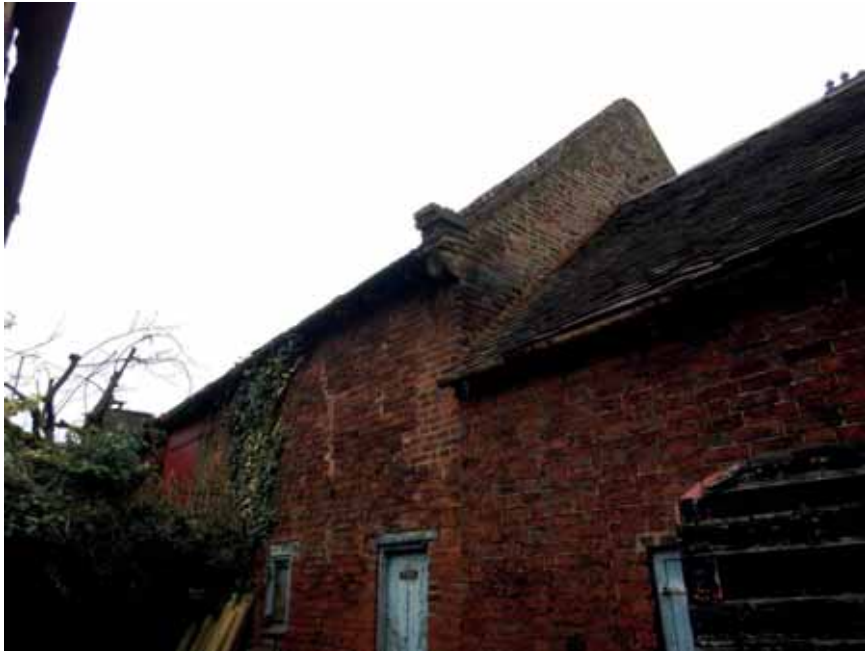
Plate 11: East facing elevation of the main barn (south side) showing sandstone corbel springer to verge parapet, looking NW.
