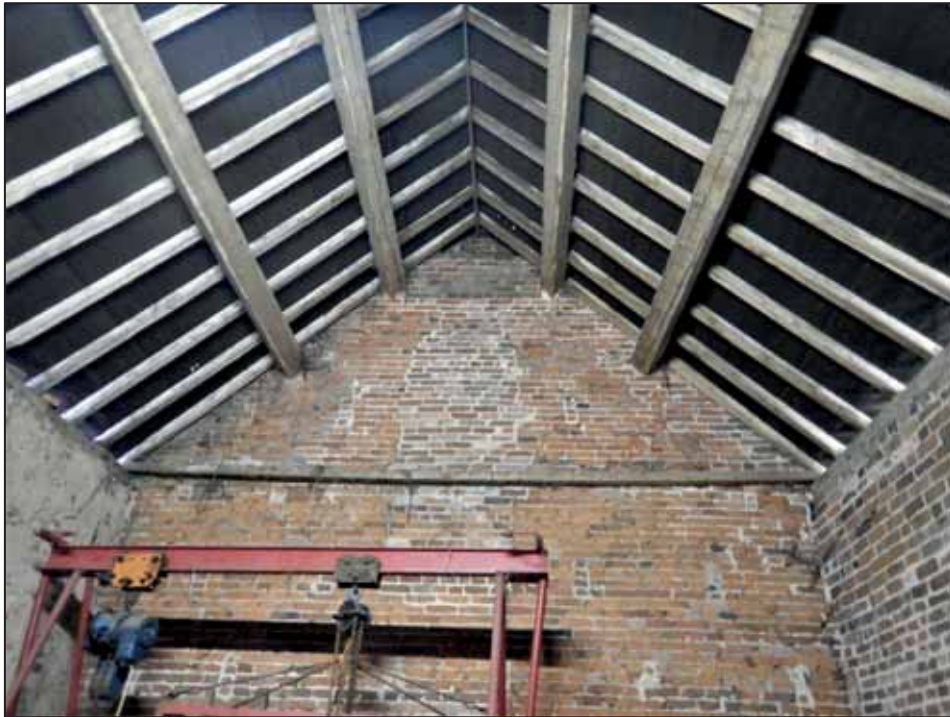
Plate 31: Main Barn, west wall, looking W.
