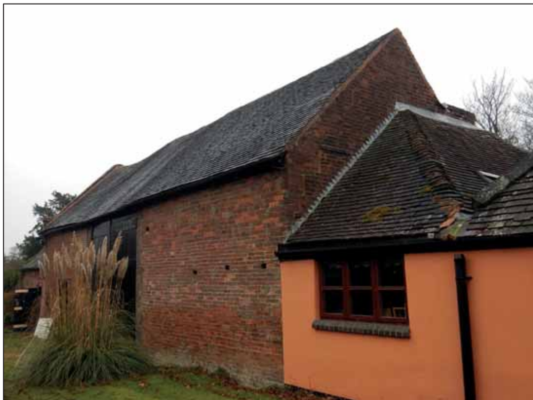
Plate 27: West facing elevation of the main barn, view to the SE.
