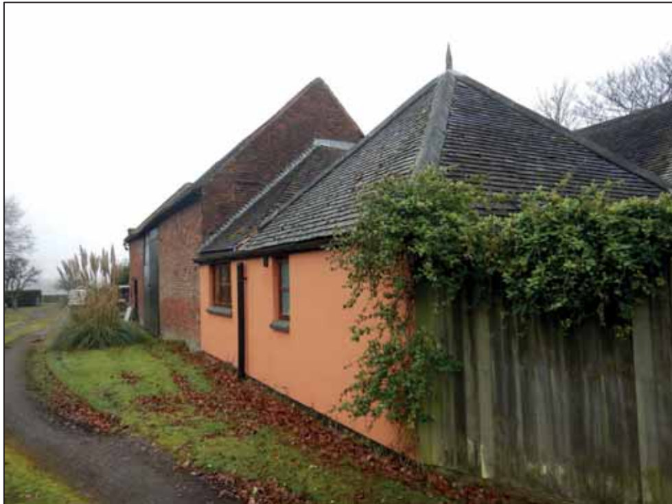
Plate 8: North Facing Elevation of Moat Bank Cottage, looking ESE.
