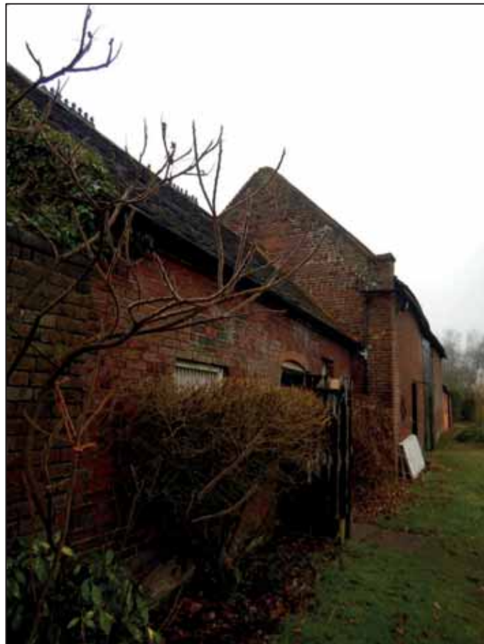
Plate 12: East facing elevation of the main barn (north side) looking ESE.
