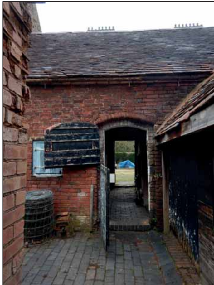
Plate 20: South Facing Elevation of the Dog Kennels, Looking N.
