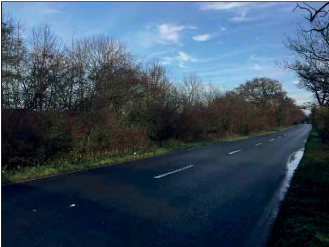
Plate 34: View of southern site boundary along the A12, looking NE.
