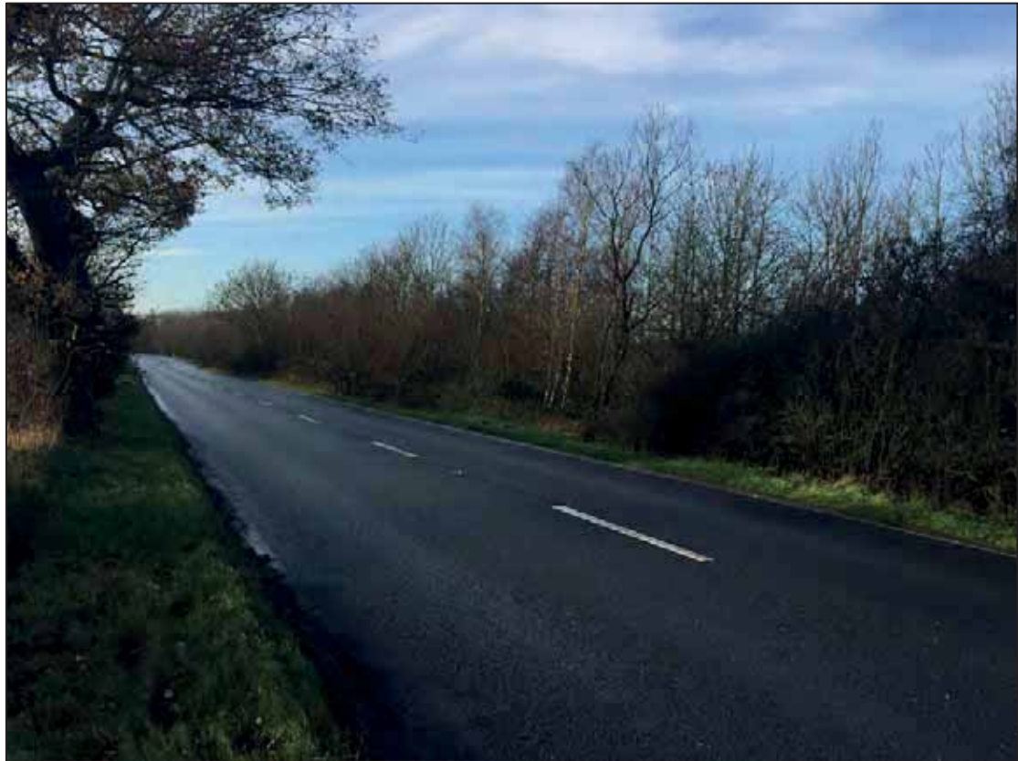
Plate 35: View of southern site boundary along the A12, looking SW.
