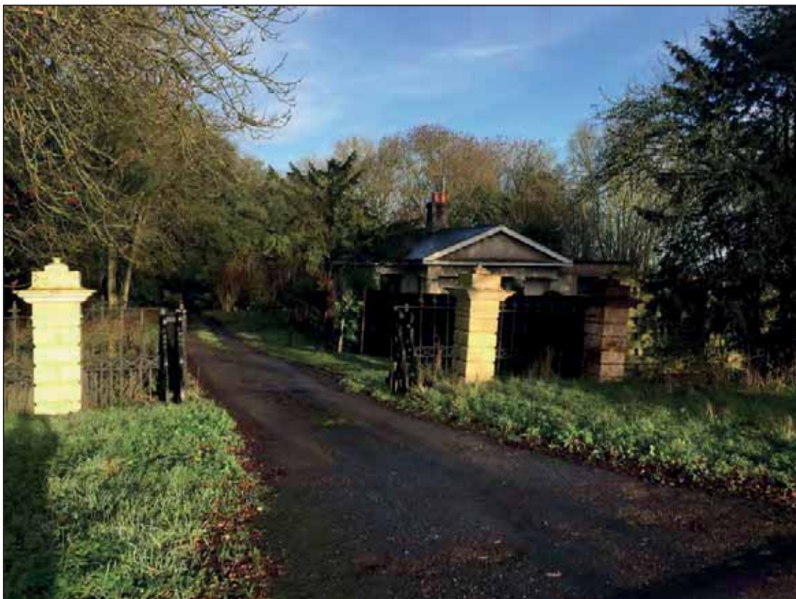
Plate 36: The Lodge and Gateway 10 Metres South of The Lodge, Looking N.
