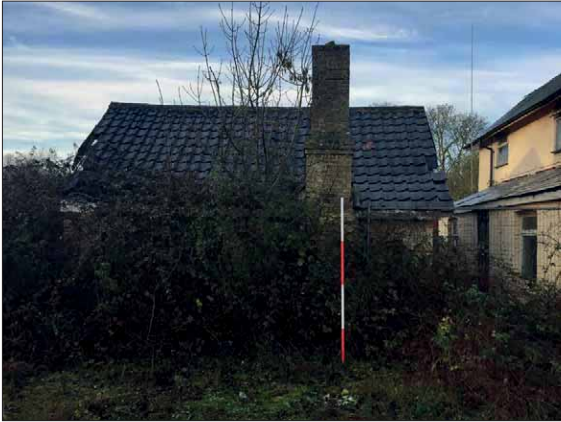
Plate 29: The former Park Farmhouse, outbuilding, looking W. 2m scale.
