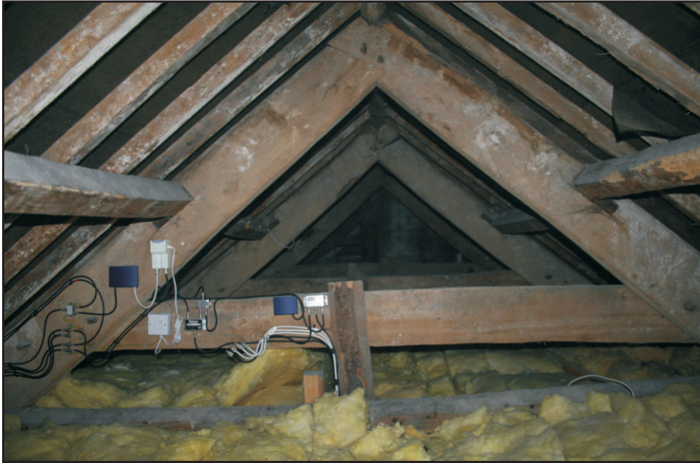
Fig. 22 The roof above the central chamber.
