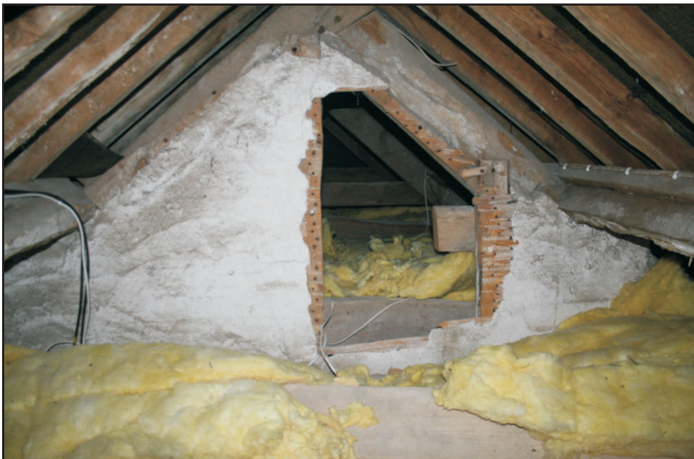
Fig. 23 Roof truss III with partition rising to the apex.
