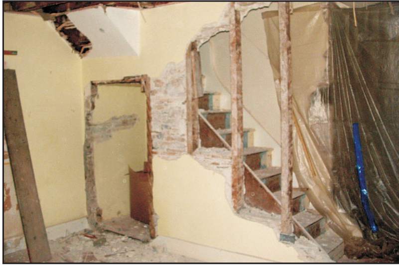
Fig. 15 Hall, stairs and primary stair cupboard, viewed from the SE.
