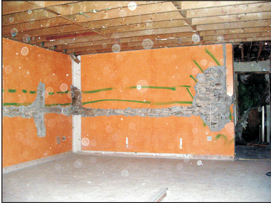
Fig. 11 Interior of the W room after stripping.
