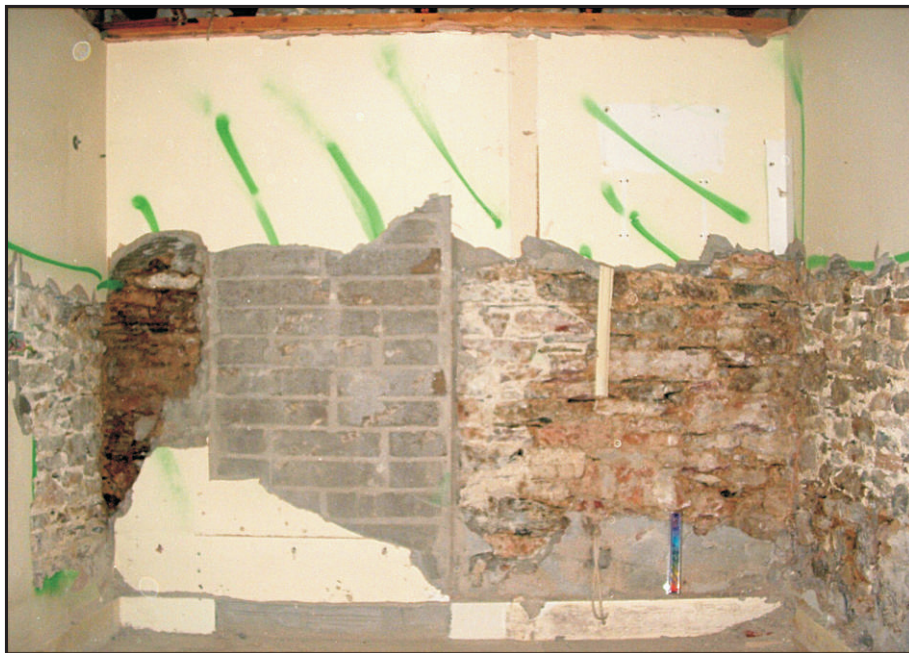
Fig. 12 The entry after stripping, showing blocked doorway in N wall.
