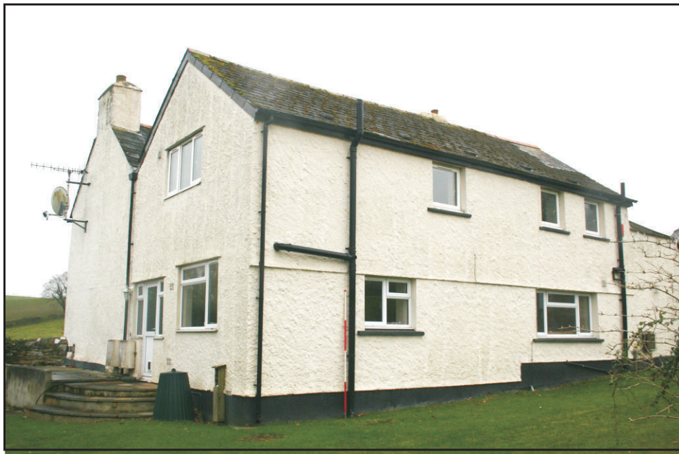
Fig. 10 Exterior from NE with N range in foreground.
