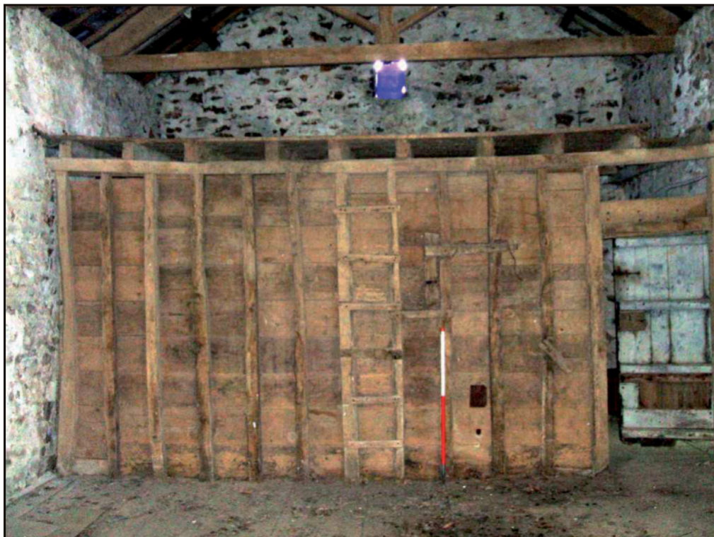
Photo. 4 First floor showing partition, looking west. 1m scale.
