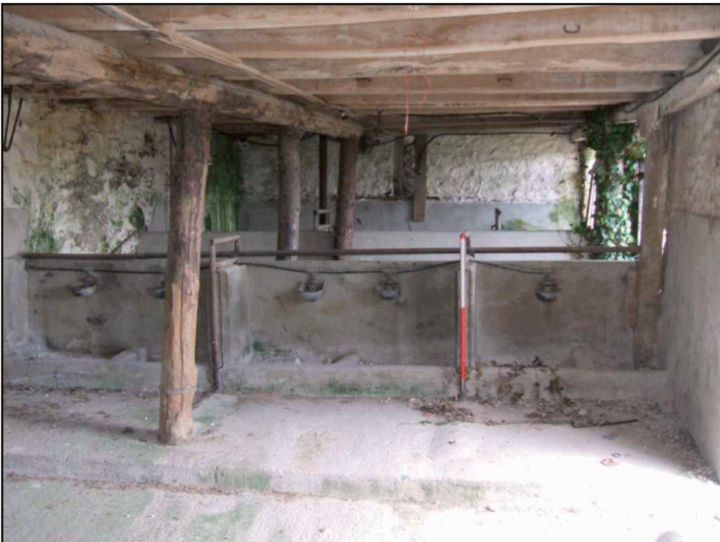
Photo. 2 Ground floor showing the west stalls, looking east. 1m scale.
