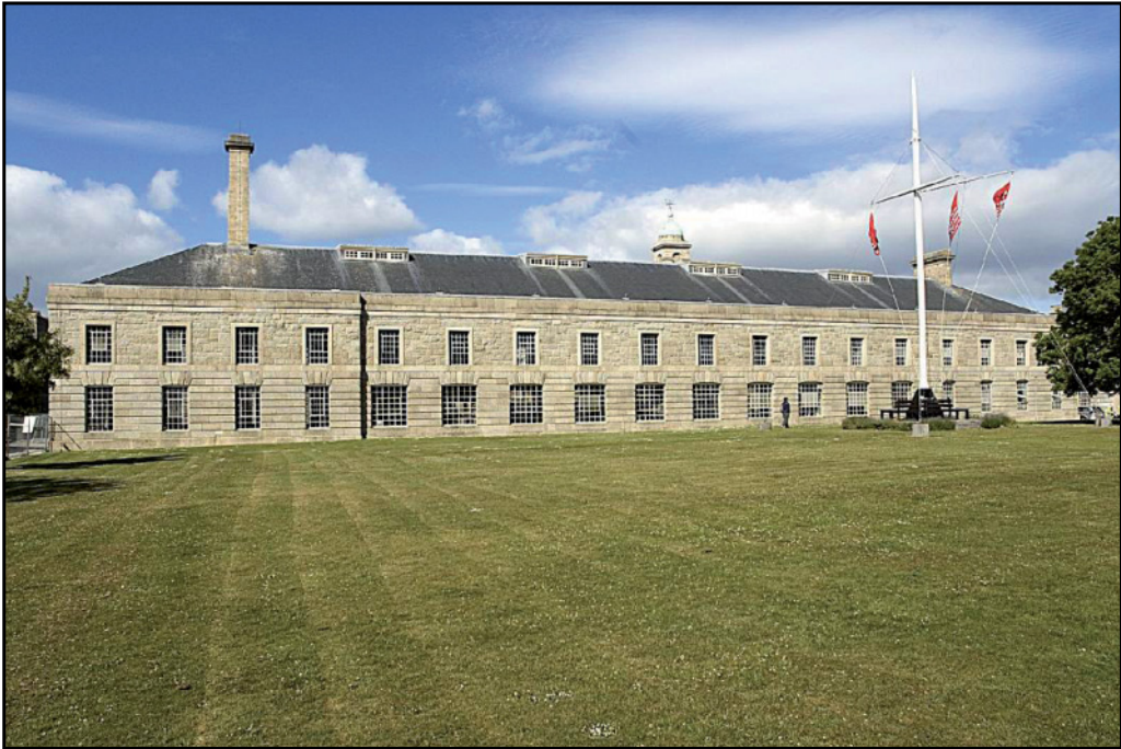
Photo. 1 East exterior elevation, looking west.
