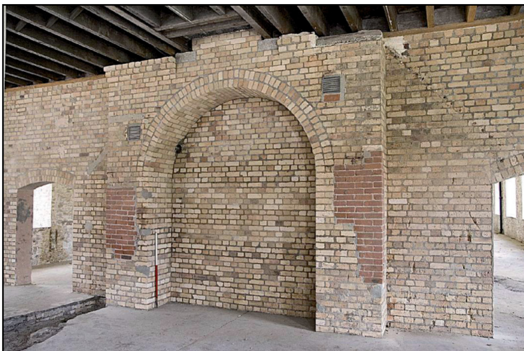
Photo. 6 Room G8, north partition wall showing arches, looking north-west. 1m scale.
