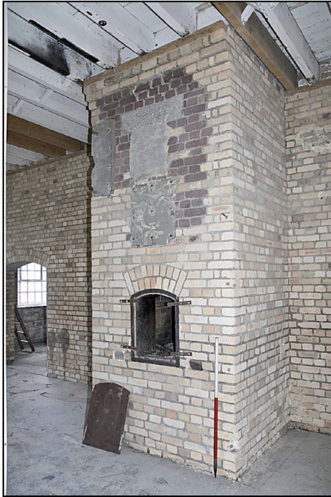
Photo. 5 Room G7, view of chimney with firebox, looking south-east. 1m scale.
