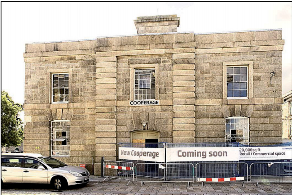
Photo. 2 North exterior elevation, looking south. 1m scale.
