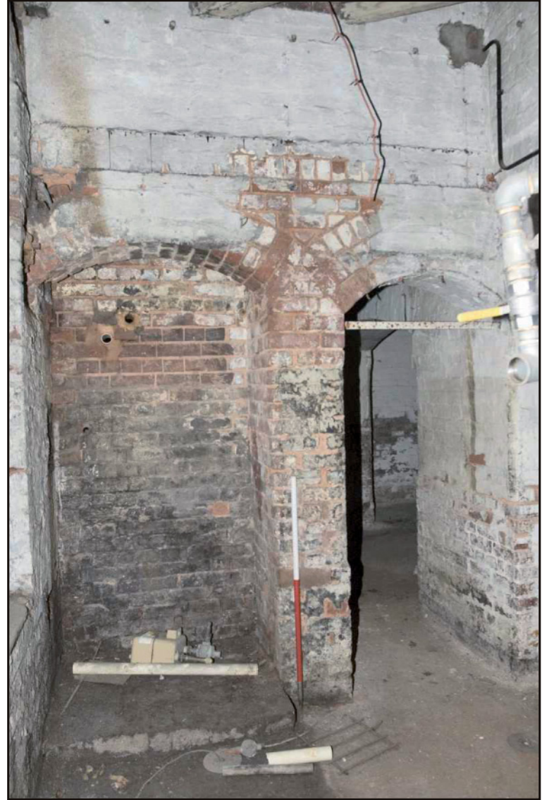
Photo. 6 The basement, showing coal cellar, looking south east. 1m scale.
