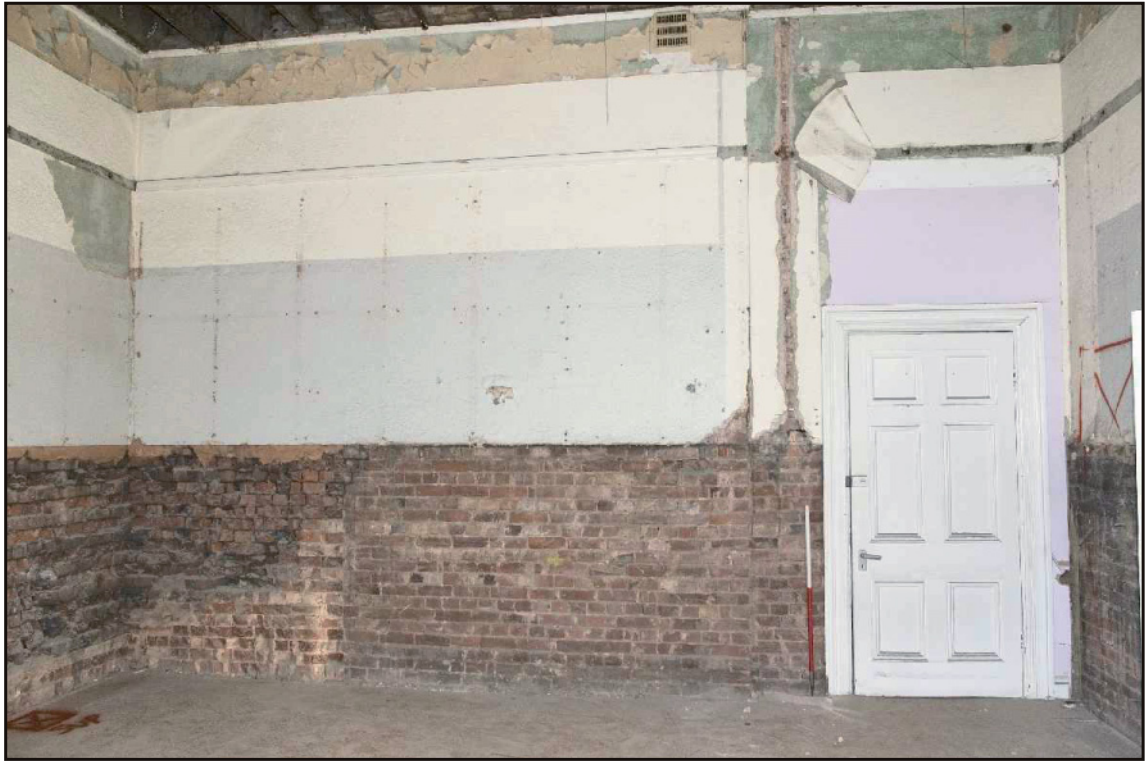
Photo. 3 A ground floor classroom, showing altered fireplaces, looking west. 1m scale.
