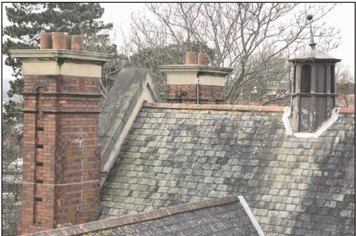
Photo. 8 Chimney stacks of 1908 and vent above science rooms.
