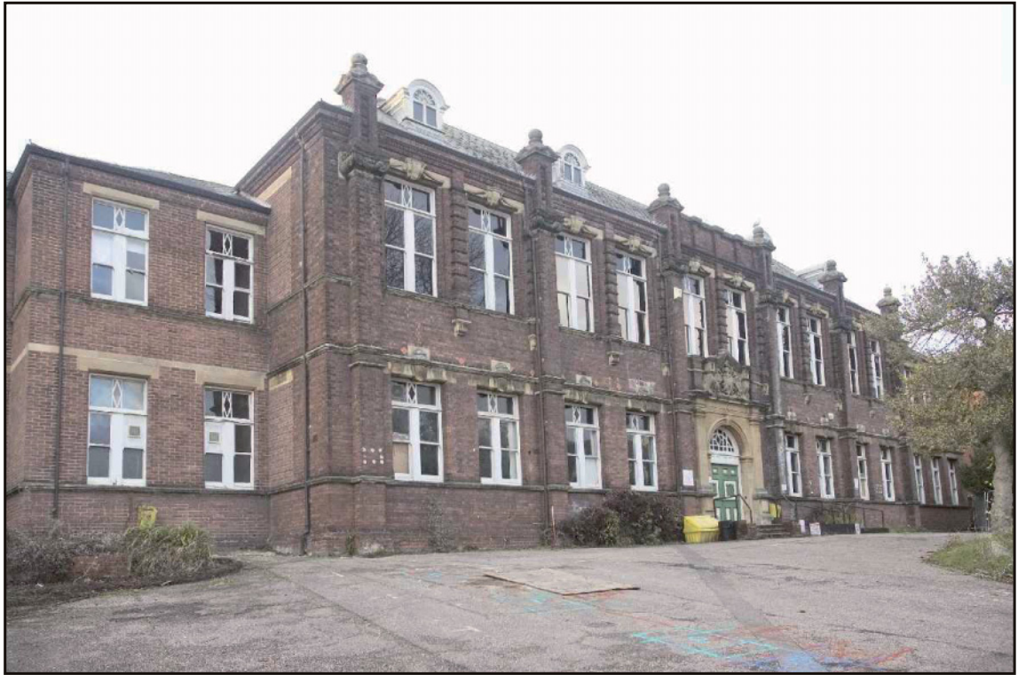
Photo. 1 The north east and south east wings, fronting Pennsylvania Road, looking north west. 1m scale.
