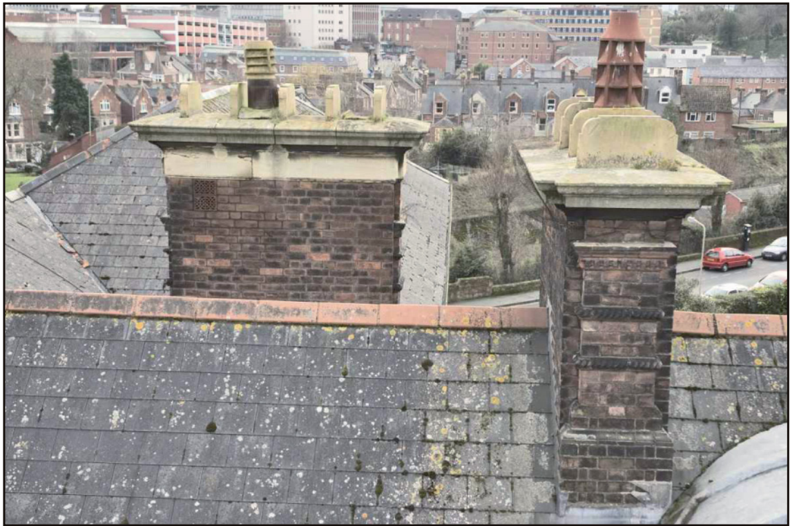
Photo. 7 Original chimney stacks, looking south.
