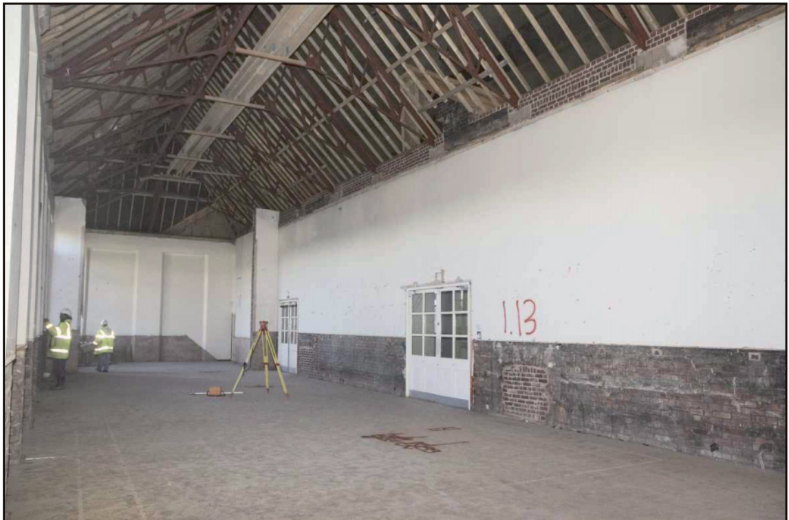
Photo. 4 The first floor hall, looking southwest. 1m scale.
