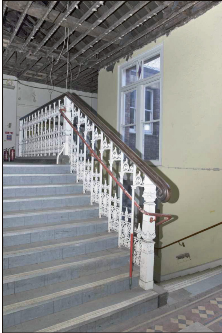
Photo. 5 The main staircase, looking south east. 1m scale.
