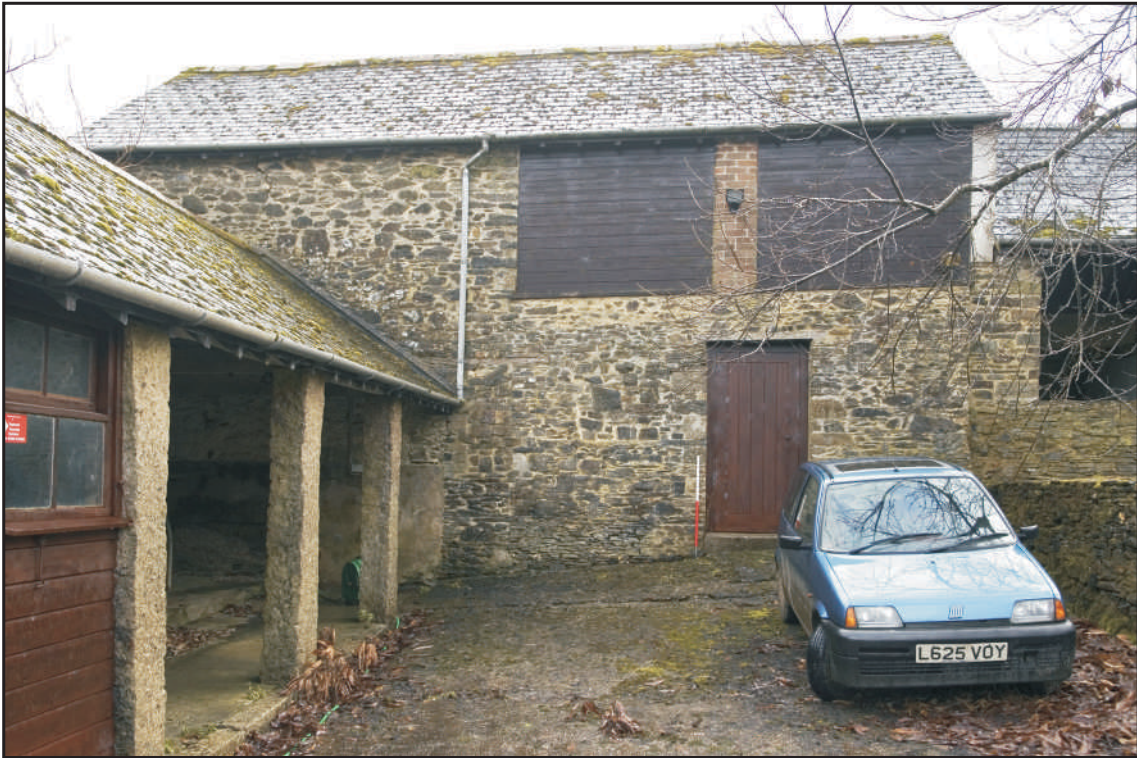
Photo 9 The stables/cow house, looking southeast. 1m scale.
