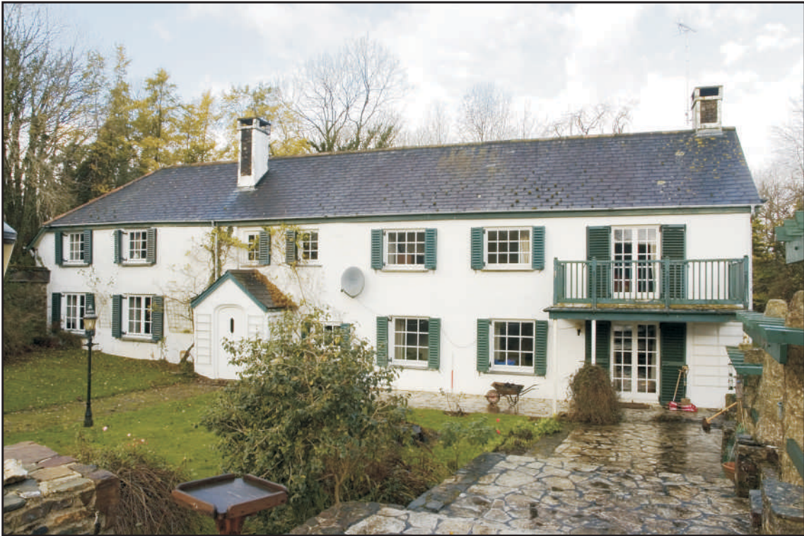
Photo 1 The farmhouse, looking west. 1m scale.
