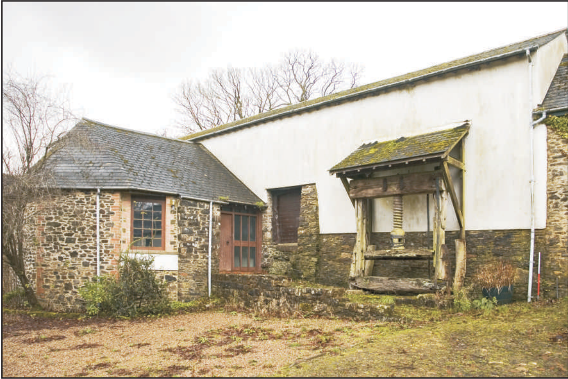
Photo 3 The threshing barn and engine house, looking south. 1m scale.
