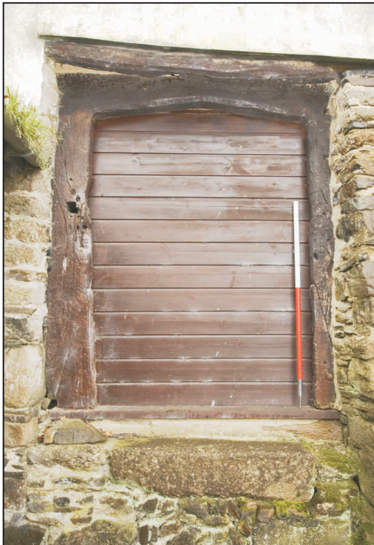
Photo 4 The reused door in the threshing barn, looking southwest. 1m scale.
