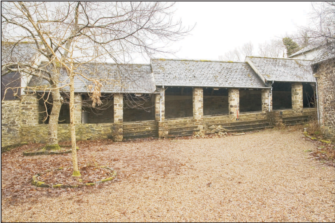
Photo 7 The southern range shippon, looking southeast. 1m scale.
