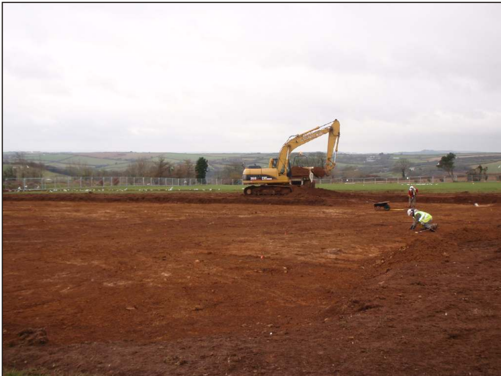
Plate 2 General view of Area 2 during stripping. Looking southwest.
