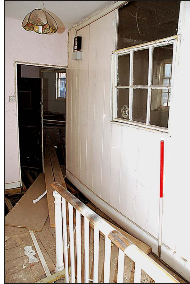
Fig. 18 View of the 19th-century corridor at third-floor level, showing the timber screen incorporating a reused sash and the handrail of the 19th-century staircase to the second floor.
