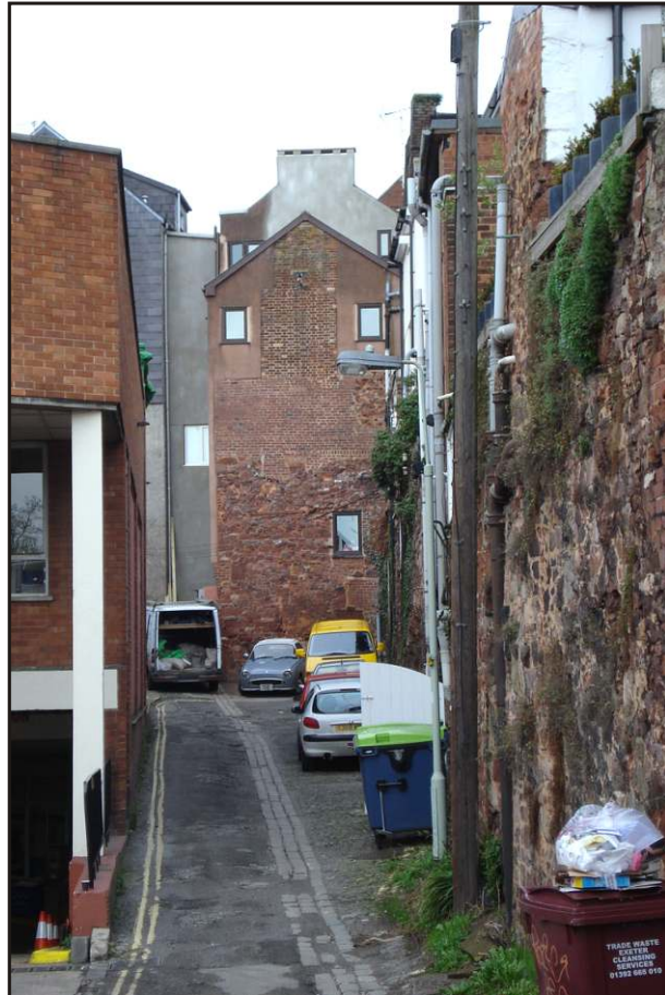
Fig. 3 View along Rackclose Lane from the site of the West Gate showing the south-eastern gable of the house (centre) standing against the city wall (right) and the narrow building (recently refaced with grey render) infilling the end of the lane alongside the original frontage.
