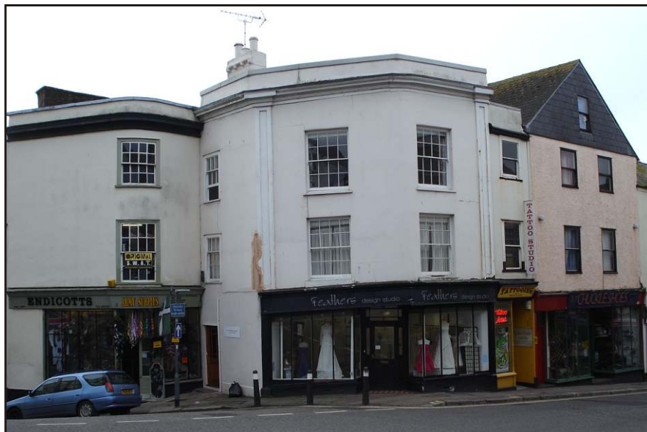
Fig. 4 The frontage of the rebuilt house towards West Street (left) and New Bridge Street (right) showing the narrow frontage of the adjoining house infilling the lane.
