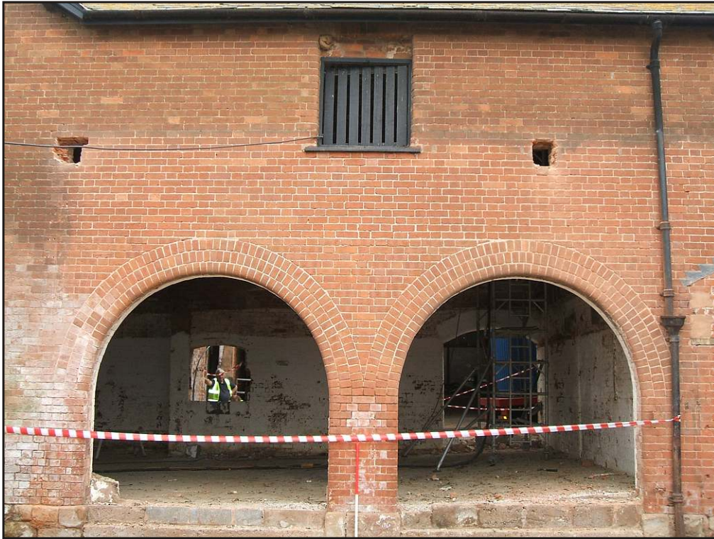
Plate 9 Barn 8, north elevation. 1m scale.
