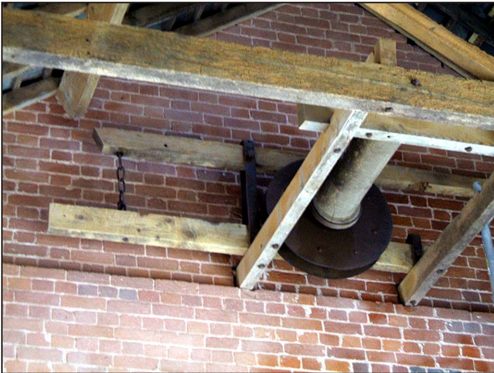
Plate 12 The hoist in barn 8. Looking northwest.
