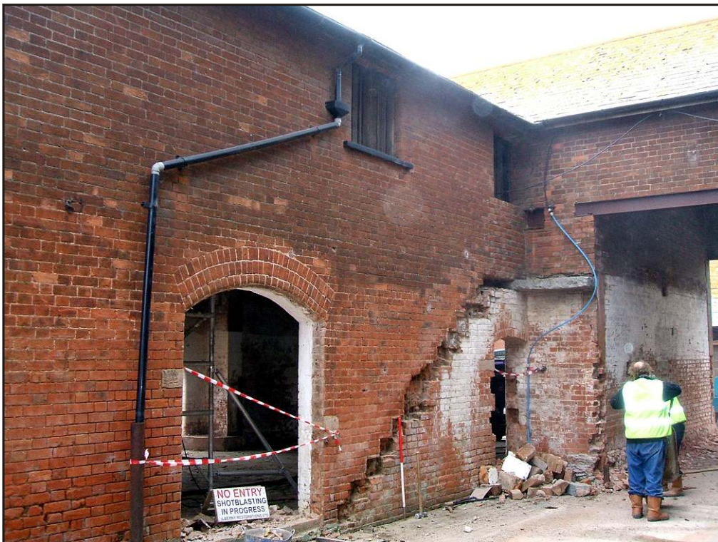
Plate 10 Barn 8, south elevation showing former steps, looking north. 1m scale.
