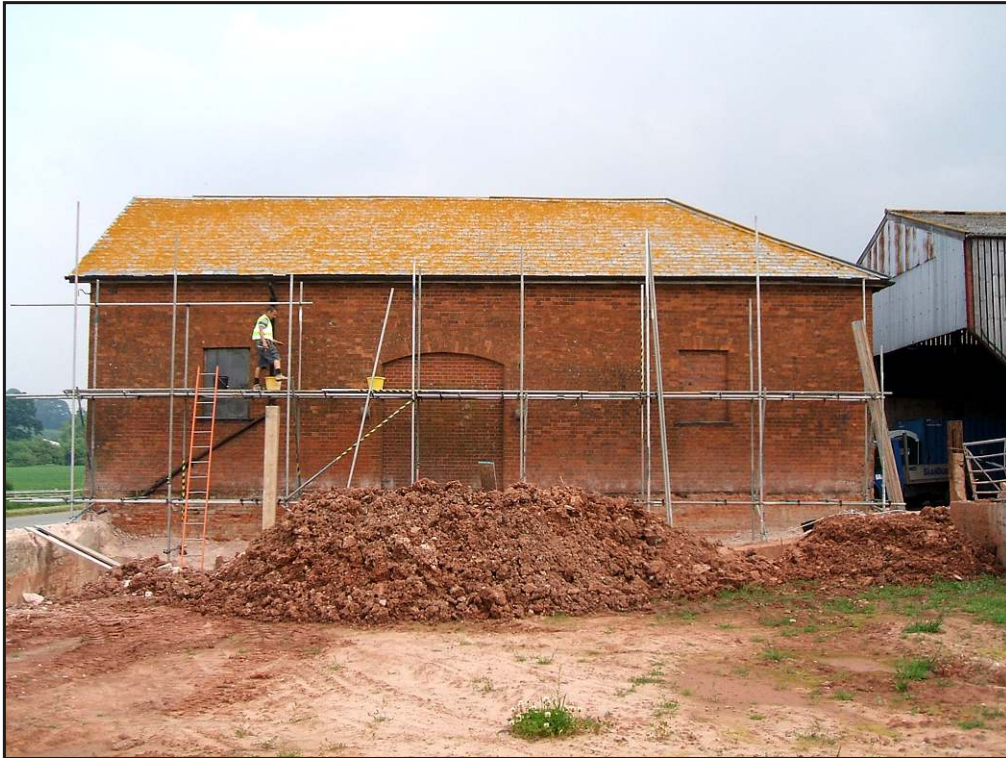
Plate 7 Barn 7, south elevation, looking northeast.
