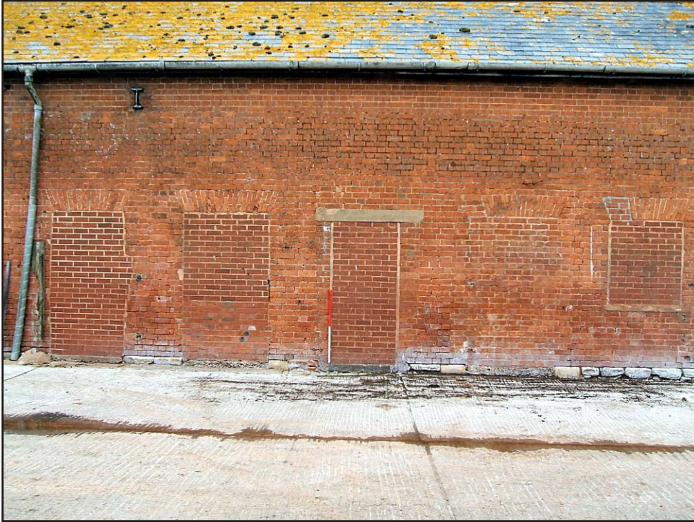
Plate 5 Barn 2, south elevation showing blocked openings, looking northwest. 1m scale.
