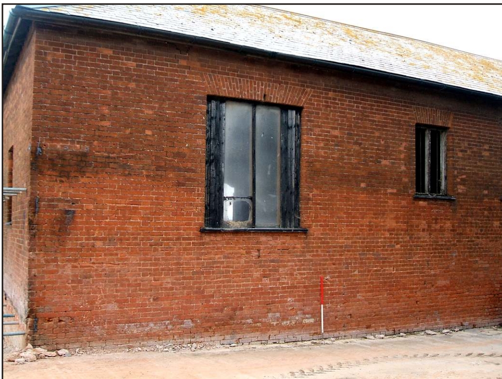
Plate 8 Barn 7, south elevation, looking north.
