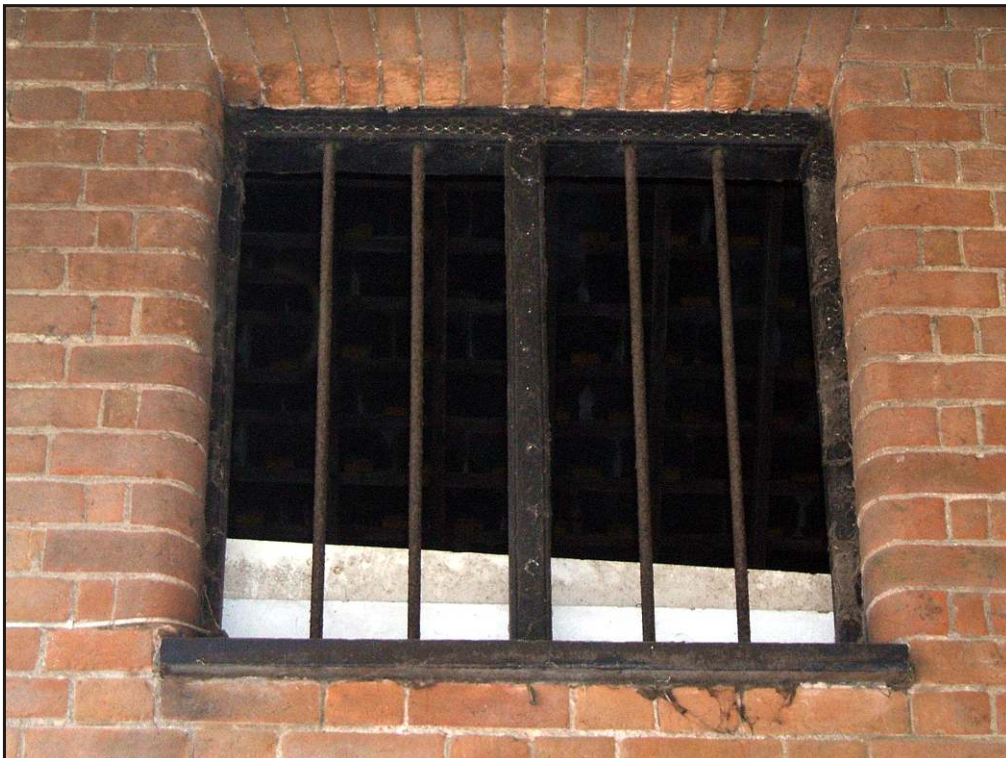
Plate 6 Barn 4, close-up view of first floor window, looking southwest.
