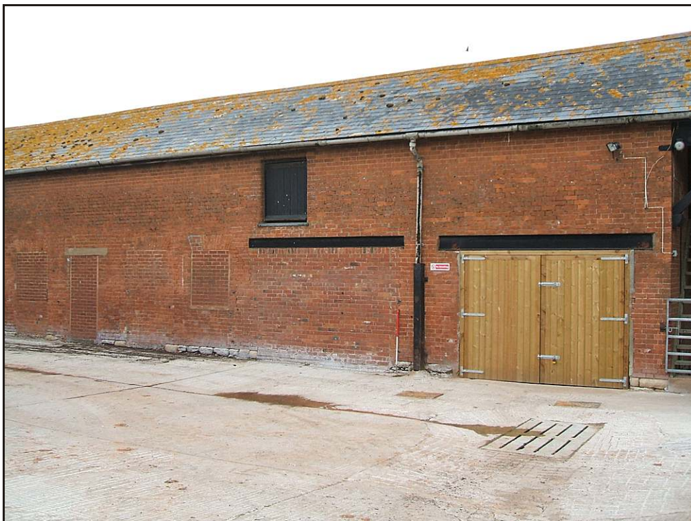
Plate 4 Barn 2, south elevation showing blocked openings, looking west. 1m scale.
