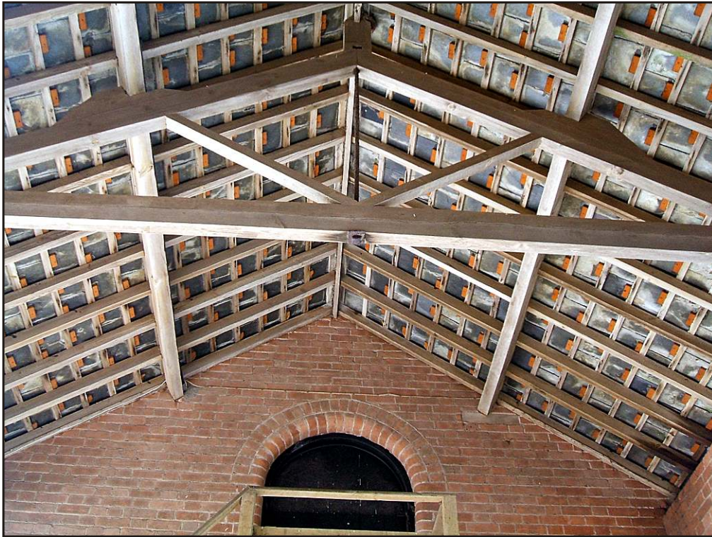
Plate 3 The roof over the entrance of barn 2. Looking southwest.
