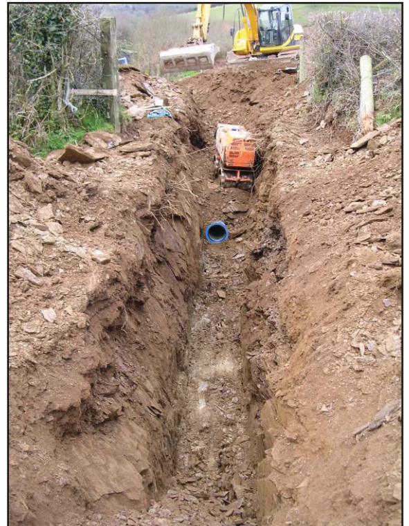
Plate 4 General view of pipeline in Field 8. Looking east.
