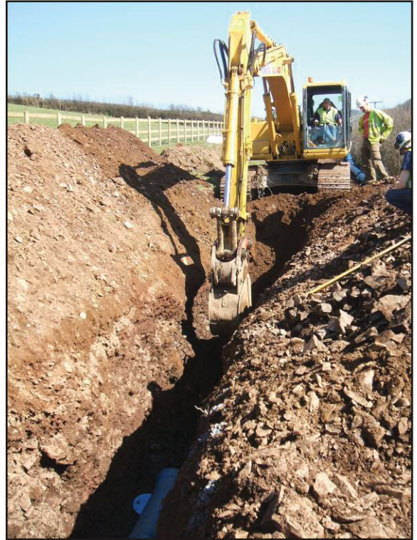
Plate 2 General view of pipeline in Field 7. Looking east.
