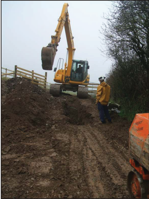
Plate 1 General view of pipeline in Field 6. Looking east.
