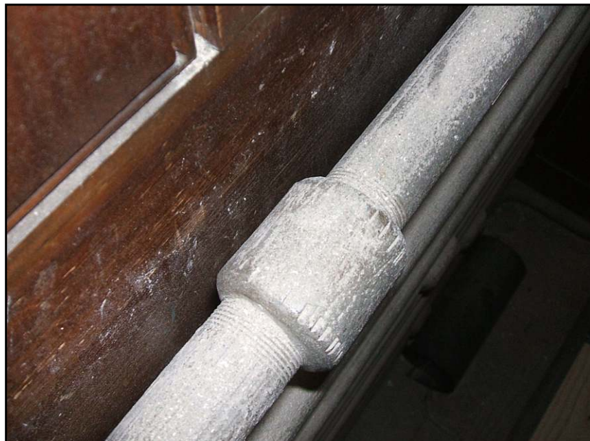
Plate 2 The coil heater in the tower: close-up view of a pipe joint socket, looking north-east.
