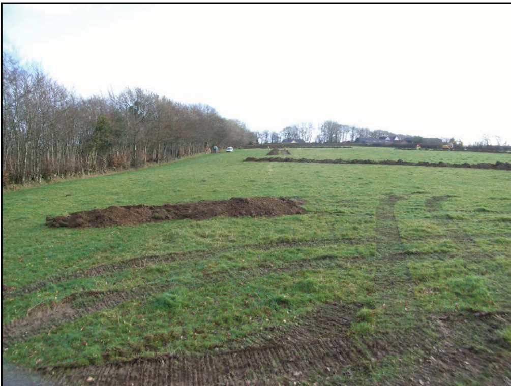
Plate 4 General view of site showing trenches 9 (foreground) and 8 (centre). Looking east.
