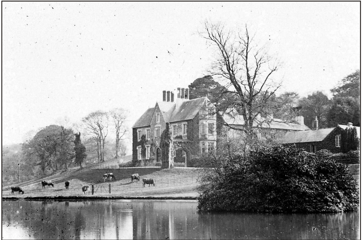
Fig. 17 View of the house c.1900 showing the service buildings and the north-west range prior to 20th-century alterations (Westcountry Studies Library framed picture collection, source unknown).
