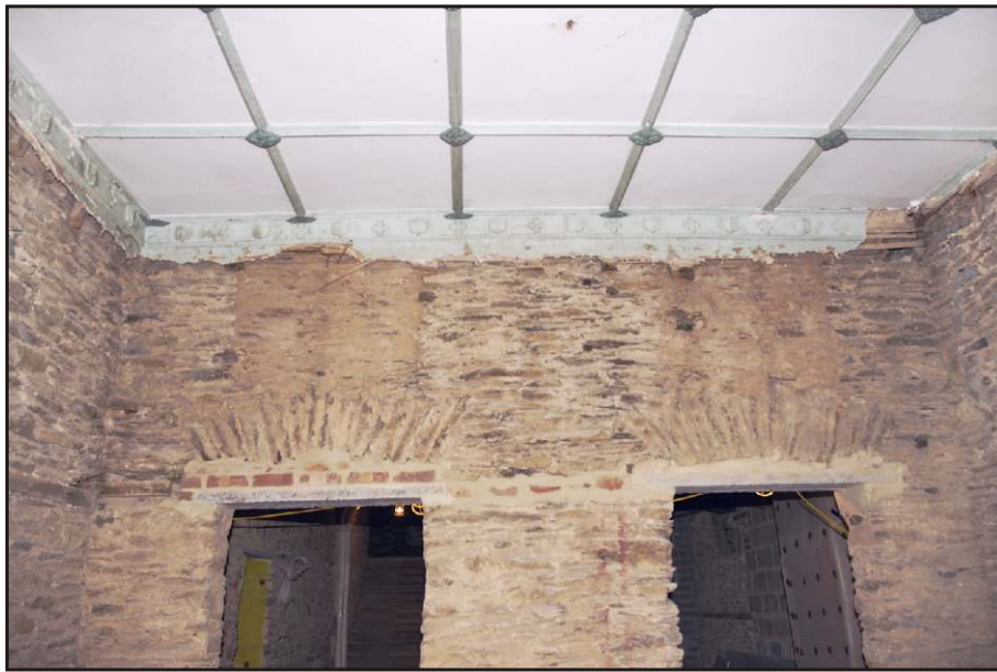
Fig. 19 View within the entrance hall, looking west, showing the paired entrances with their blocked openings over.
