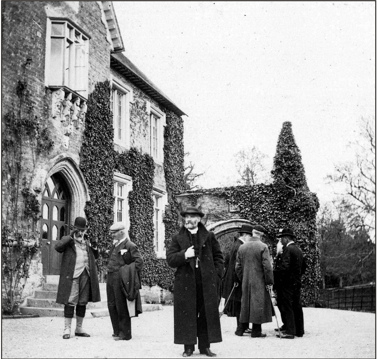
Fig. 10 Photograph of c. 1900 showing the original doors and fanlight in situ, the original form of the windows and the absence of the string course over the doorway (Westcountry Studies Library).
