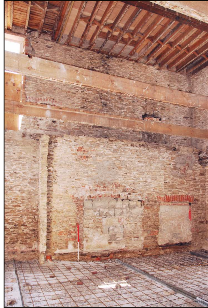
Fig. 26 Blocked fireplaces in the west wall of the new kitchen and in the rooms above, showing the character of the mid 19th-century fabric.
