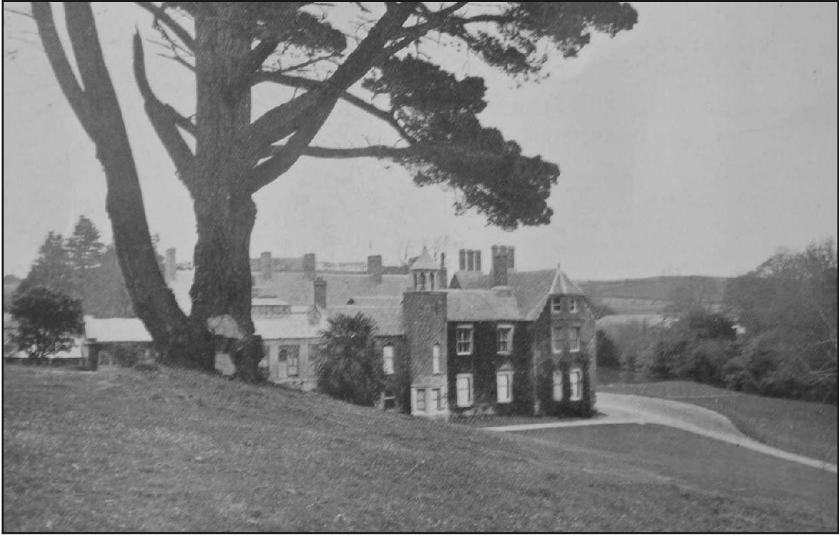
Fig. 14 Photograph of the house from the 1928 sale catalogue showing the glazed roof and lantern of the south-western range (Devon Record Office 547B/P2714).
