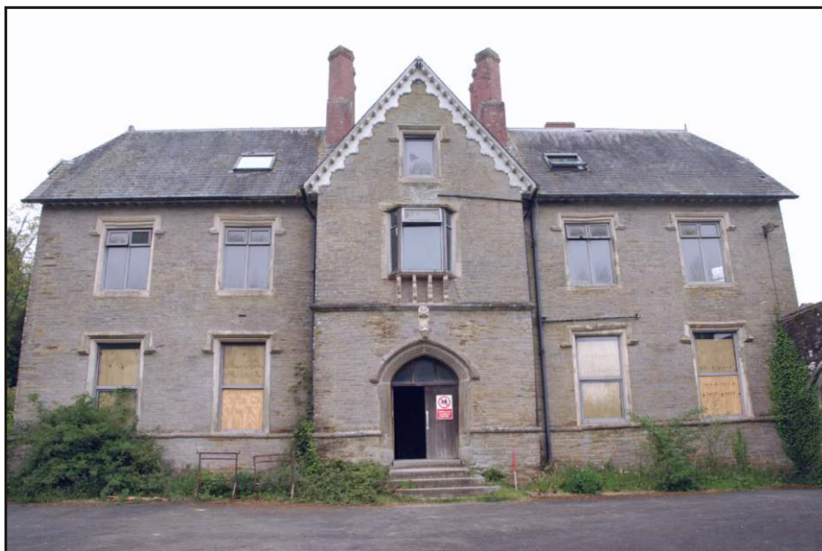
Fig. 7 View of the east elevation or entrance façade of the house showing the reused entrance archway and modern doors.
