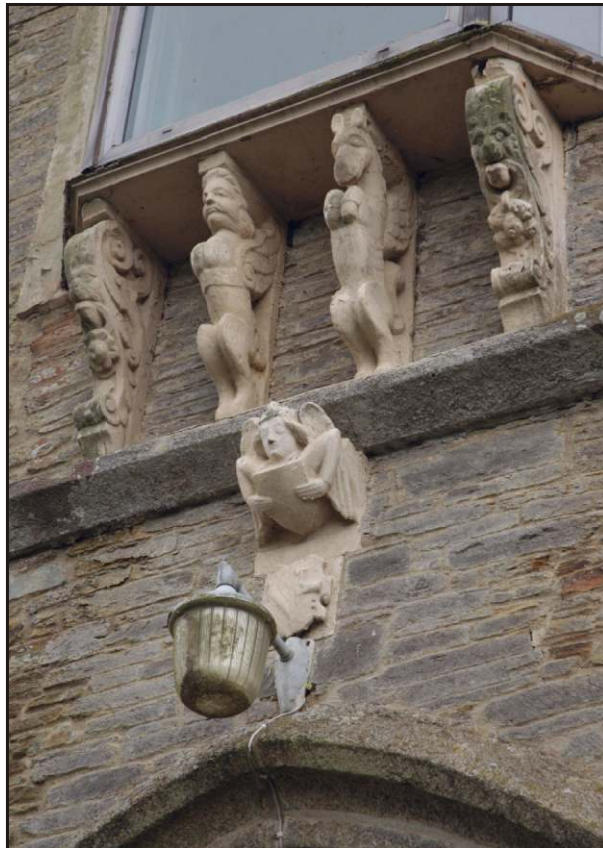
Fig. 8 Detail of the reused 16th-century and 17th-century carvings over the main doorway, and the reused corbels supporting the oriel window.
