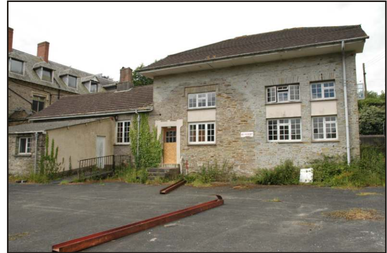
Fig. 33 The eastern range of the service buildings, showing the extent of 20th-century alteration.
