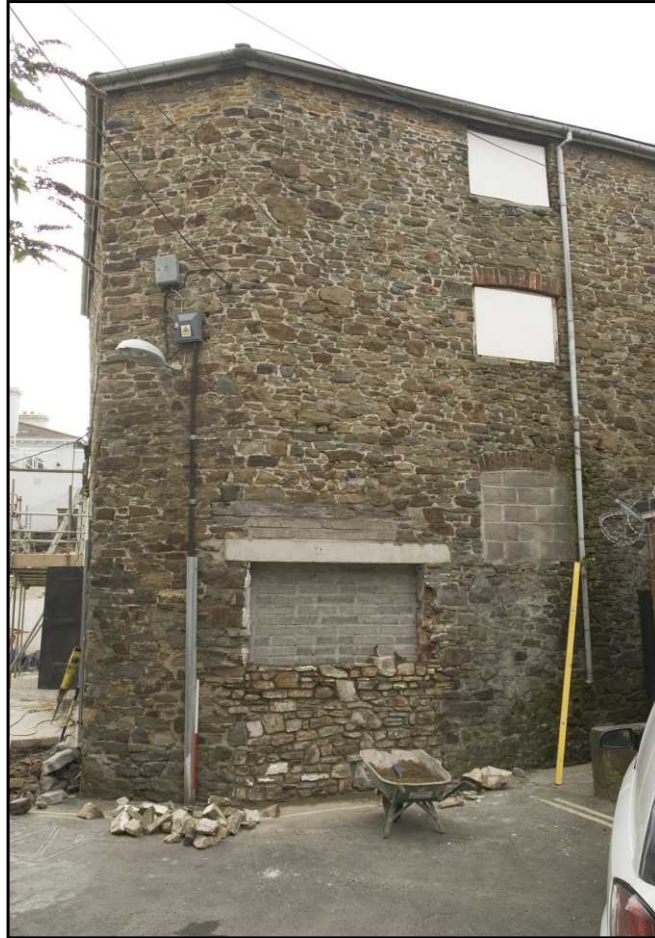
Plate 1 The warehouse viewed from King Street, looking south-west. 1m scale.
