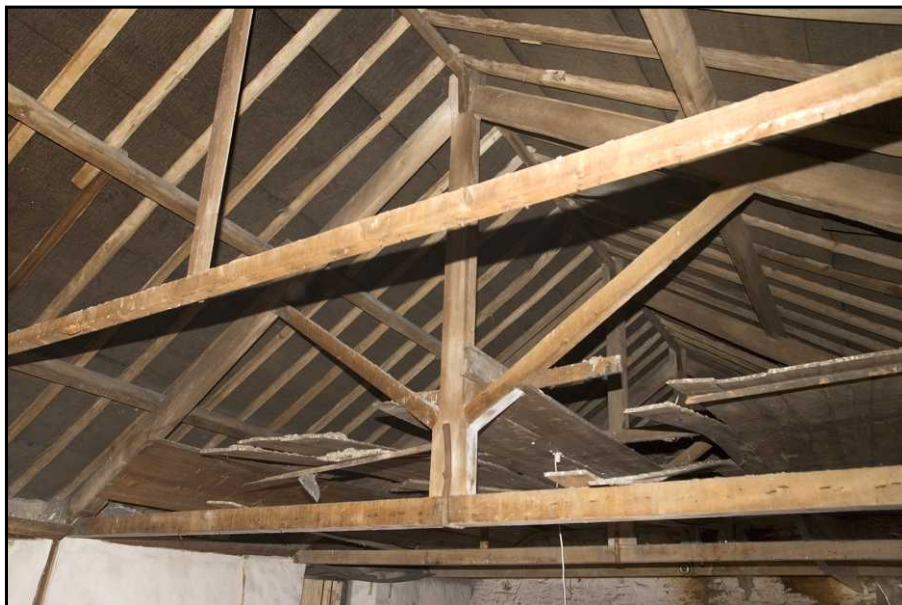
Plate 6 Roof trusses showing boards, looking south-west.
