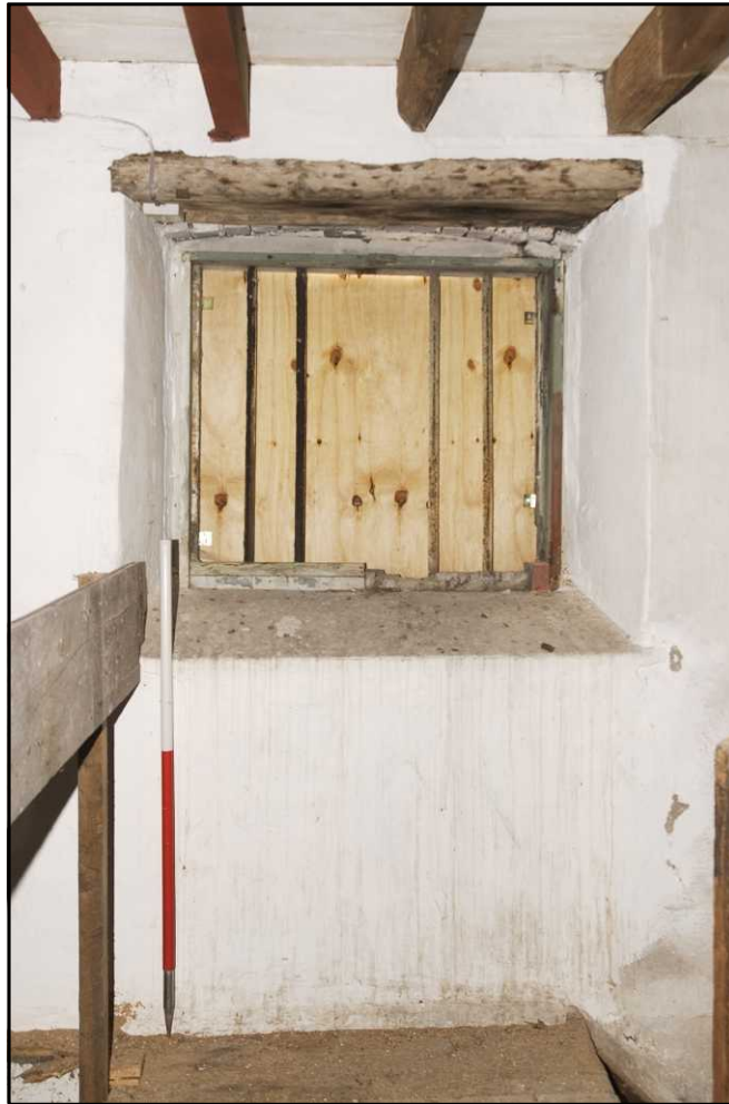
Plate 3 Close-up view of a first-floor window, looking south. 1m scale.
