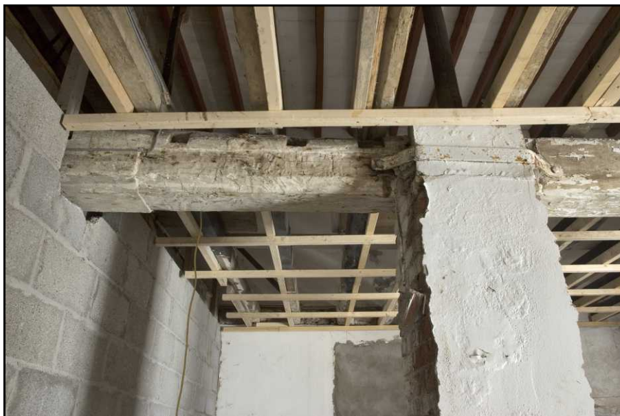
Plate 4 Reused beam supporting the first floor, looking west.
