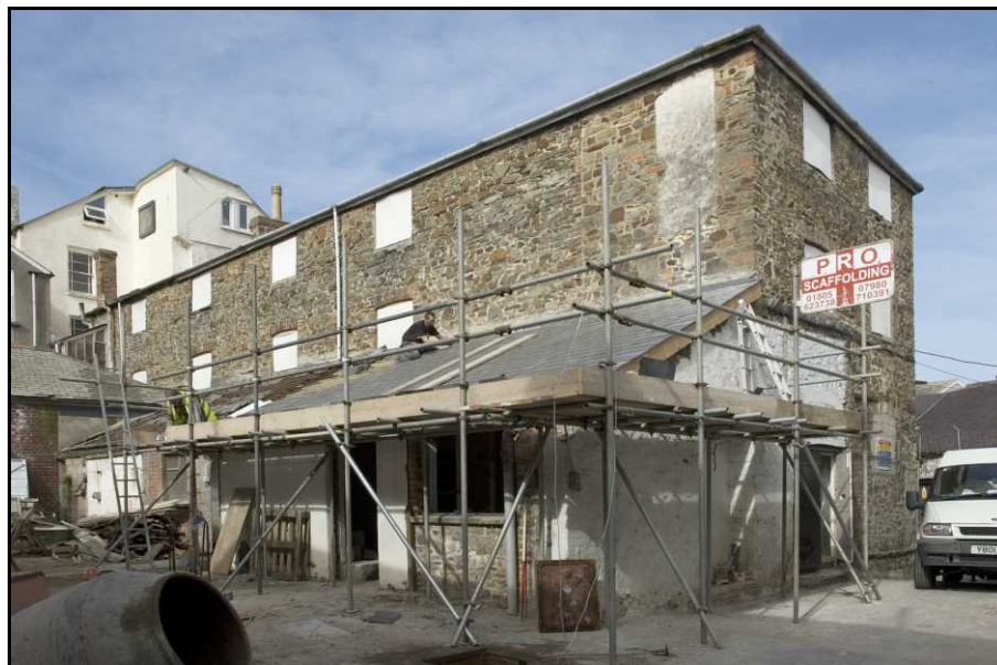
Plate 2 The warehouse viewed from its courtyard, looking north-west. 1m scale.
