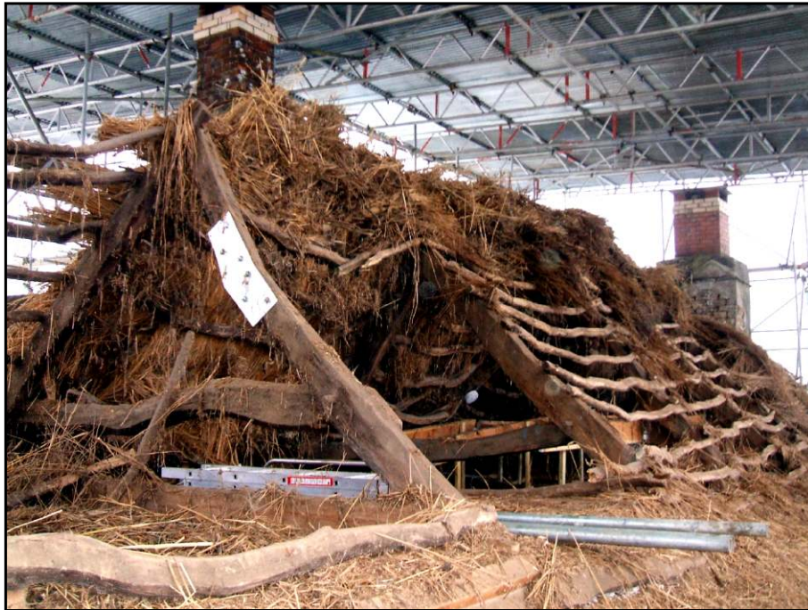
Pl. 1 The north side of the roof following removal of thatch, looking south-west.
