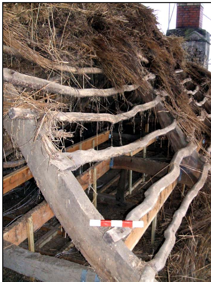
Pl. 2 The roof between trusses 2 and 3 showing thatching batons, looking south. Scale 0.25m.
