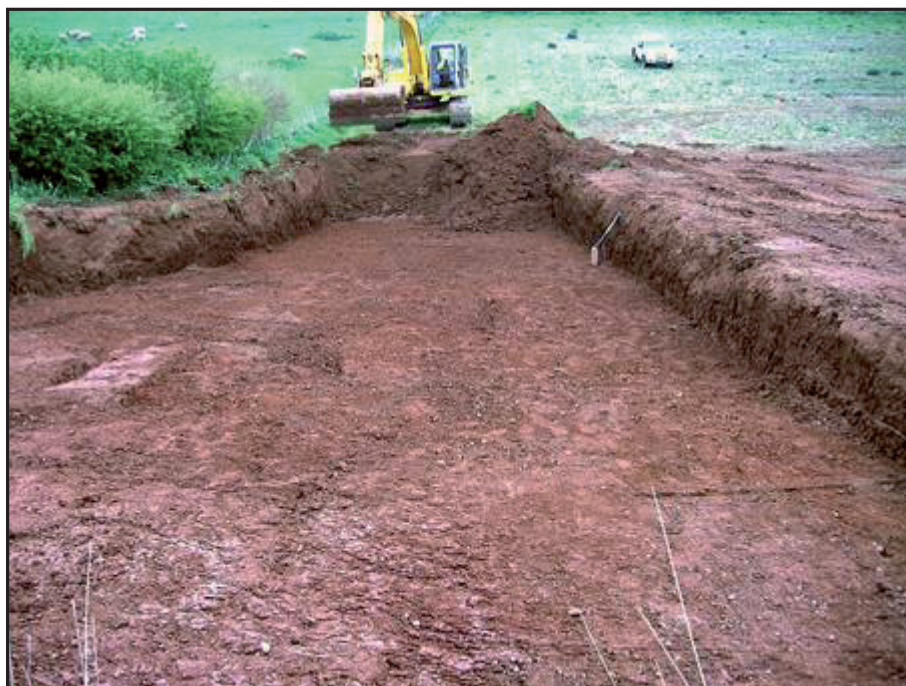
Pl. 1 Topsoil stripping, looking west.
