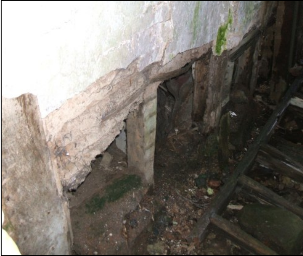
Plate 3 Screen, showing infilled doorway, looking north.
