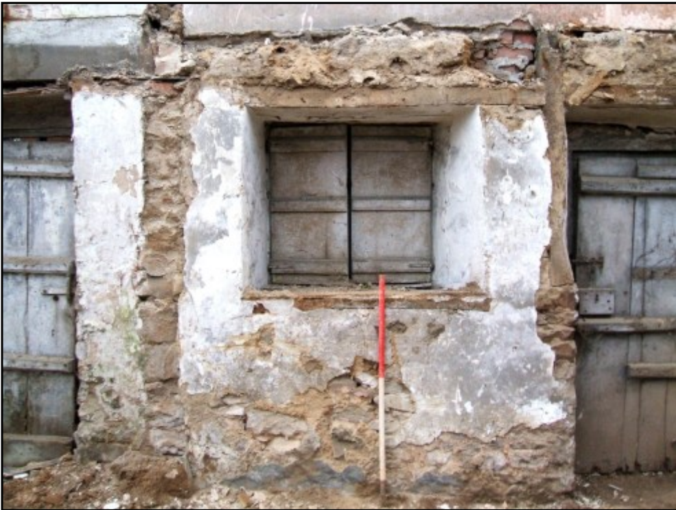
Plate 4 East internal elevation of the house showing scar of screen, window shutter, and cruck, looking south-east. 1m scale.
