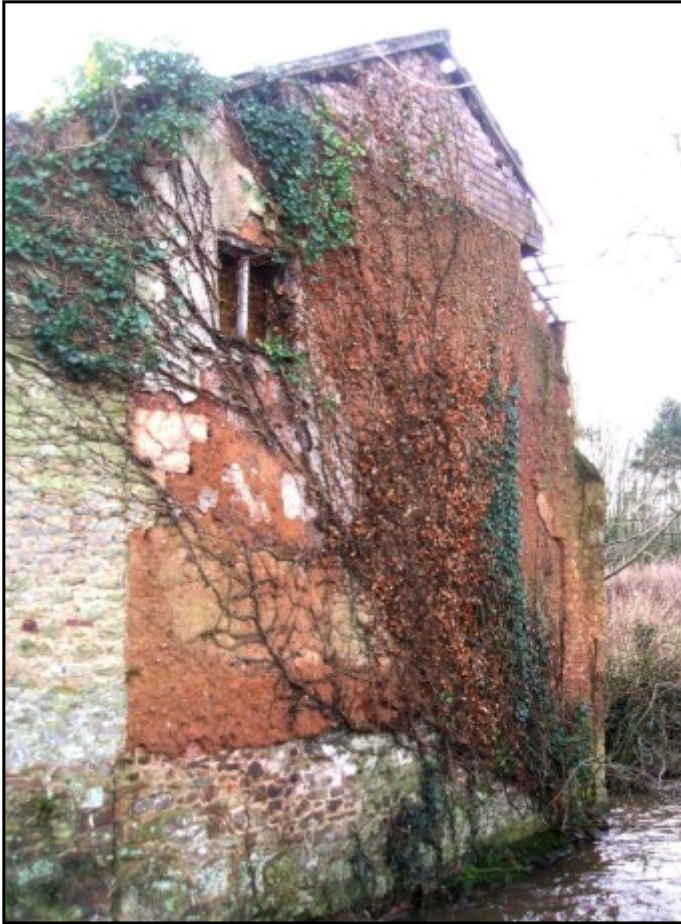
Plate 1 The north elevation of the barn, looking south-west.
