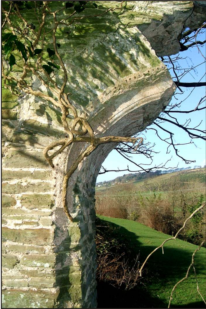
Pl. 5 Close-up of inside of four-centred arch. Looking north-west.
