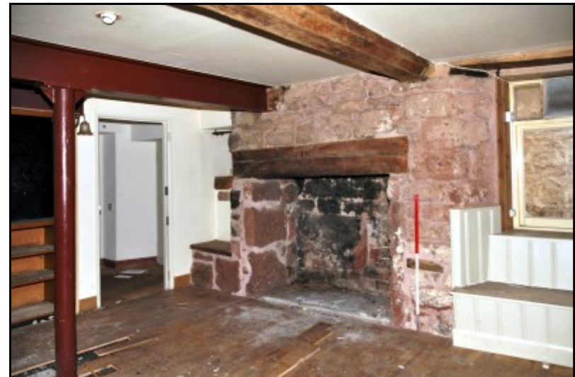
Fig. 12 View of the fireplace in the hall prior to stripping.
