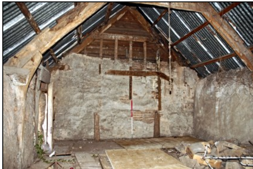
Fig. 25 View of the first-floor interior, looking to south east.
