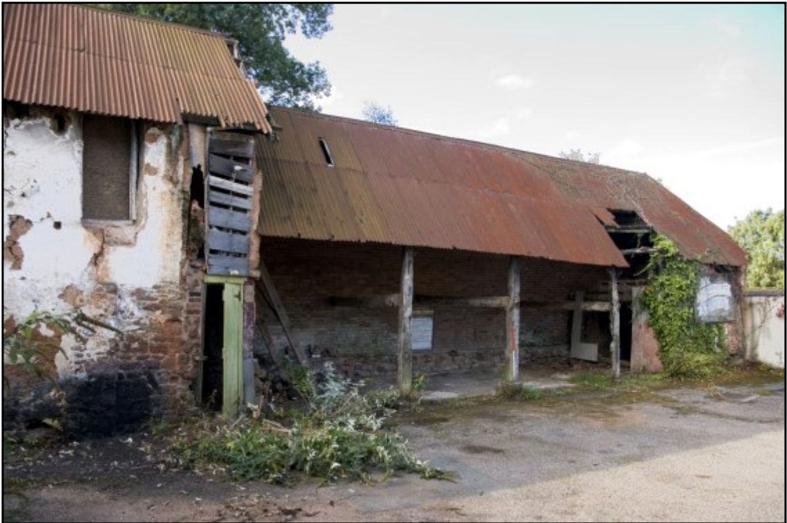
Fig. 28 View of the linhay prior to demolition, looking south west.
