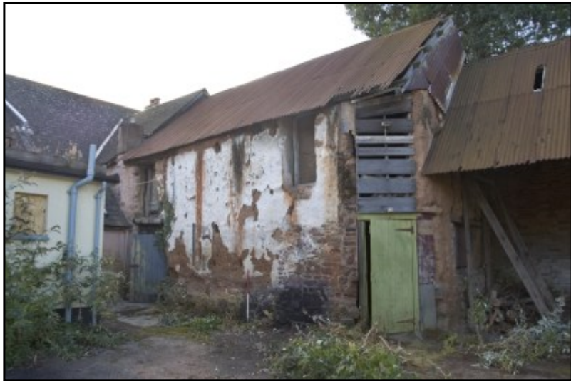
Fig. 21 The main elevation of the stable before refurbishment, showing the truncated corner.
