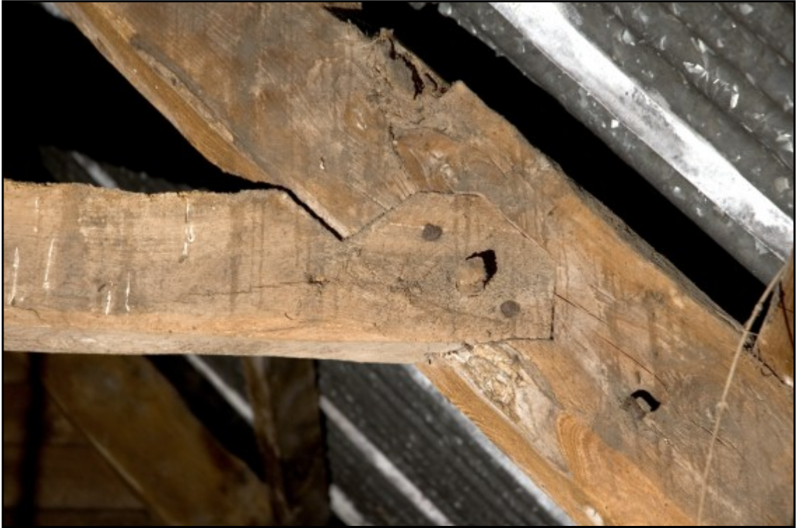
Fig. 27 Detail of a notched lap joint from the stable roof.
