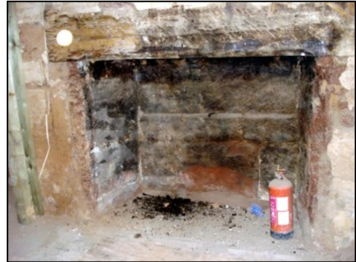
Fig. 10 View of the northern fireplace following the removal of modern fabric.
