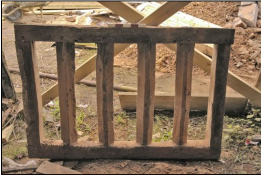
Fig. 23 Detail of the early window salvaged during demolition of the gable.
