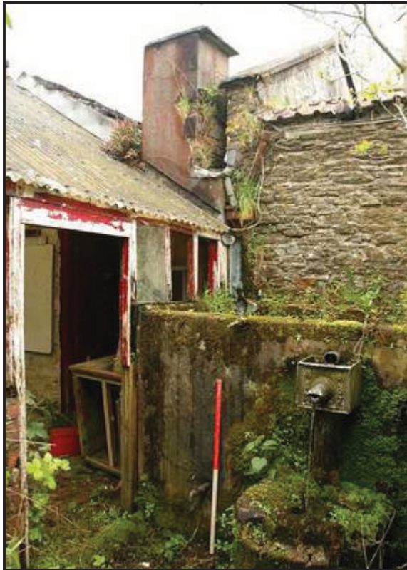
Plate 16 Well-head and tank, service buildings and masonry gable and north wall of southern greenhouse (Sites 24 to 26).
