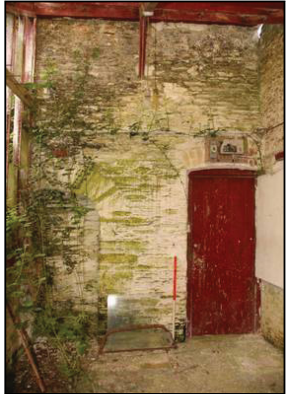
Plate 17 Interior of northern service building, showing doorway in east wall of garden, with adjacent earlier stone recess (Site 25b).
