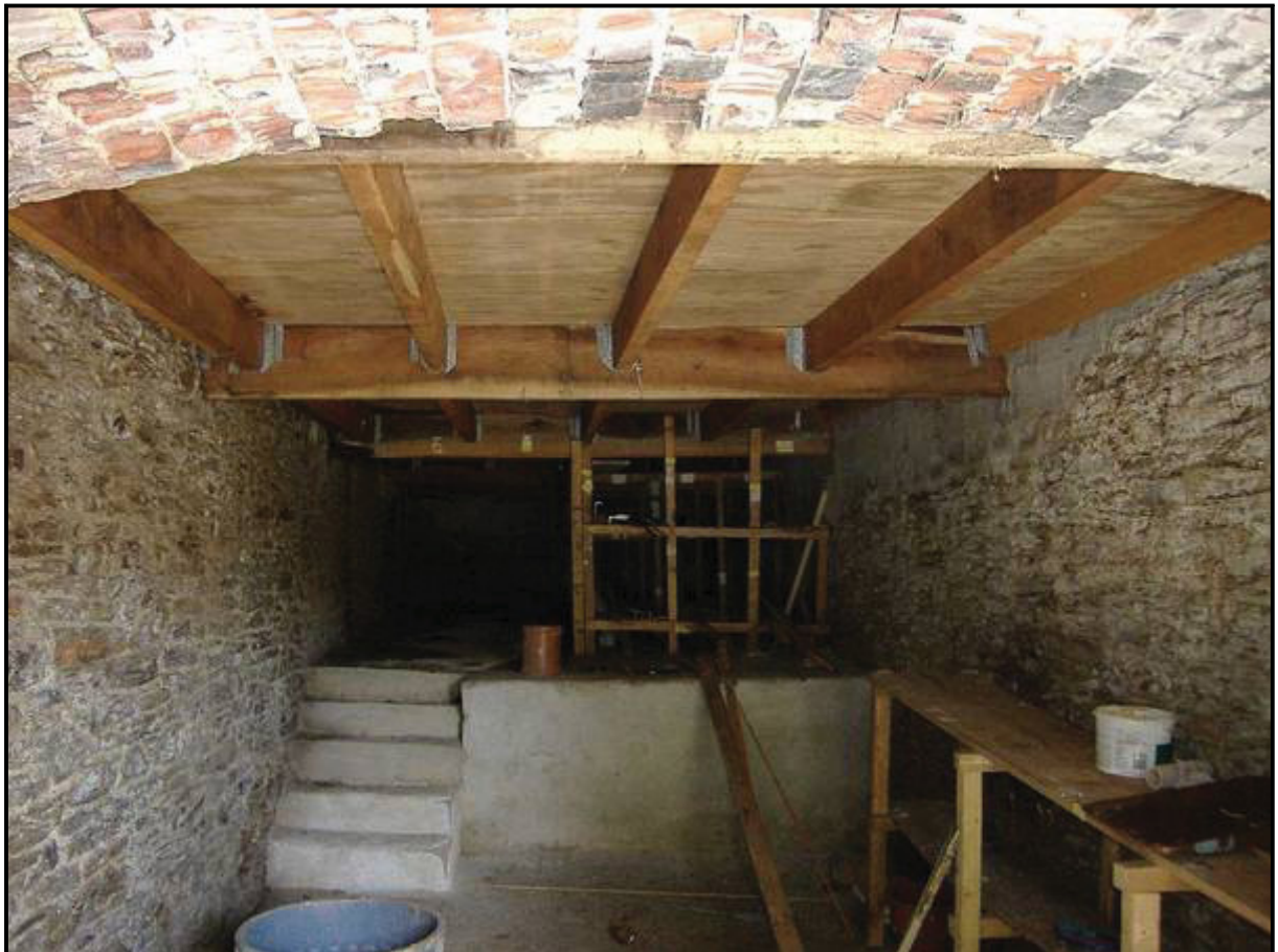
Plate 11 View looking north of the interior of the building (Site 9), showing internal slate rubble walls and concrete platform at the rear of the building.
