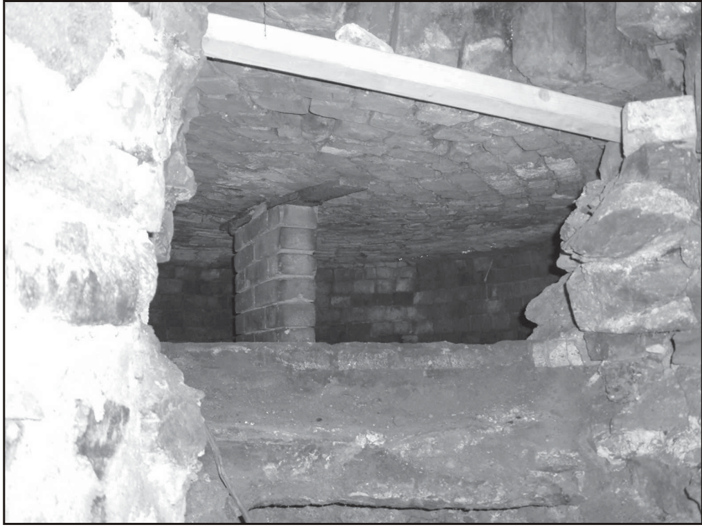
Fig. 10 Bakery oven, showing floor, central pedestal and bar supporting the vault.
