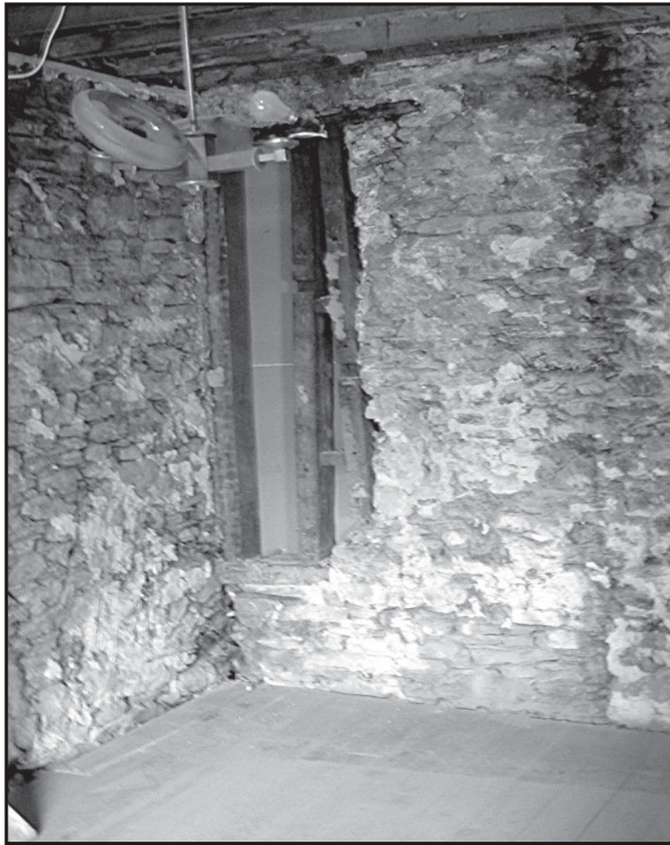
Fig. 14 Rear room, first floor, showing party wall (left) and rear of 17C stack. Note change in mortar in the centre of the right hand view.
