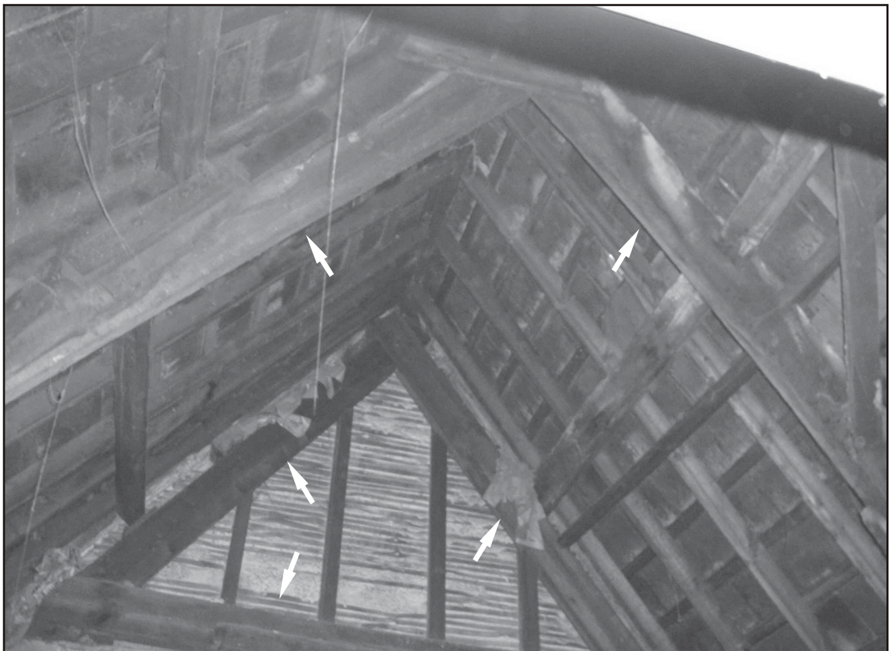
Fig. 15 17C roof over rear room looking north, showing old trusses and purlins (arrowed), with recent re-roofing and rebuilt back wall.
