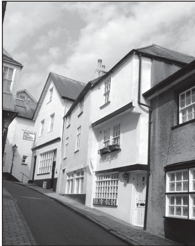
Fig. 4 The frontage on Smith Street.
