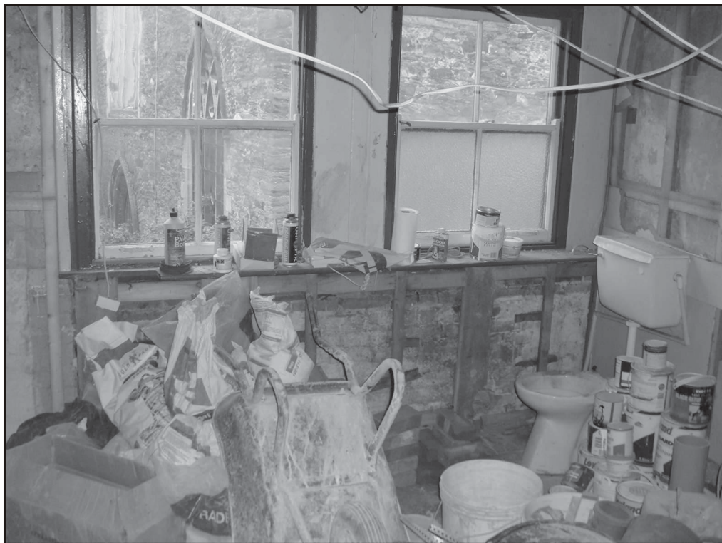
Fig. 9 The rear room, ground floor, showing modern brickwork below the window.
