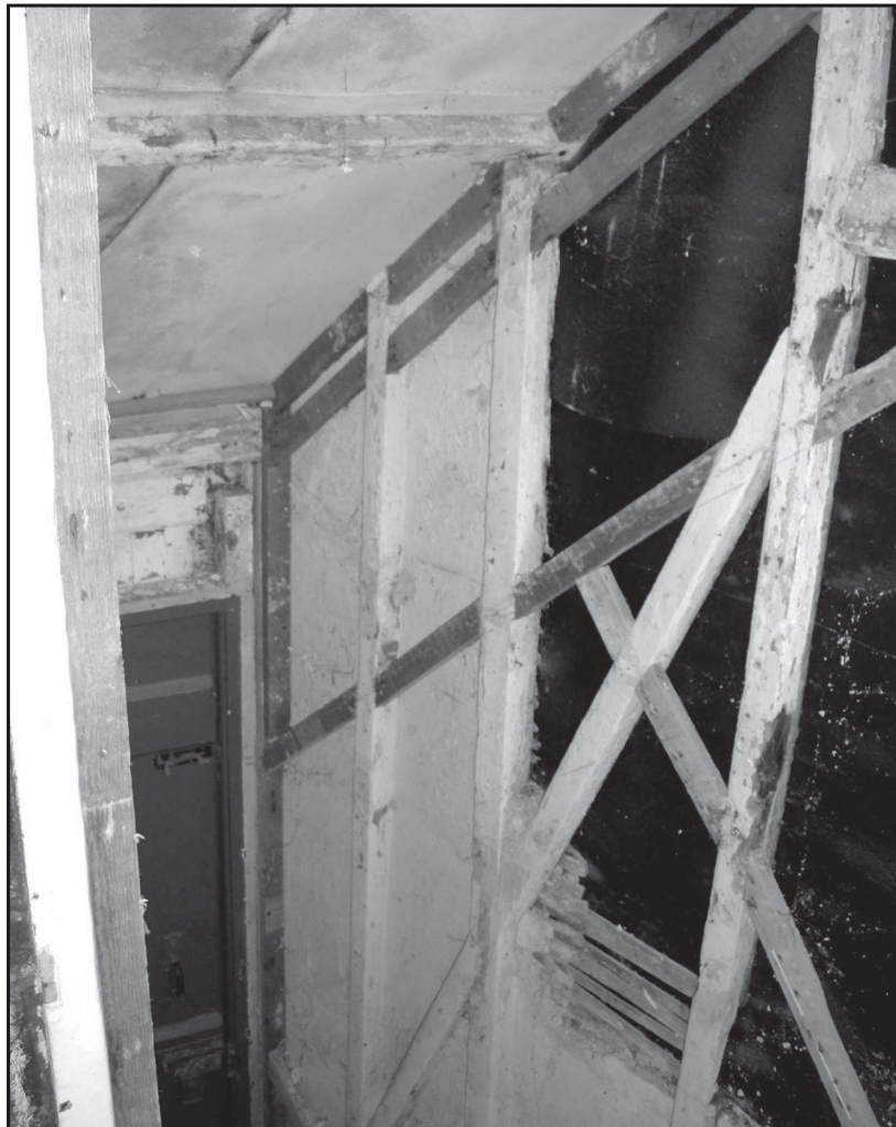
Fig. 17 The rear stairs.
