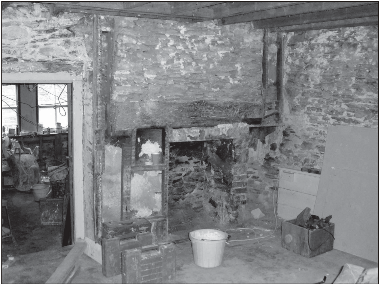
Fig. 6 The ground floor front room showing party wall (right), 17C fireplace with 19C fireplace below (centre) and 17C/18C doorway (left).
