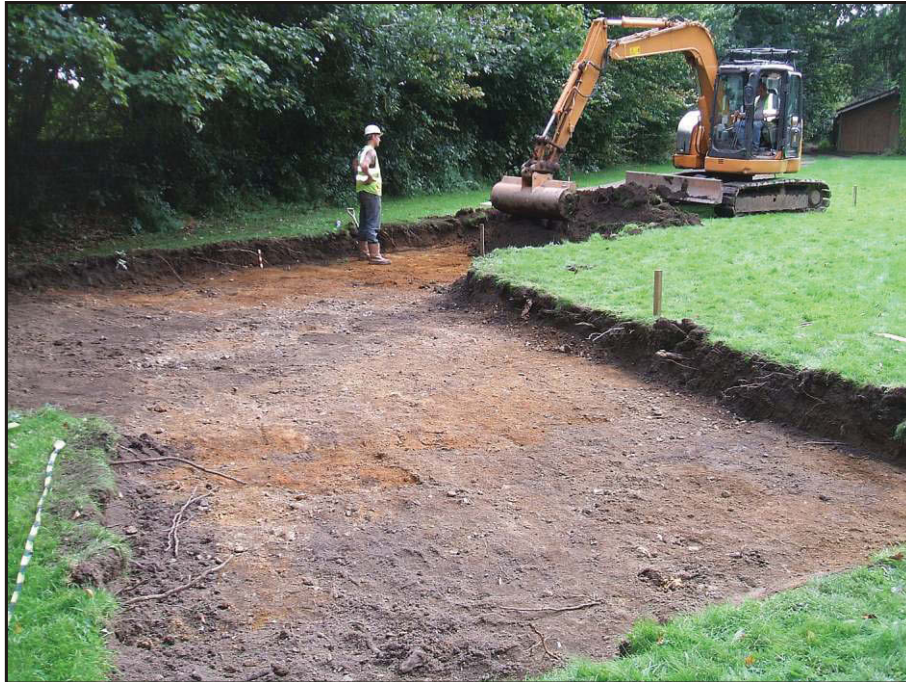
Pl. 1 General view of topsoil removal, looking north-east.
