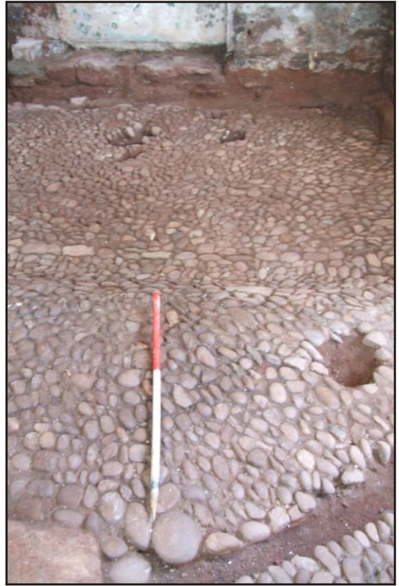
Plate 10 General view of pre-1678 quay surface (5022/3) and postholes (5008-5012). Looking north (scale 1m).
