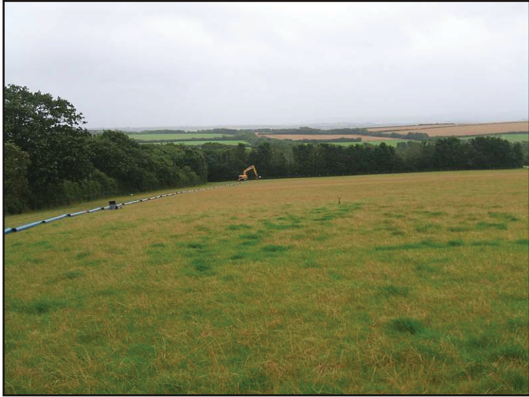
Pl. 1 General view of pipeline. Looking south.
