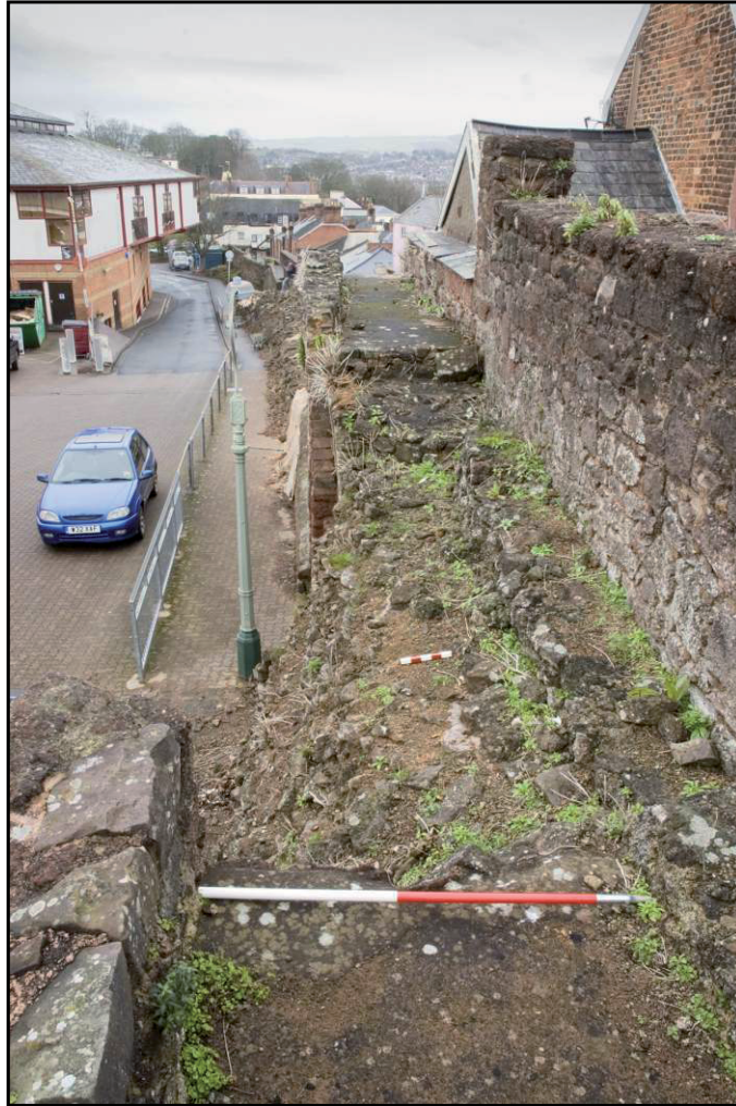
Plate 1. General view of site prior to work commencing, looking SW.
