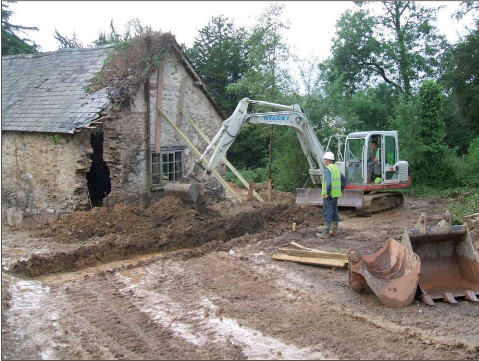
Plate 1 General site view, looking south-east
