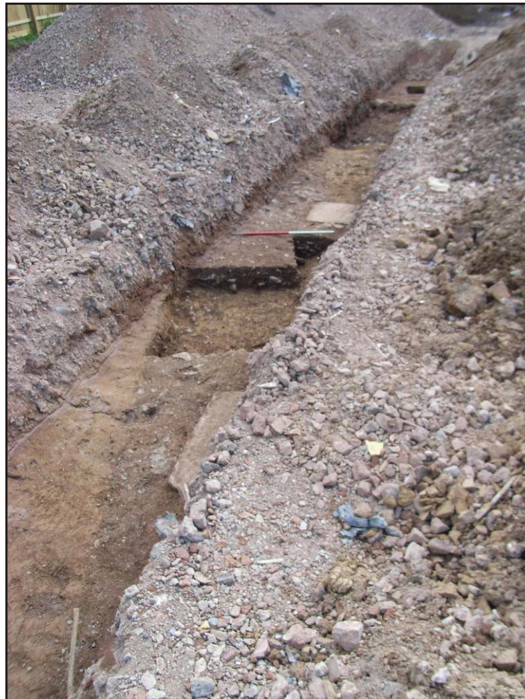
Plate 2 View of trench 1 showing robbed out wall footings 204 and 210. Looking north-east.
