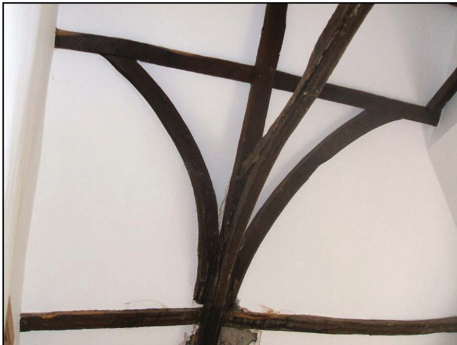
Pl. 4 The medieval roof of the cross wing, showing the south truss and wind braces on the east side of the roof, looking south-east.
