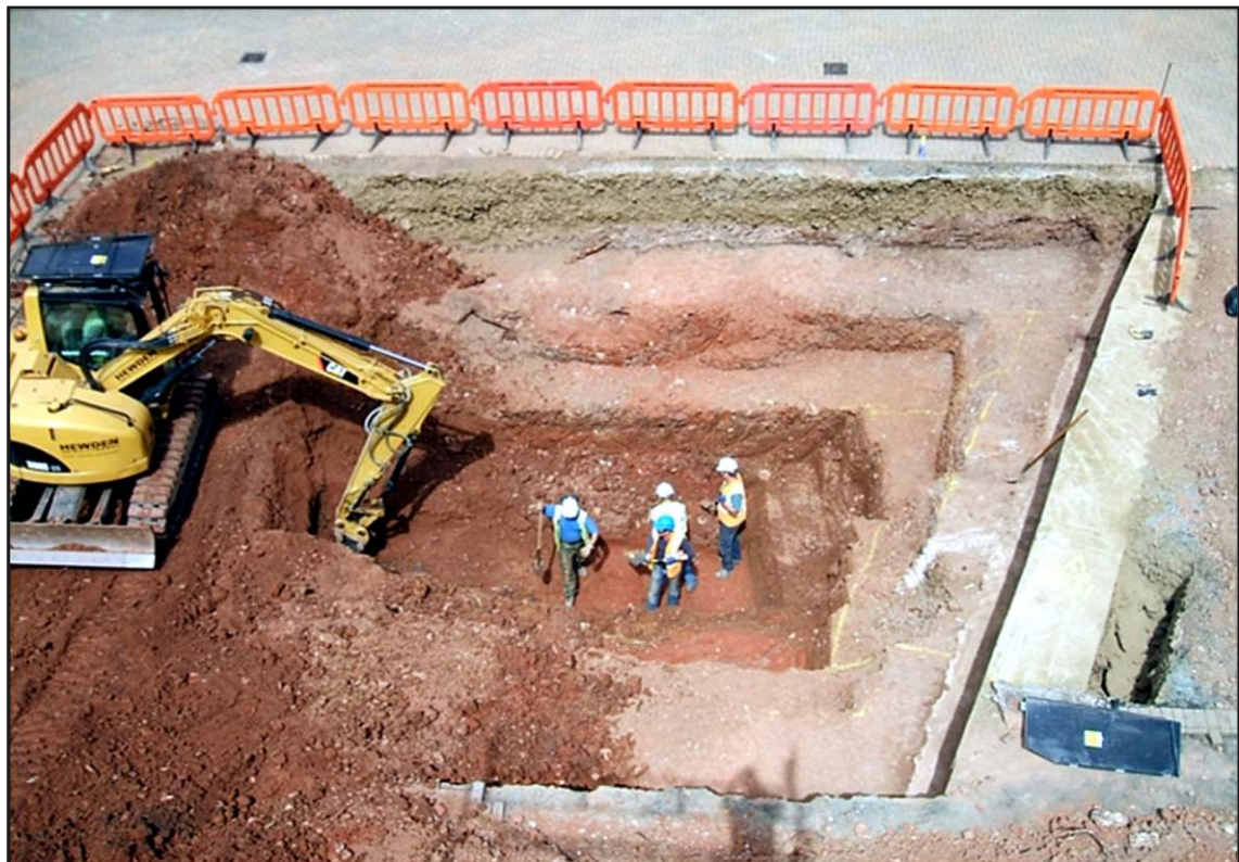
Plate 2 Stepped excavation underway within the eastern half of the site. View to north.
