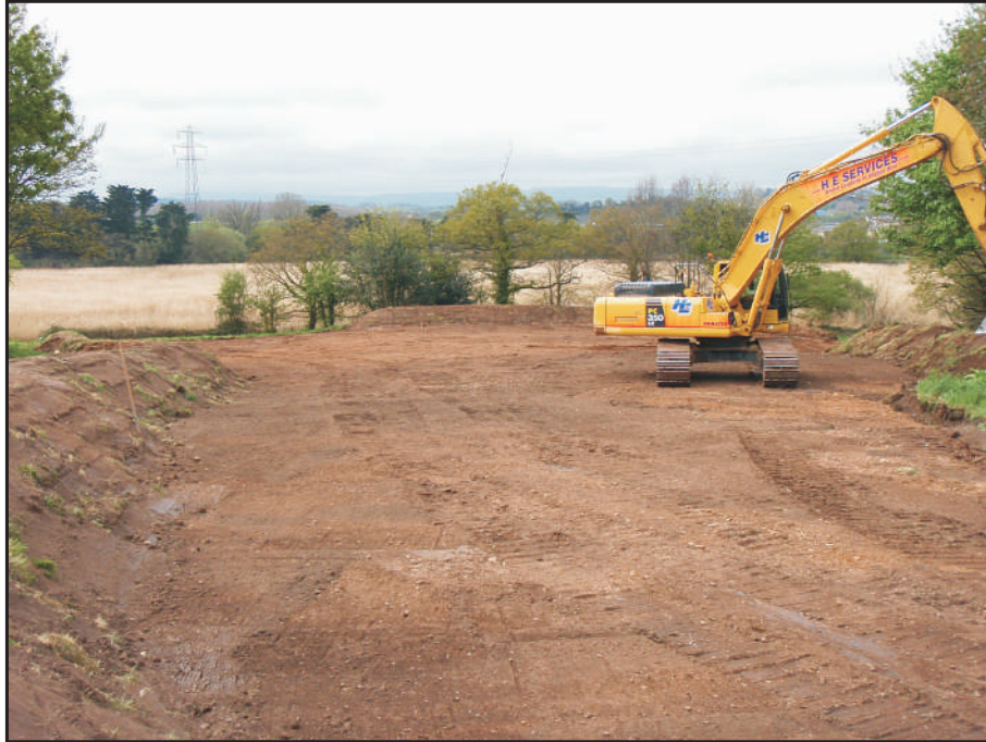
Pl. 1 General view of site. Looking southwest.
