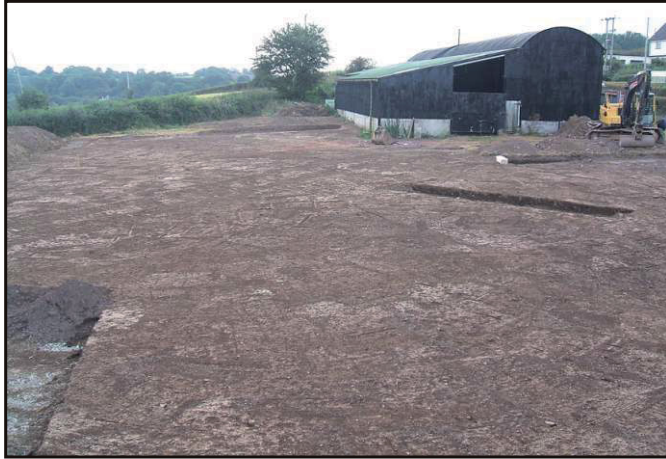
Plate 1 General view of site, looking east.
