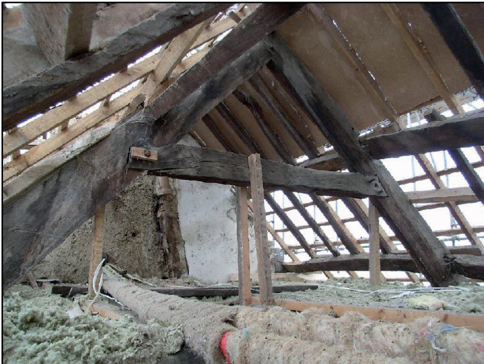
Pl. 2 The truss in the east range, looking north-east.
