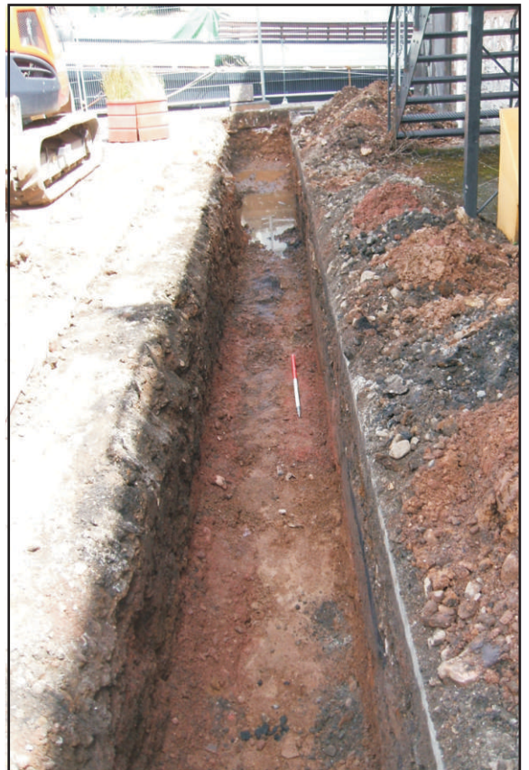
Plate 12 General view of Trench 5. Looking northeast. 1m scale.
